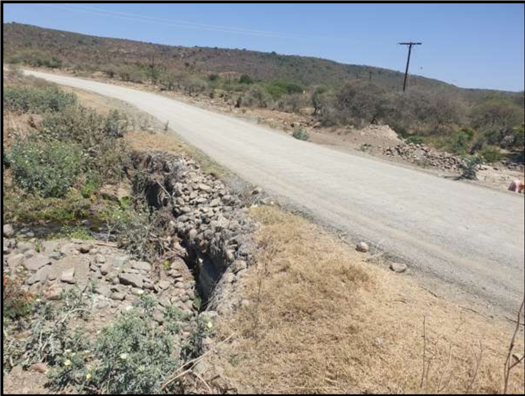
FIG. 9: EXISTING CAUSEWAY AT UMSOBOTSHE RIVER
