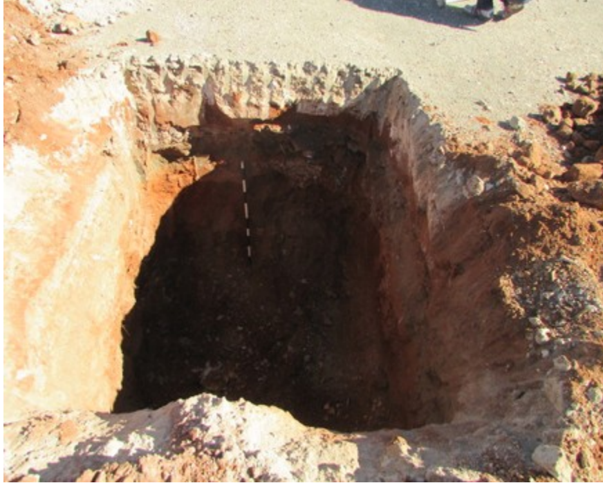
Figure 17: TP2 - Building rubble visible on eastern side of pit.
