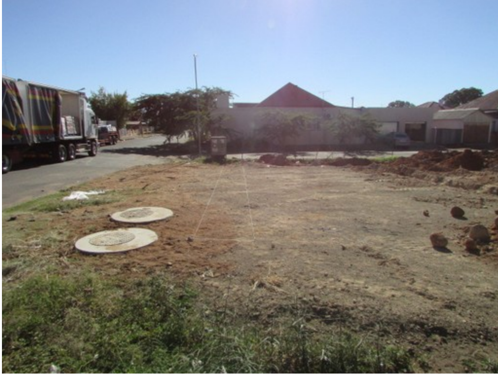
Figure 7: Test Trench 1 prior to excavation. The man-holes show the approximate Neotel Line connection.
