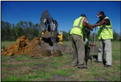
Excavations at T33.2
