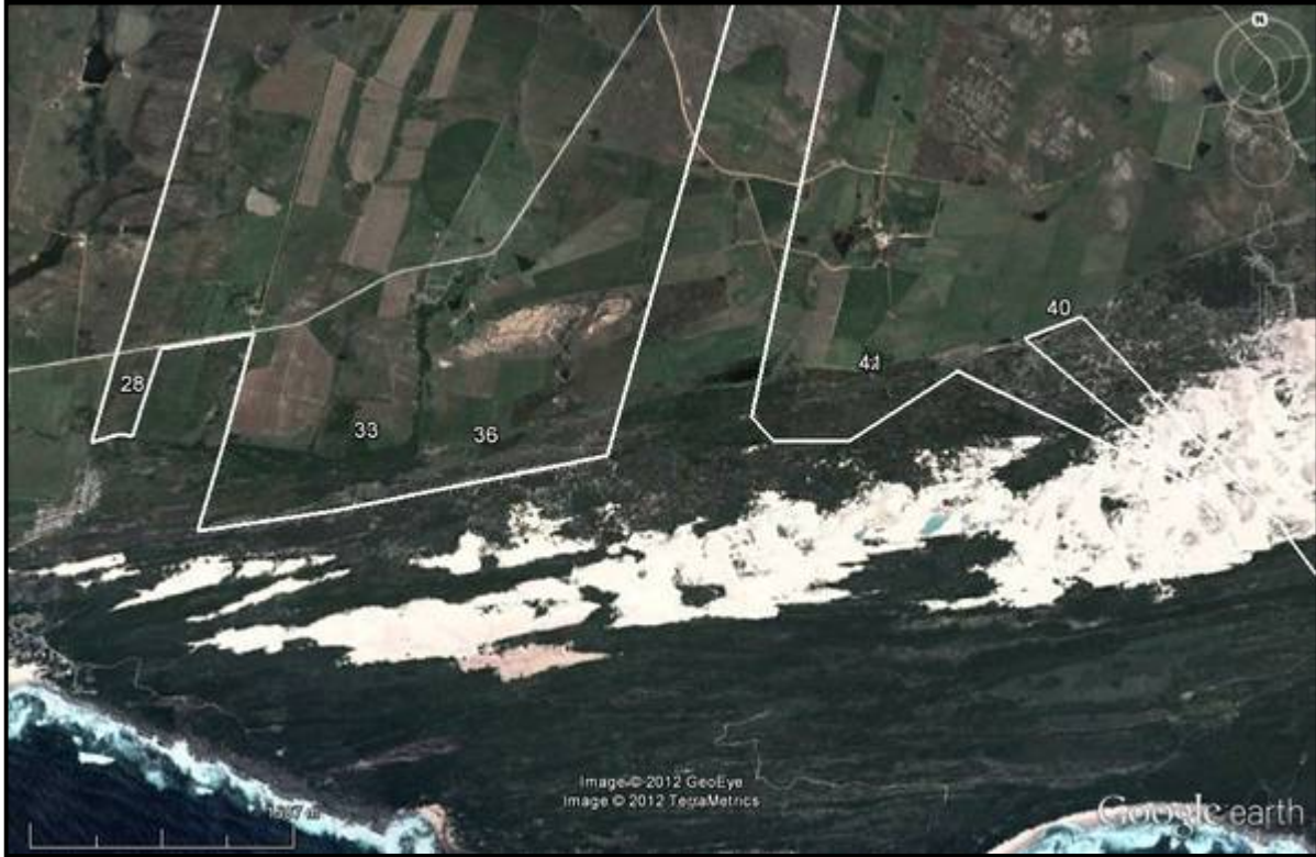
Figure 15: Turbine Line 33-36 in relation to turbines 28, 41 and 40
