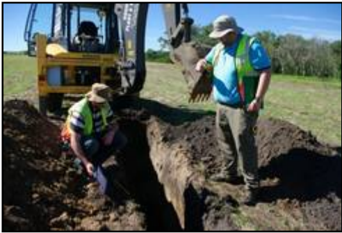
Excavations at T33.1
