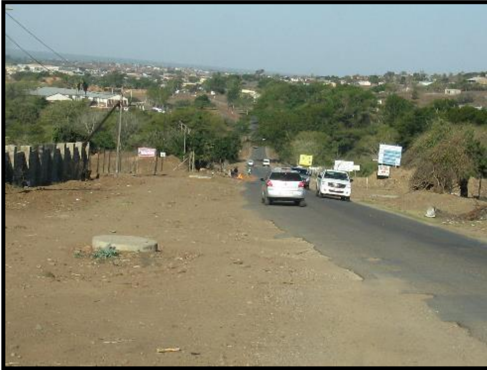
Figure 3. Northern section of the P449.
