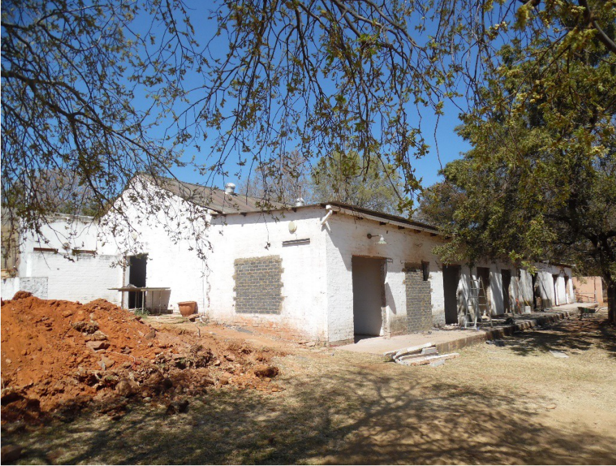
Photograph 1: Structure situated on area earmarked for development (structure does not appear to be 60 years or older)
