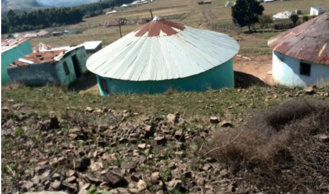
Figure 6: Houses located close to eastern boundary of borrow pit
