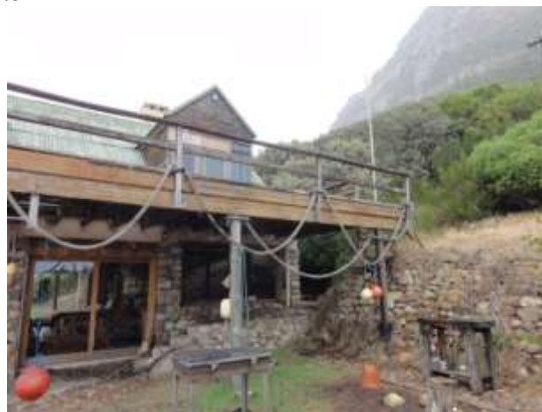
Fig 11. Existing house at Partridge Point situated on a flat portion of the site, with the slope to the west and the R45 in the background. The building has no heritage significance
