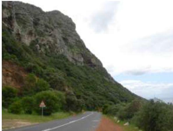
Fig 3. View from M4 looking north and showing the steepness of the terrain above the road.
