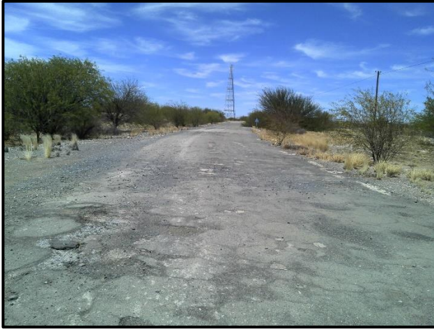
Figure 10. Existing site conditions
