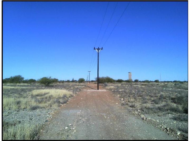
Figure 7. General site conditions
