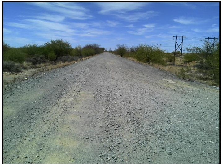
Figure 9. General site conditions
