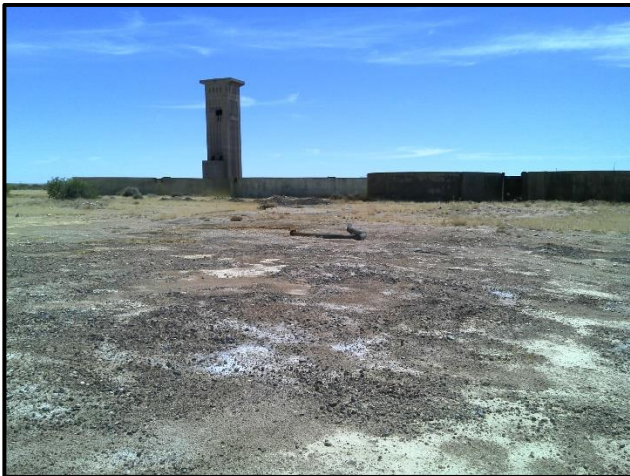
Figure 12. General site conditions
