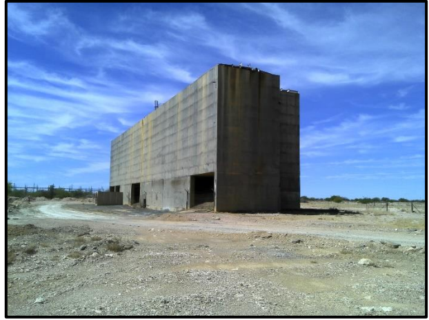
Figure 11. Abandoned mining infrastructure. .
