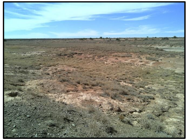
Figure 19. General Site conditions TSF1
