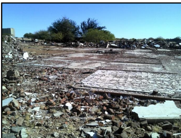
Figure 39. Remains of dilapidated structures
