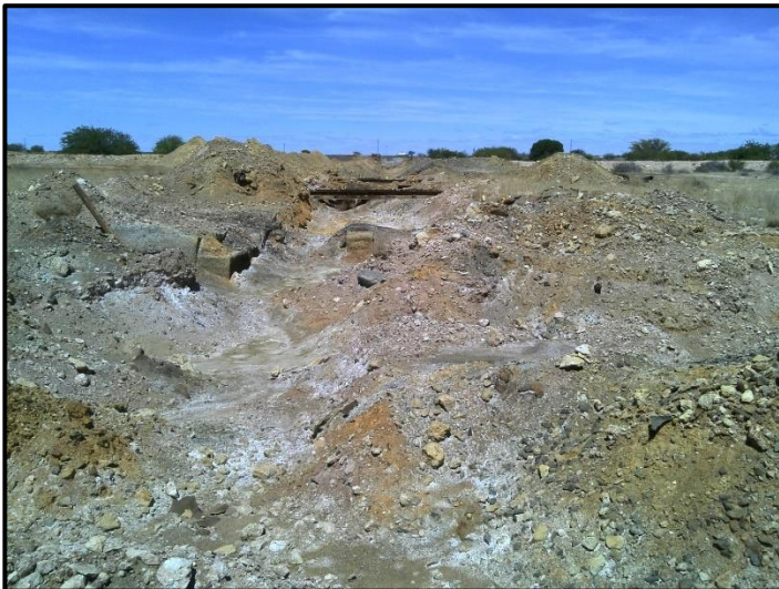
Figure 8. General site conditions
