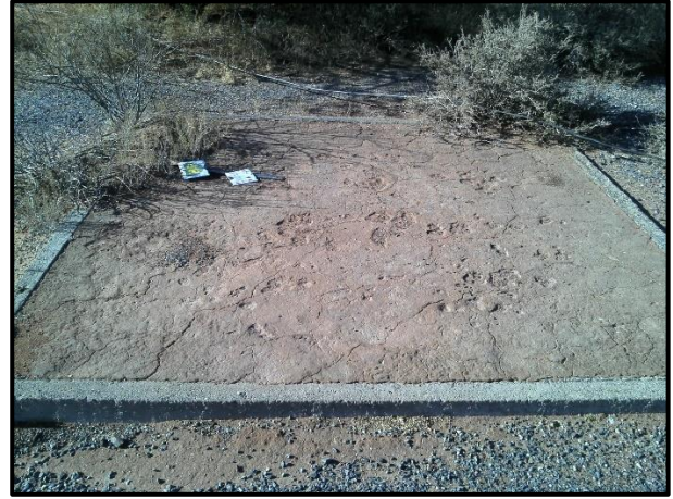
Figure 42. Cement slab in TSF 3
