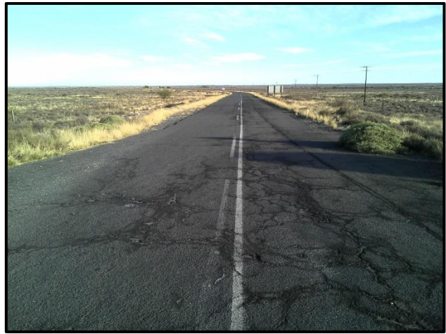
Figure 13. Existing access road
