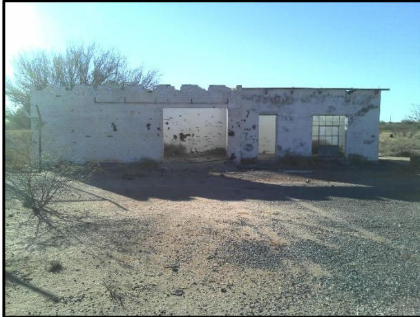
Figure 41. Structure in TSF 3
