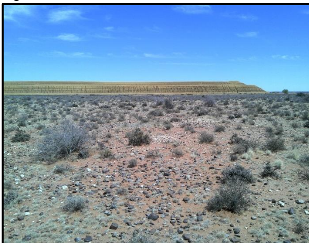
Figure 20. General site conditions TSF 2
