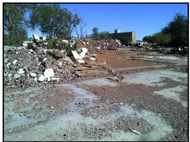
Figure 40. Remains of dilapidated structures.
