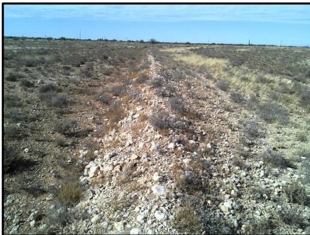
Figure 26 General Site conditions WRD 1
