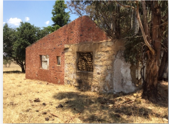
Figure 12 – The addition of the red clay brick walls are visible
