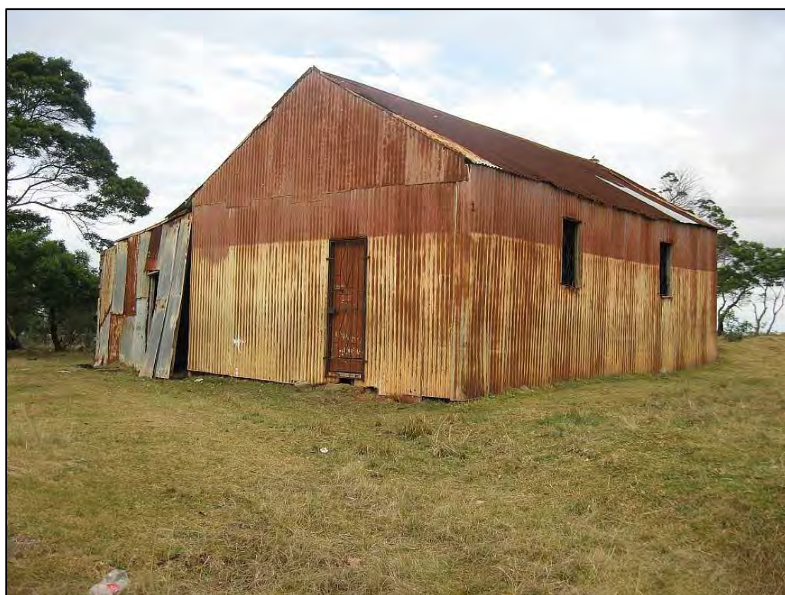
Figure 10 – Corrugated iron structure utilised as church
