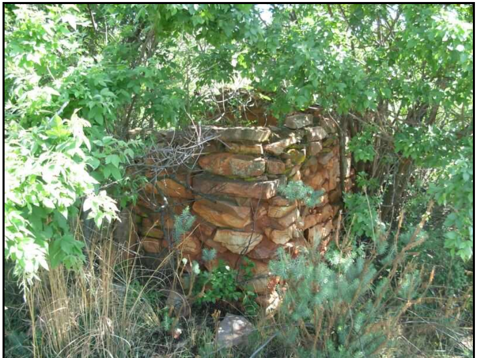
Figure 21 - Close up detail of structure
