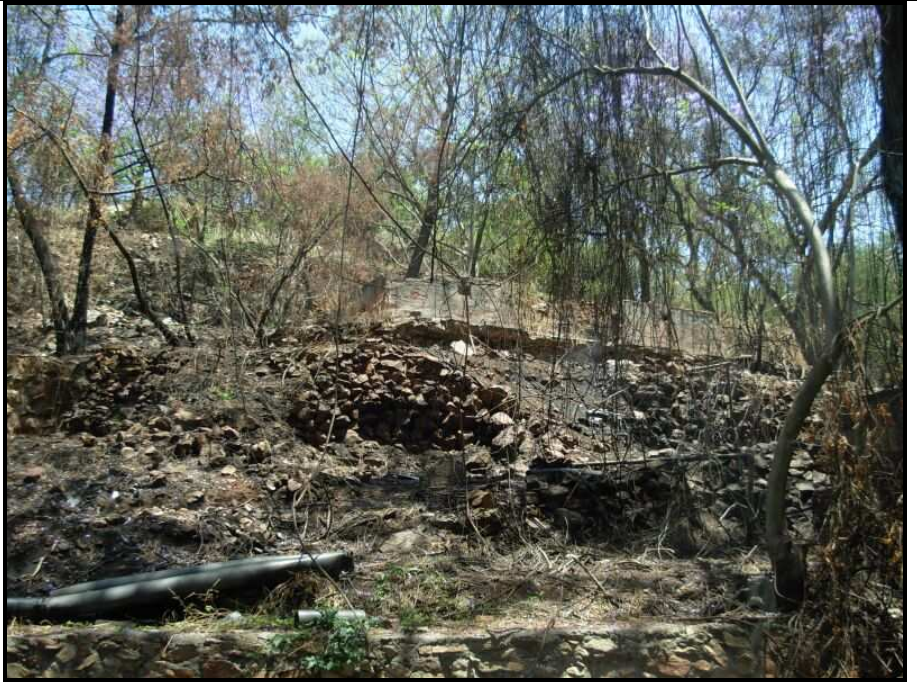
Figure 17 - Terracing close to addit on Koedoe street
