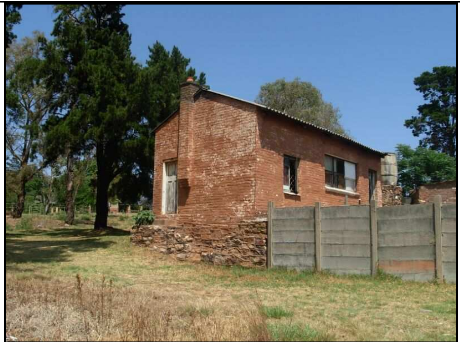
Figure 24 – Single structure as part of workers housing
