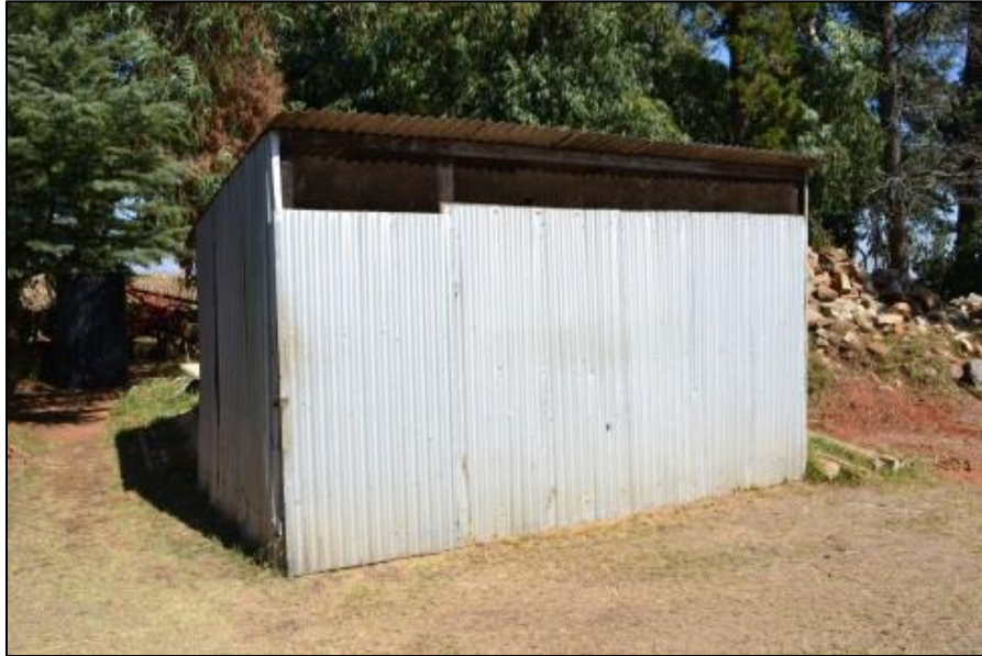
Figure 12. Timber frame corrugated iron ablution
