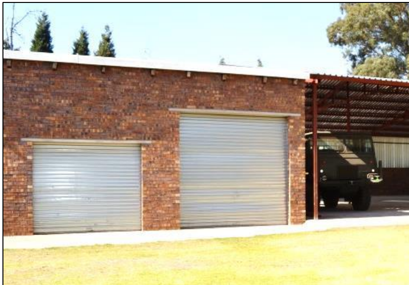
Figure 9. Face brick garages serving as annex to the large open sided shelter
