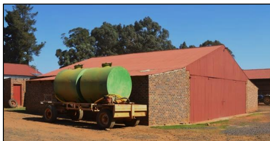
Figure 22. Old face brick shed, also known as the plane hangar, with large doors in the gable end
