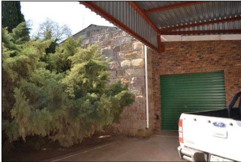
Figure 16. Back of sandstone garage (left, obscured behind the conifer) now used as storage facility
