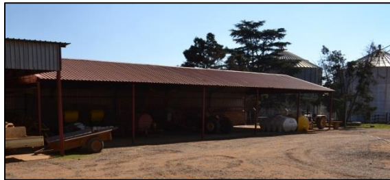
Figure 24. Large steel frame open sided storage shelter
