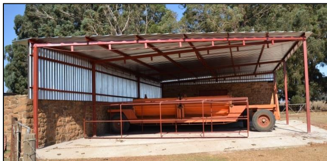
Figure 28 New open sided steel frame parking shelter
