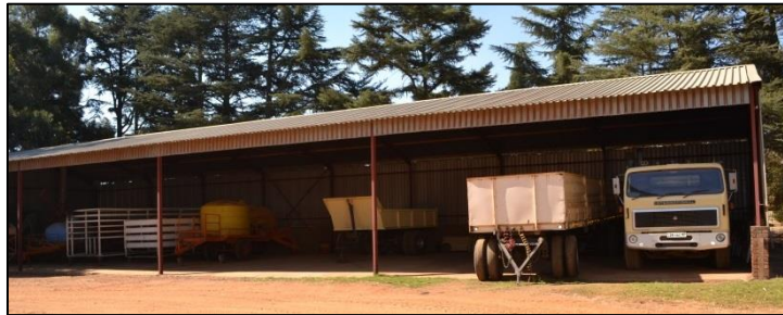
Figure 30. Large steel frame semi-open parking facility
