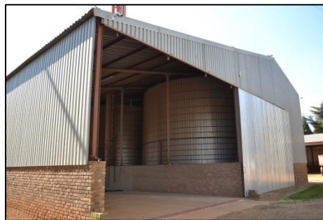
Figure 31. Large steel frame covered storage facility accommodating silos and loading bay
