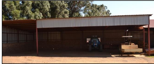
Figure 23. Open-sided steel frame parking shelter
