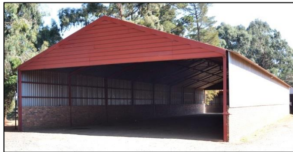
Figure 21. Large steel frame shed with open gable ends
