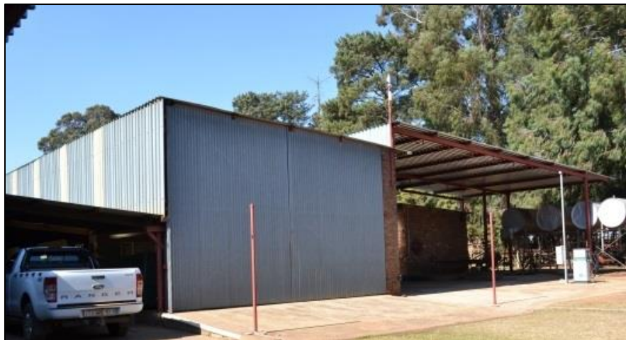
Figure 15. Steel frame galvanized sheet iron shed
