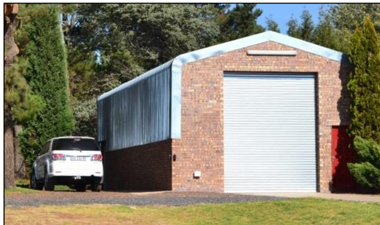
Figure 4. Northern elevation of small helicopter hangar on the north-eastern corner of the farmstead
