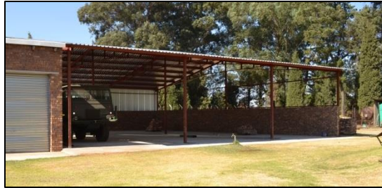
Figure 10. Open-sided steel frame shelter used as parking for utility vehicles
