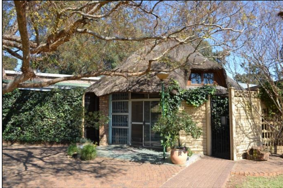
Figure 14. Entrance to office complex
