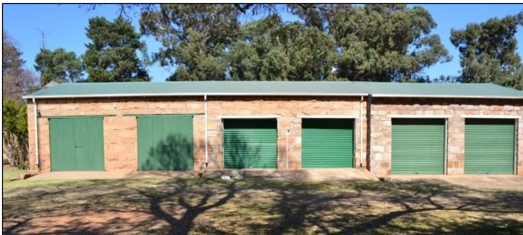
Figure 17. Series of sandstone buildings erected at different periods, now used as garages
