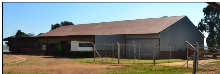
Figure 32. large steel frame storage sheds and open-sided parking shelter
