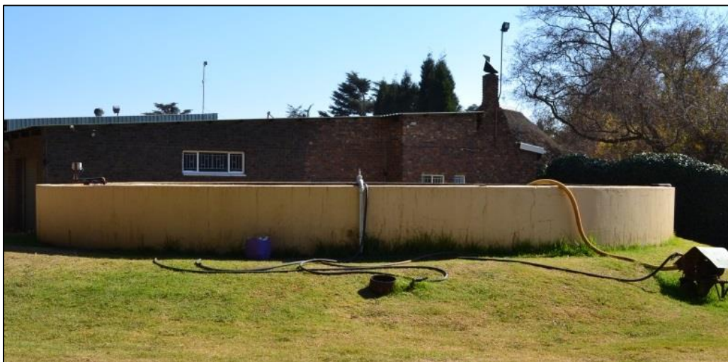
Figure 13. Circular plastered brick dam at the back of the office complex
