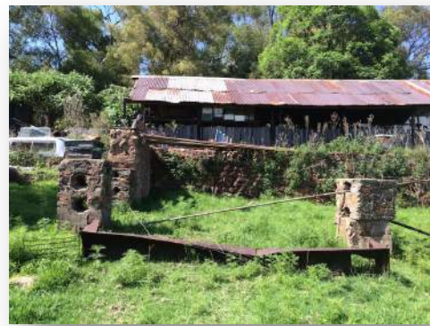
Figure 30 – Retaining wall though to have been part of British field hospital
