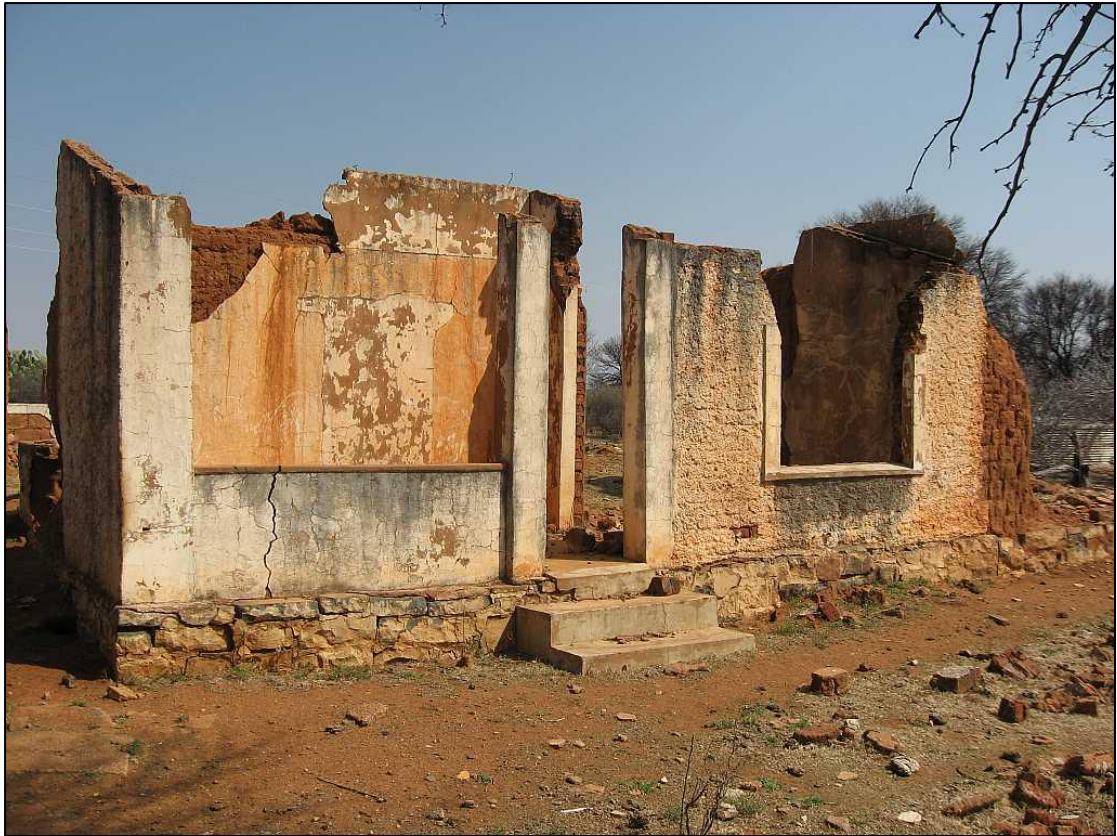
Figure 17: Main house at ACO02
