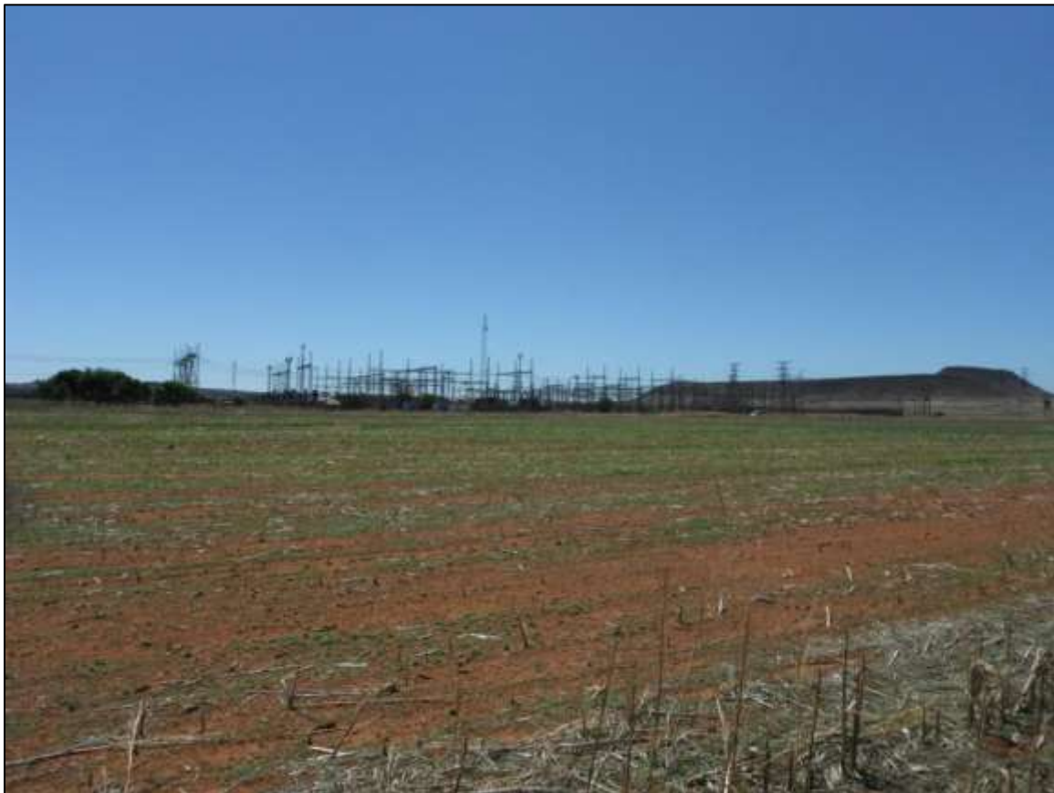
Figure 4 – General view of the proposed alternative A with Harvard Substation in the background
