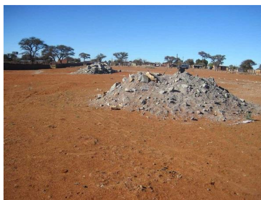
Figure 12 – Large scale dumping of building rubble on site
