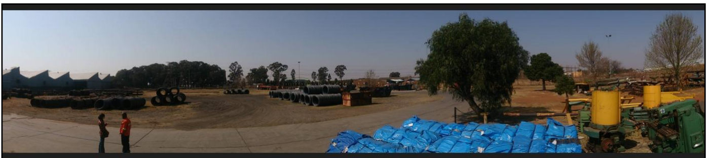
Figure 4 – Panorama view of the site from the south-west corner
