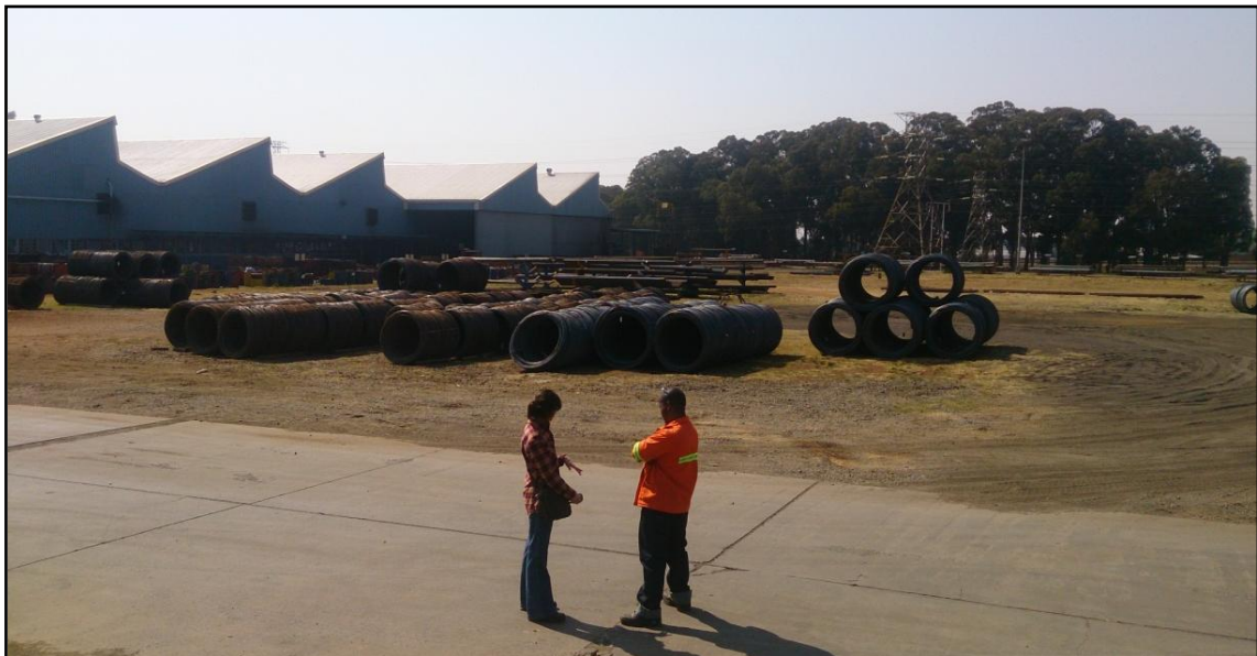
Figure 7 – View showing existing factory building
