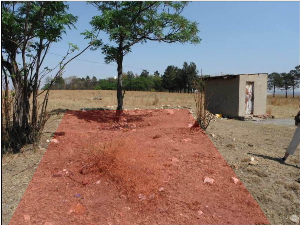
Figure 23 – View of the foundation (shaded in red) at LAN5
