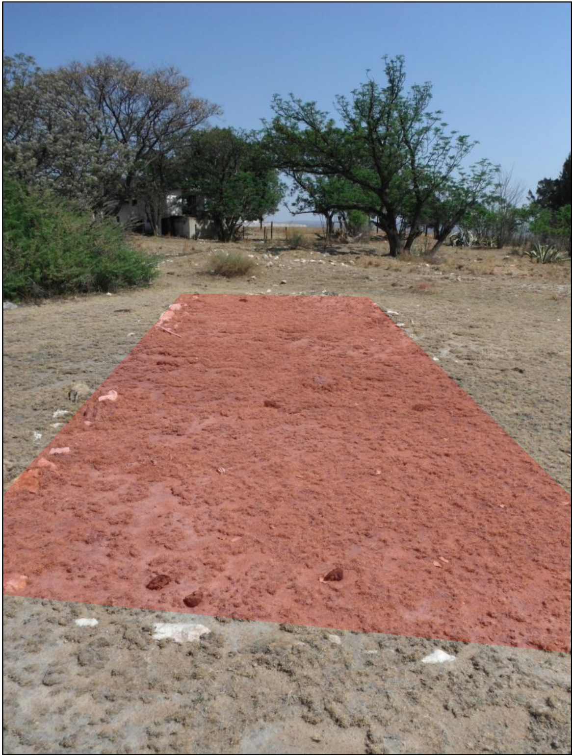
Figure 22 – View of southern section of foundation (shaded in red) at LAN4
