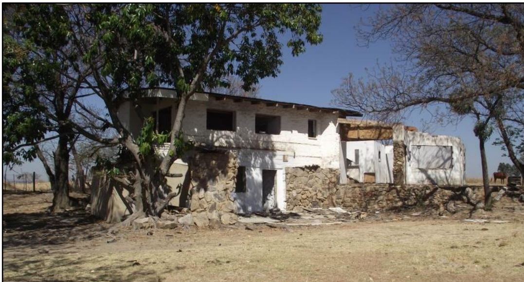
Figure 15 – View of vandalised recent/modern building
