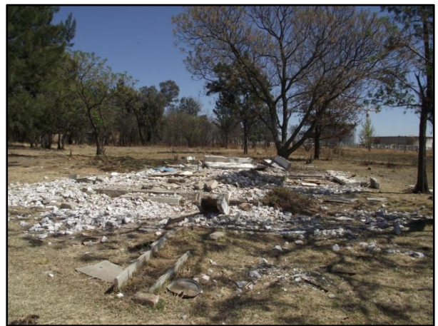
Figure 8 – View of demolished structure
