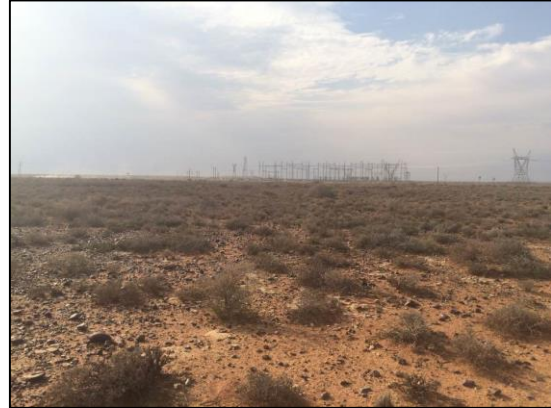
Figure 13 – View of northern corridor alignment with the Kronos substation in background
