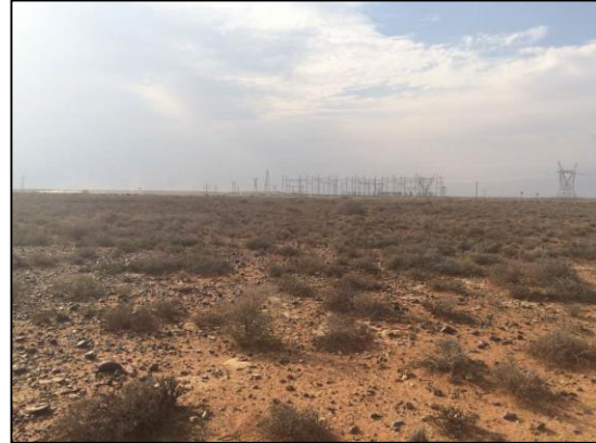
Figure 17 – View of northern corridor alignment with the Kronos substation in background
