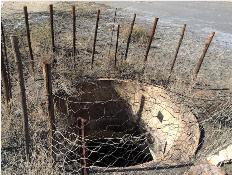
Figure 12 - Stone foundations for machinery at MS010
