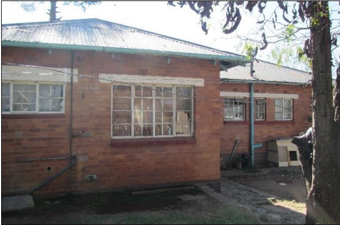
Figure 30: Closer view of one of the detached houses
