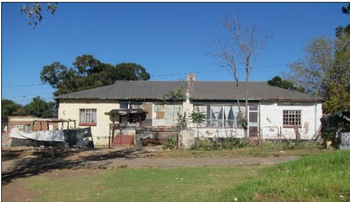
Figure 27: View of one of the semi-detached houses, showing the enclosed verandah
