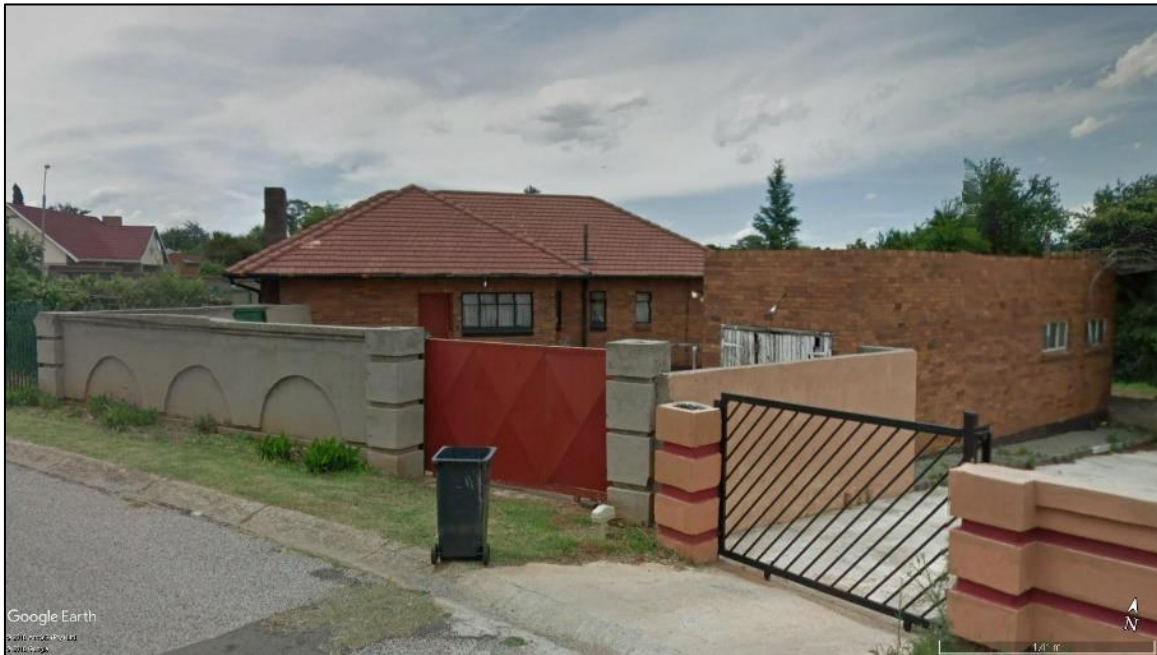
Figure 32: Site CP003, a different style of historical house in Creswell Park suburb
