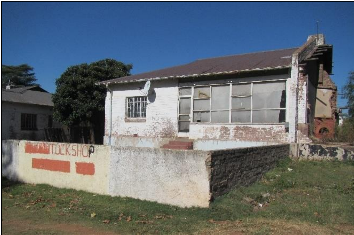
Figure 28: View of a half-demolished semi-detached house
