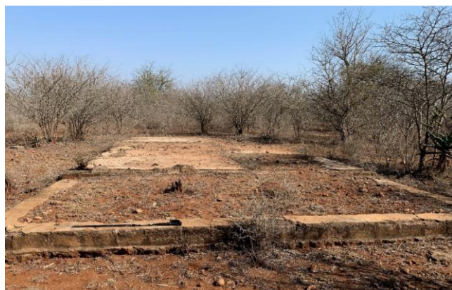
Figure 23 – General view of the floor foundation
