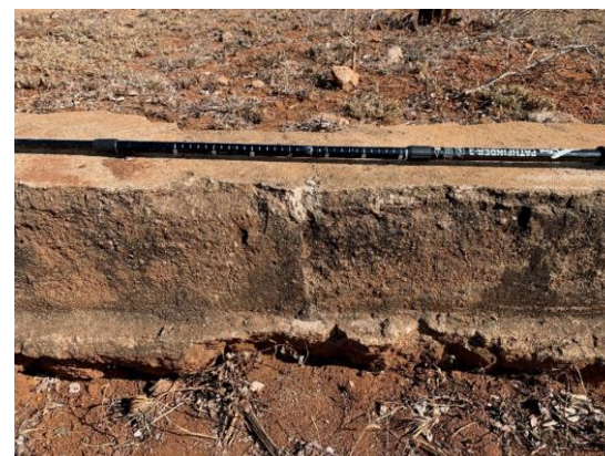
Figure 24 – Closer view of the foundation wall showing bricks and concrete
