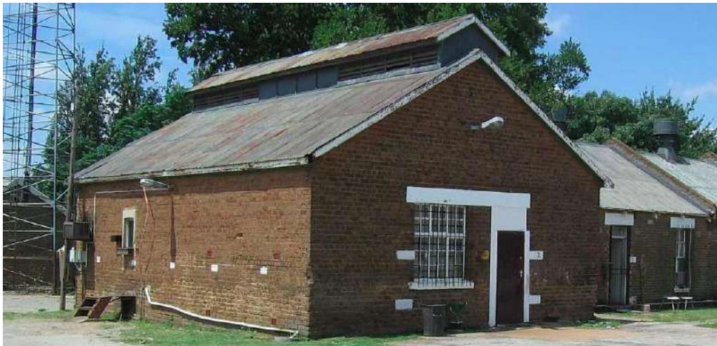
Figure 104 – General view of Building Type 60.
