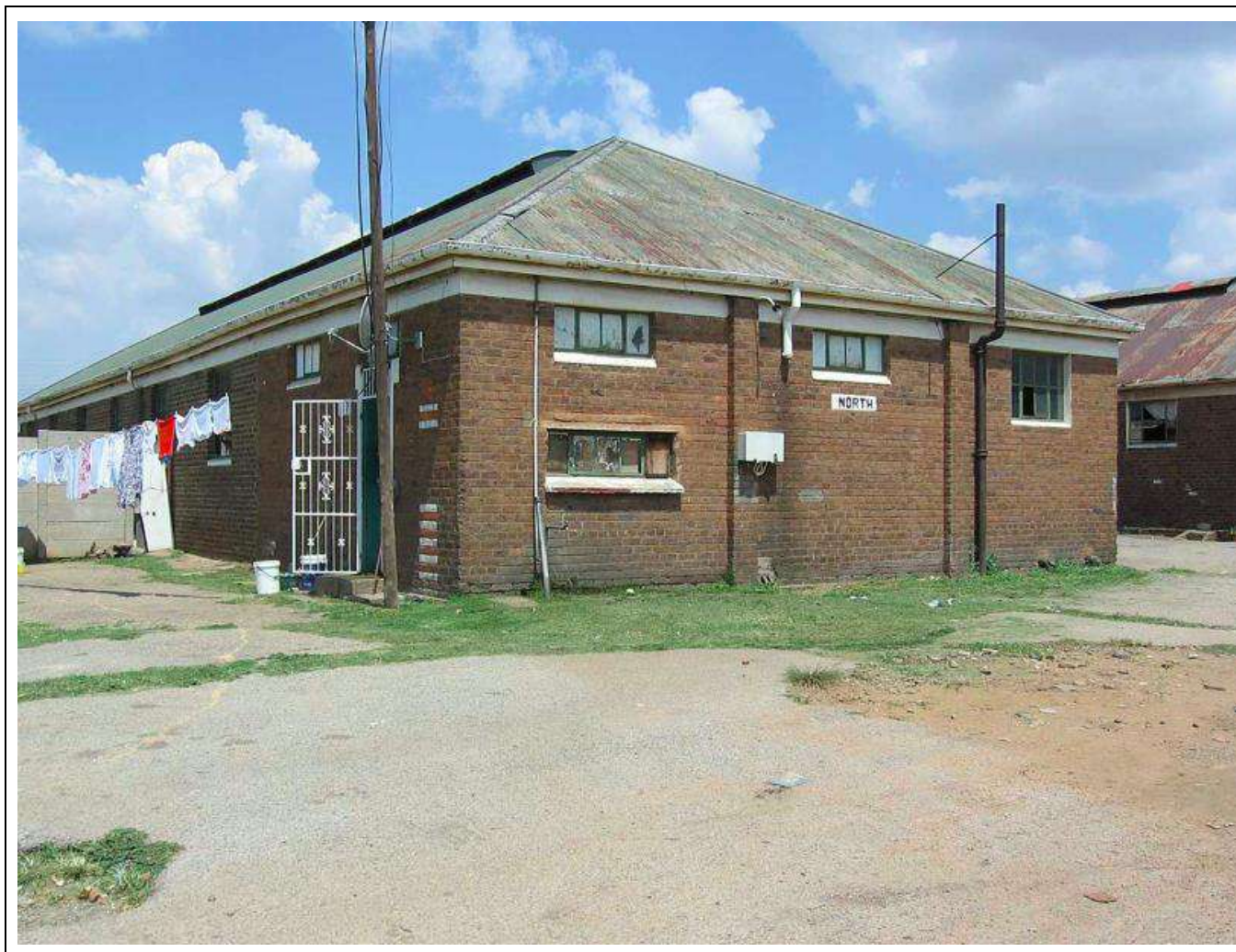
Figure 101 – General view of Building Type 57.
