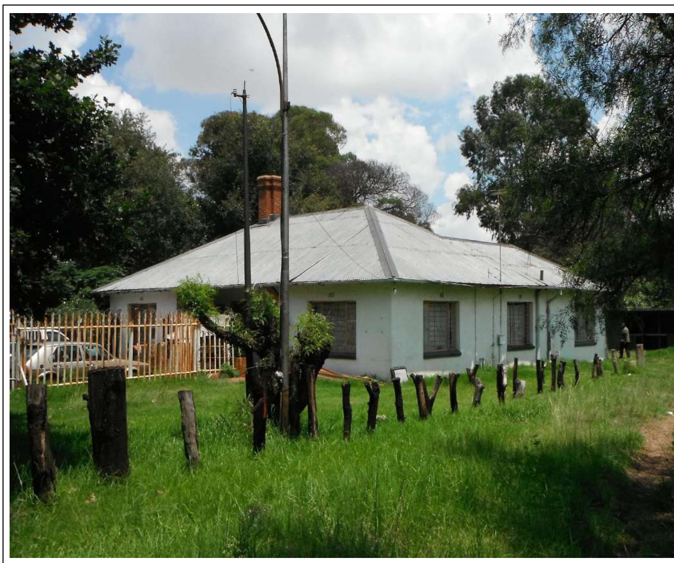
Figure 74 – General view of Building Type 31.
