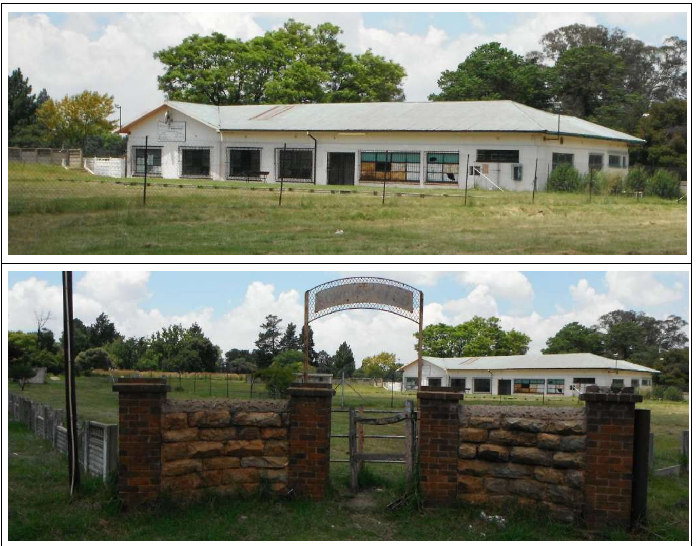
Figure 71 – General views of the structure as well as the main entrance gate at Building Type 29 .
