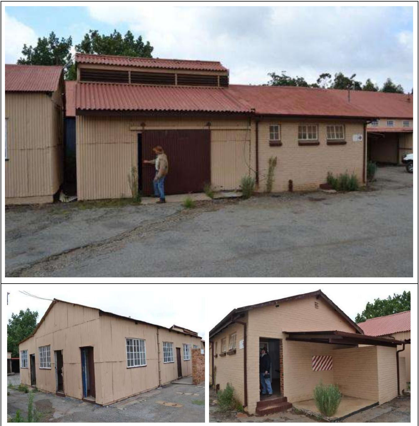
Figure 112 – General views of Building Type 71.
