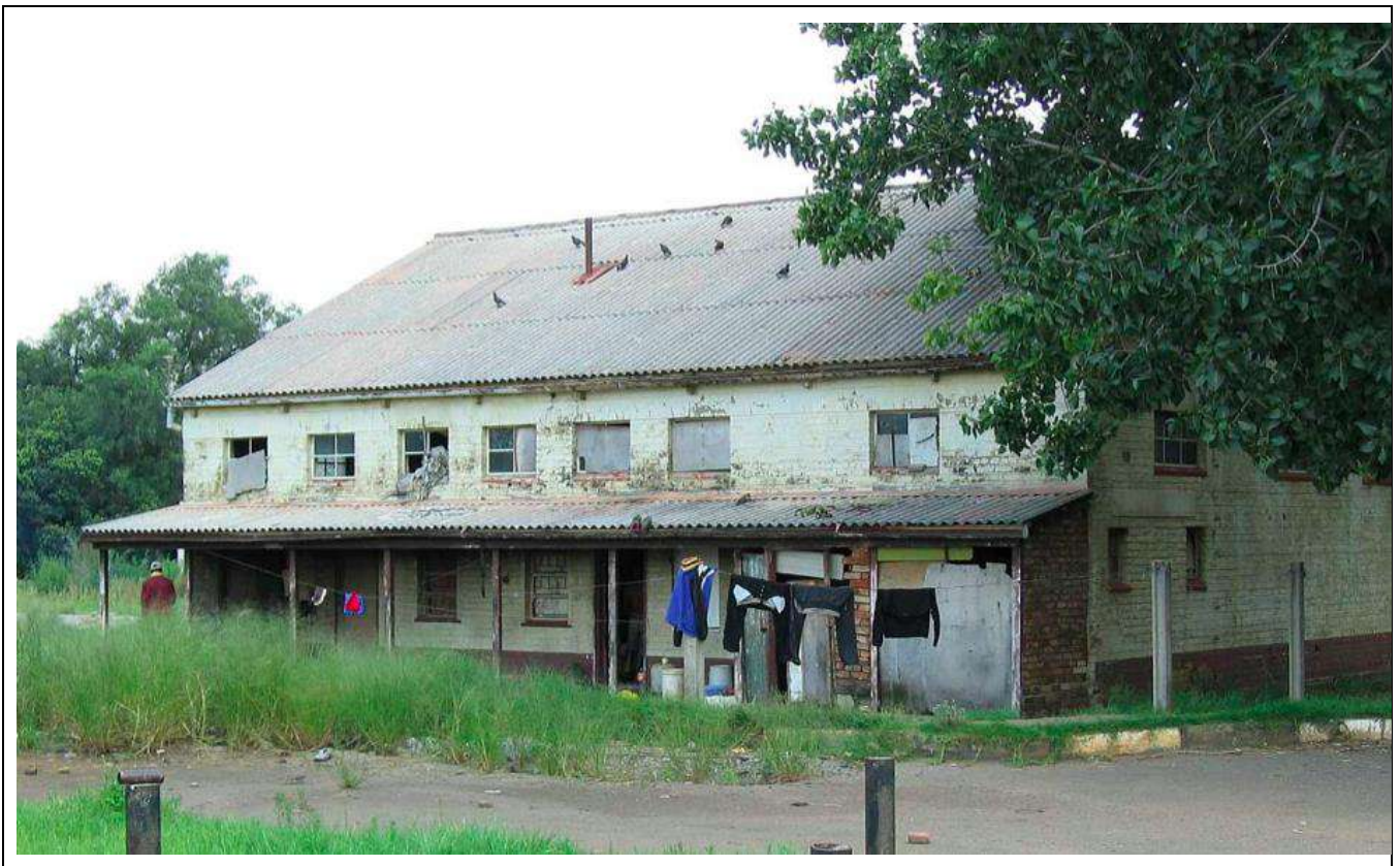
Figure 99 – General view of Building Type 54.
