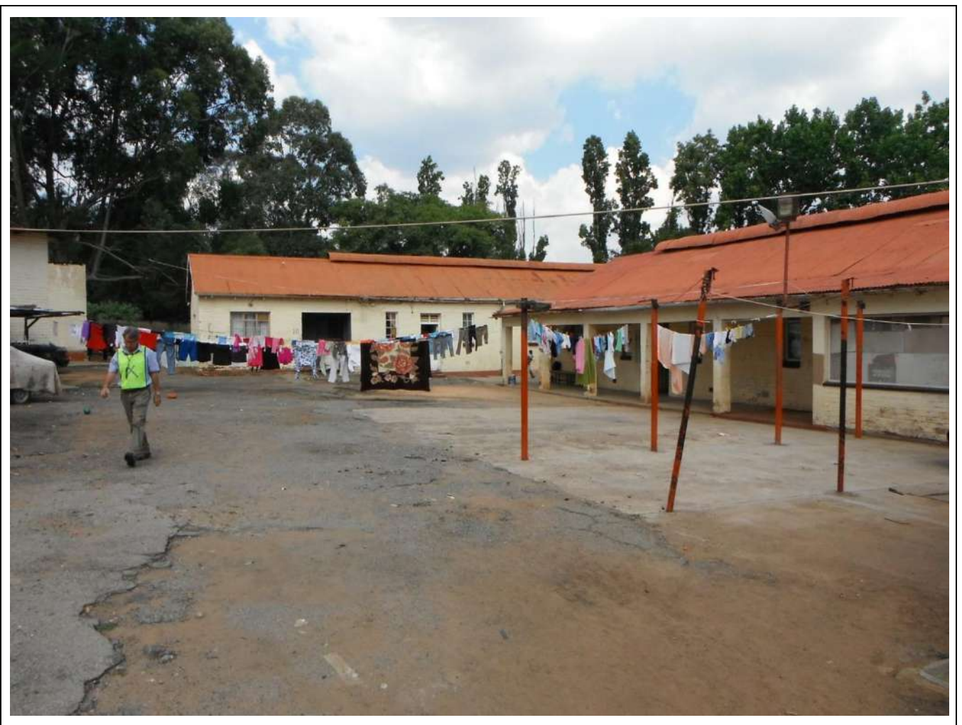
Figure 92 – General view of Building Type 48.
