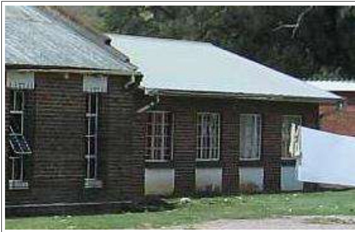
Figure 106 – General view of Building Type 62.
