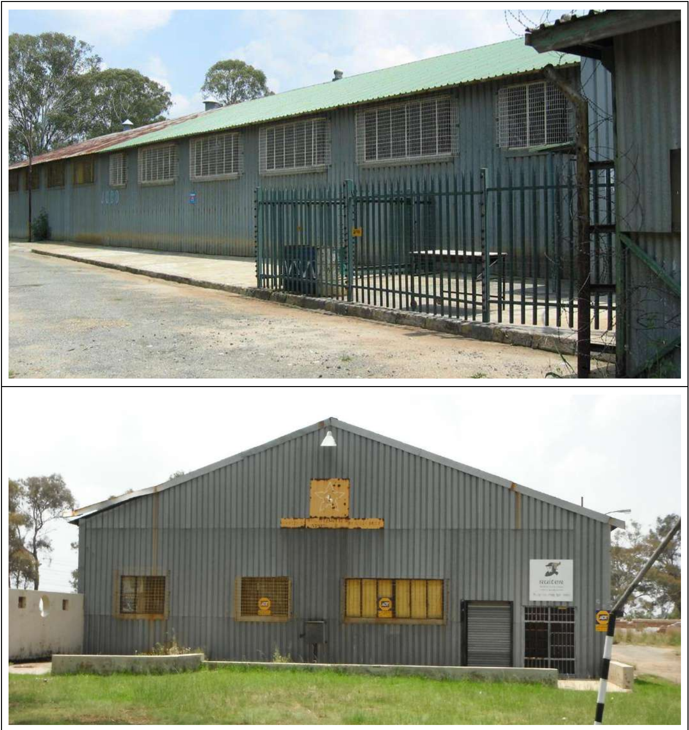
Figure 52 – General views of Building Type 15.
