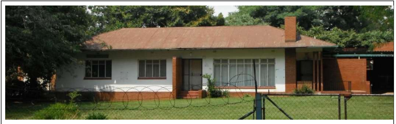
Figure 41 – General view of Building Type 4.
