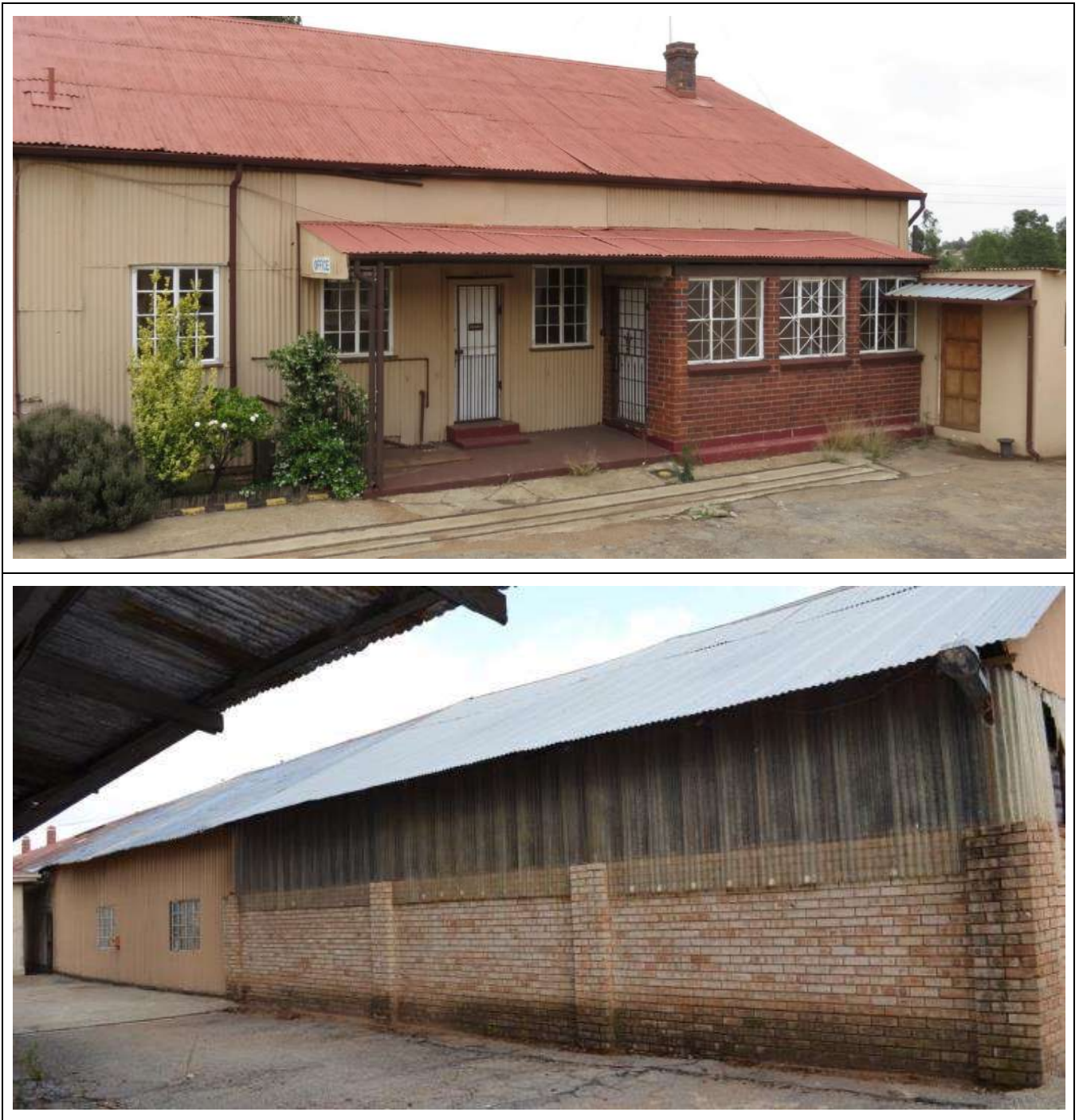
Figure 117 – General views of Building Type 76.
