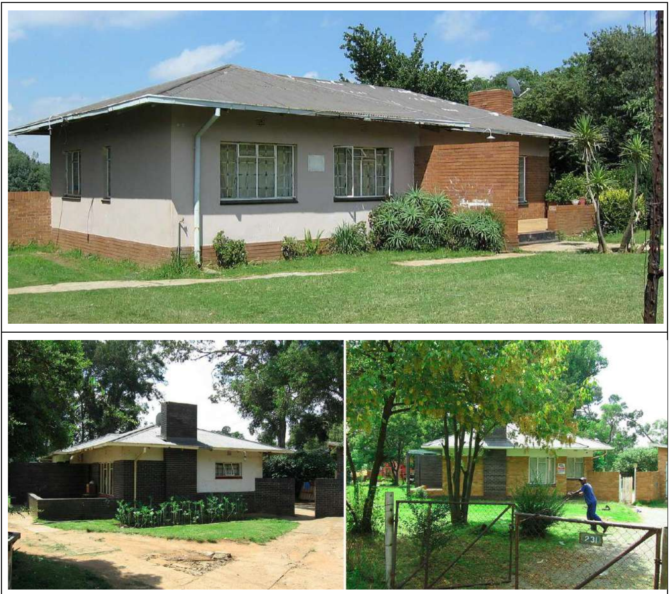
Figure 62 – General views of Building Type 21.
