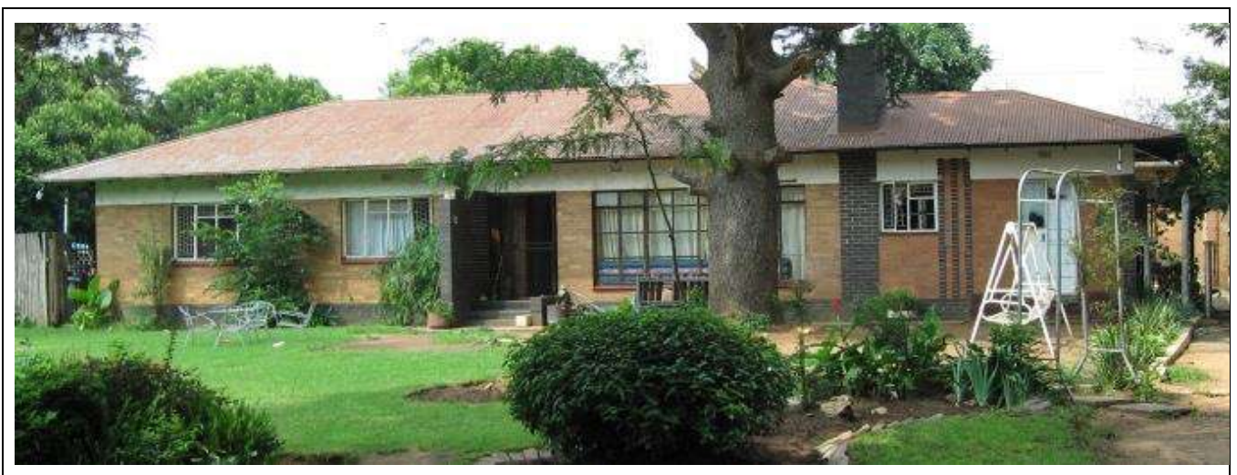
Figure 42 – General view of Building Type 5.
