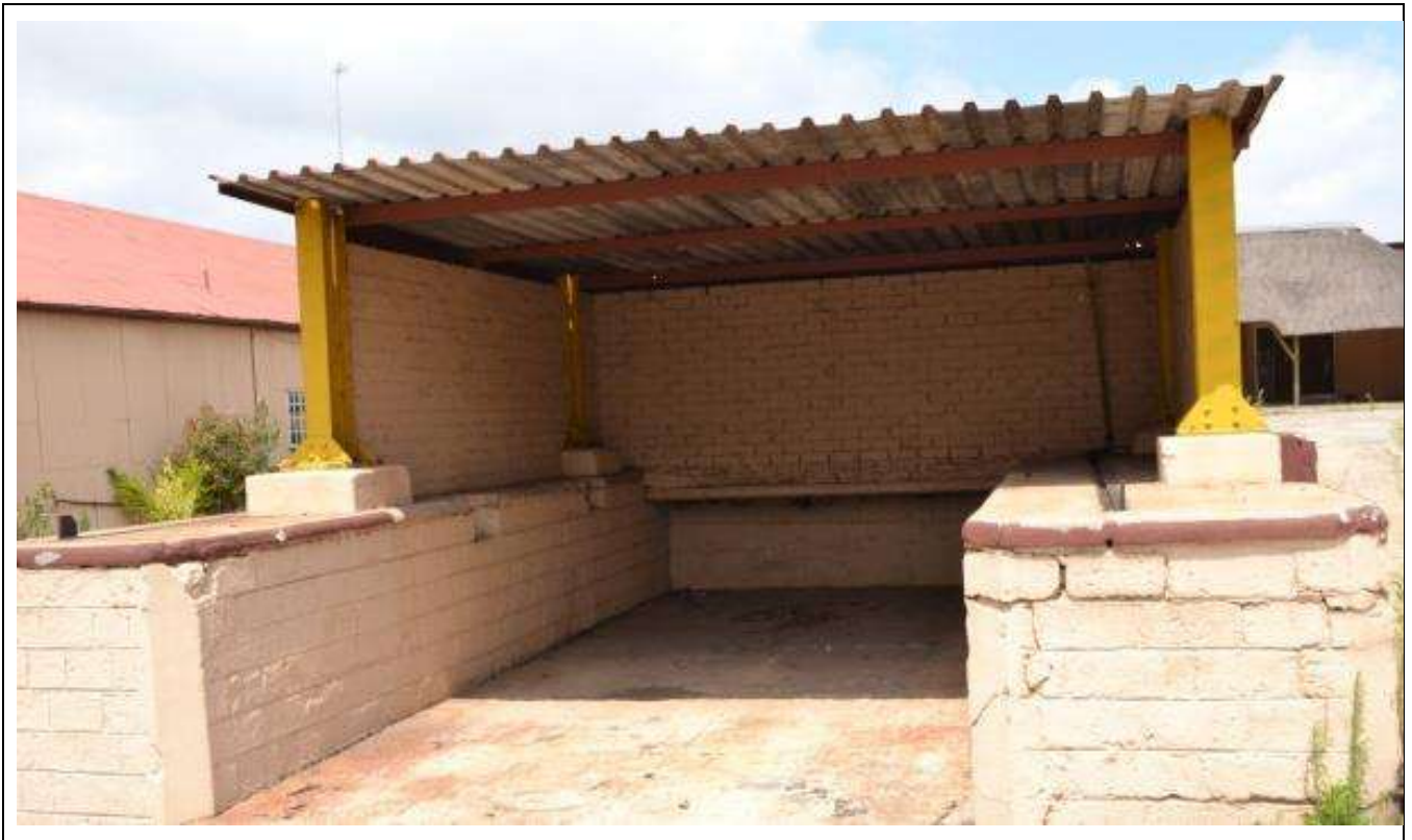
Figure 121 – General view of Building Type 80.
