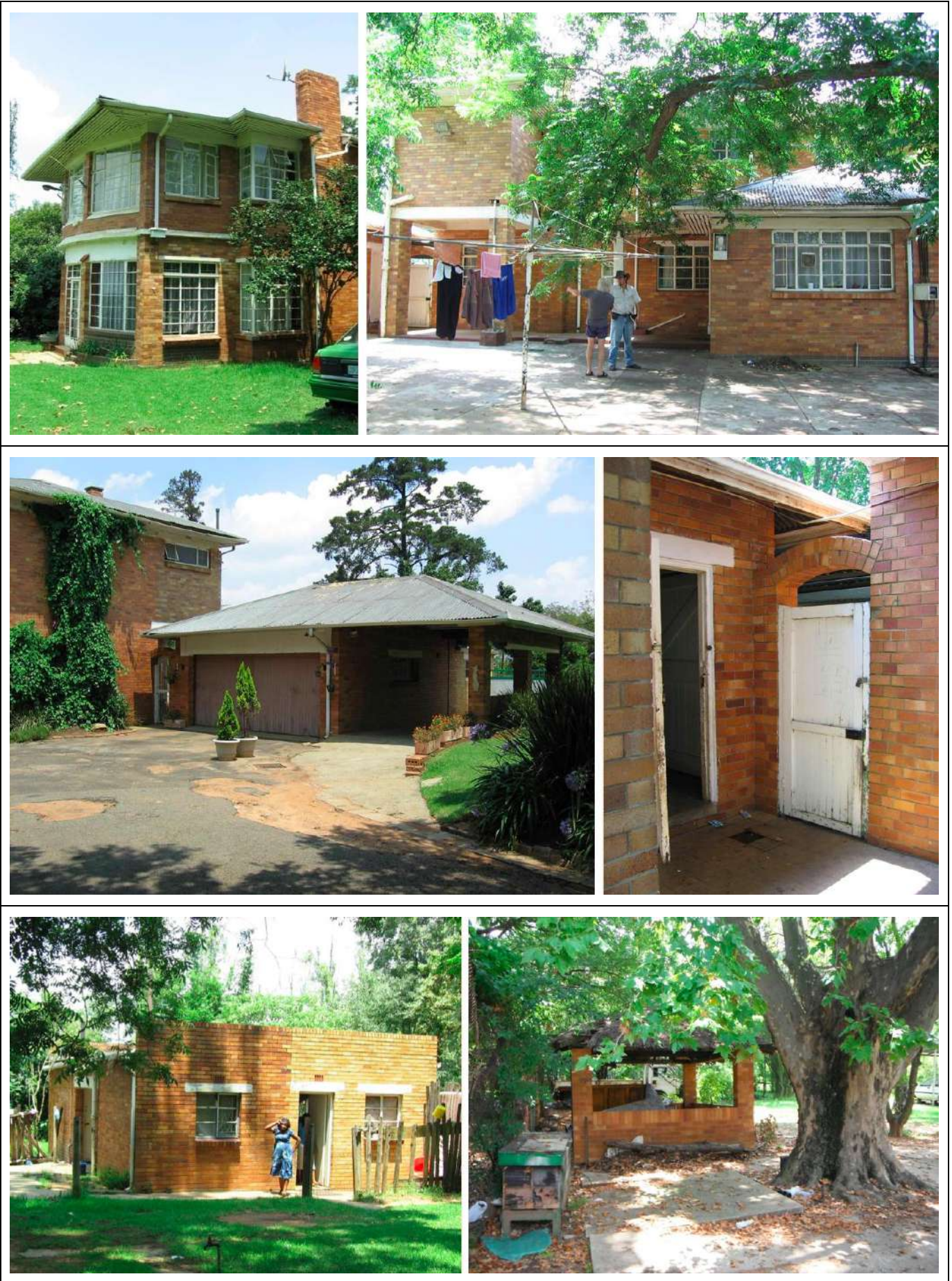
Figure 55 – General and detail views of Building Type 17.
