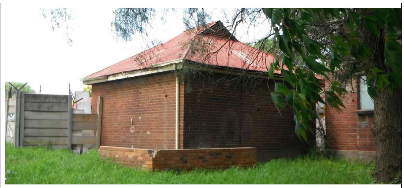
Figure 88 – General view of Building Type 44.
