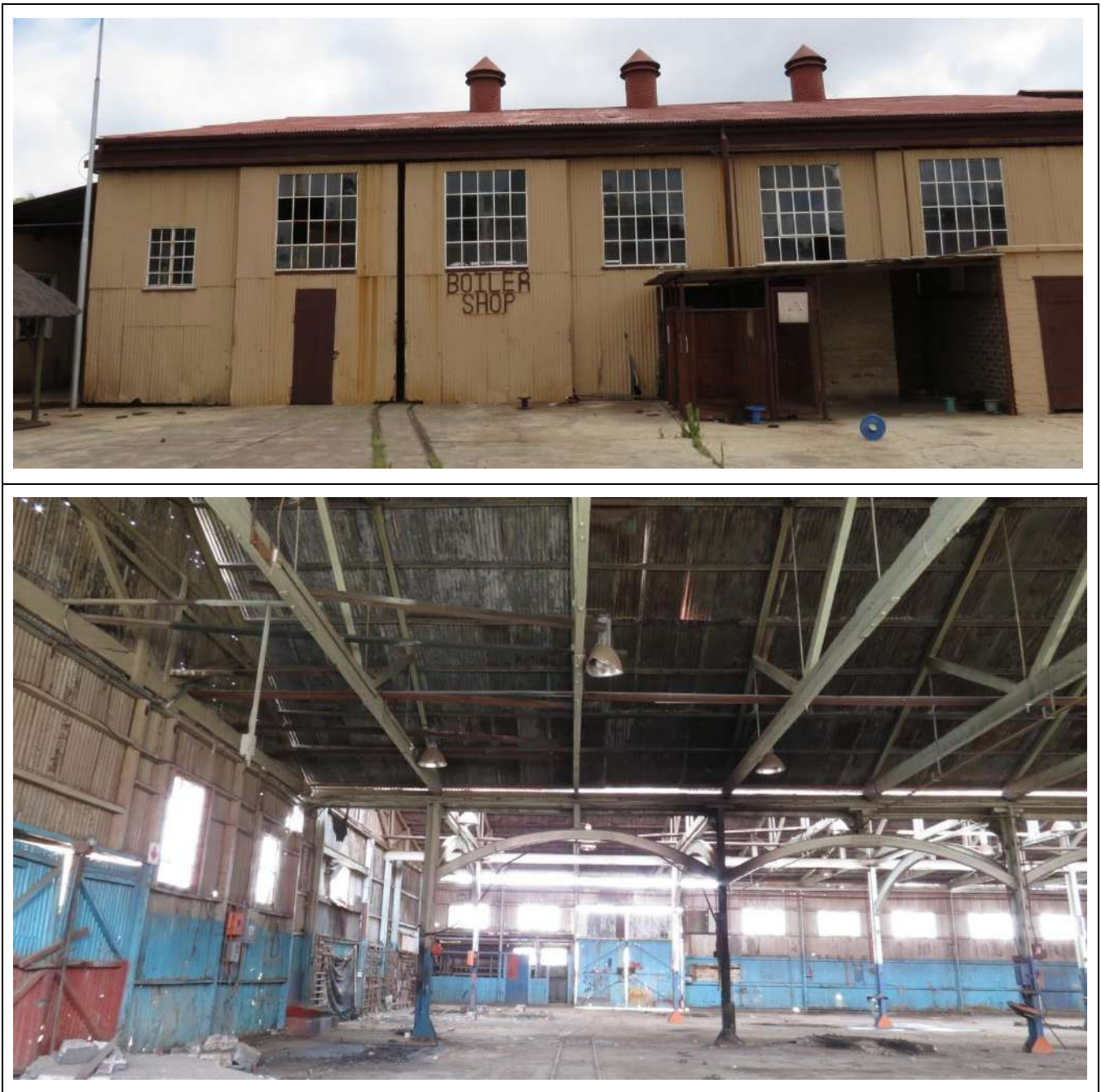
Figure 110 – General views of the exterior and interior of Building Type 69.
