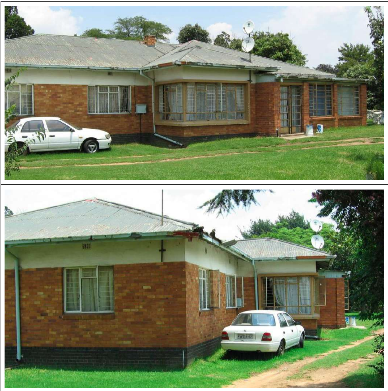
Figure 50 – General views of Building Type 13.
