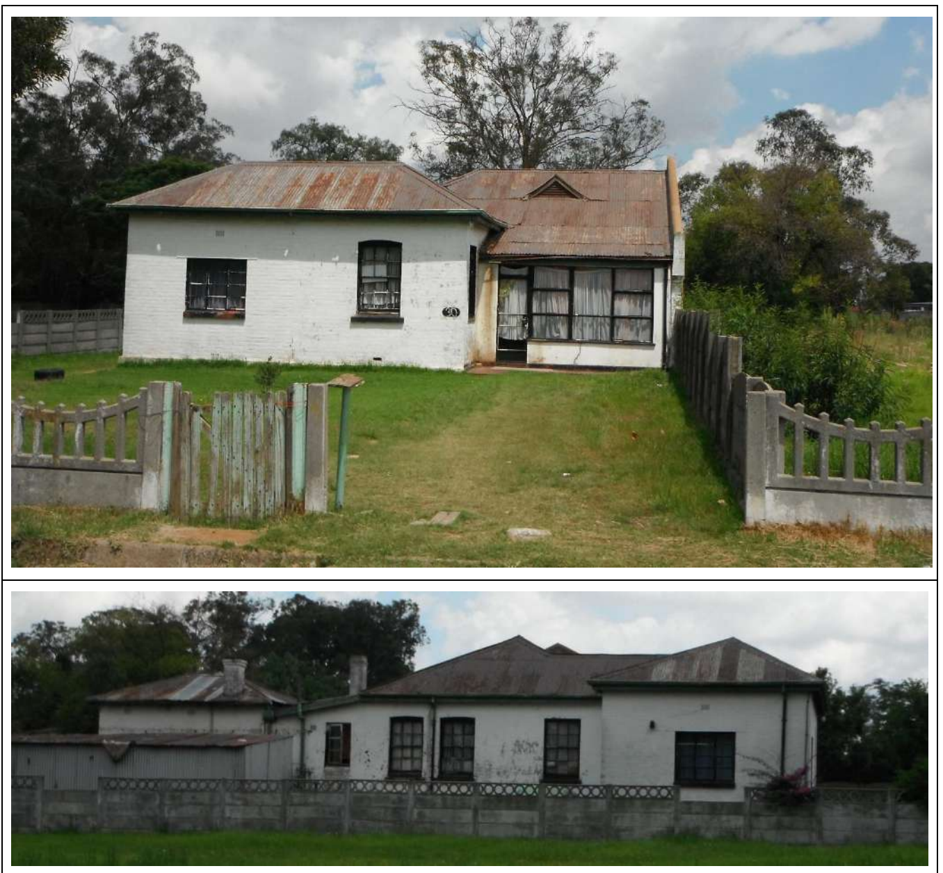
Figure 80 – General view of Building Type 37.
