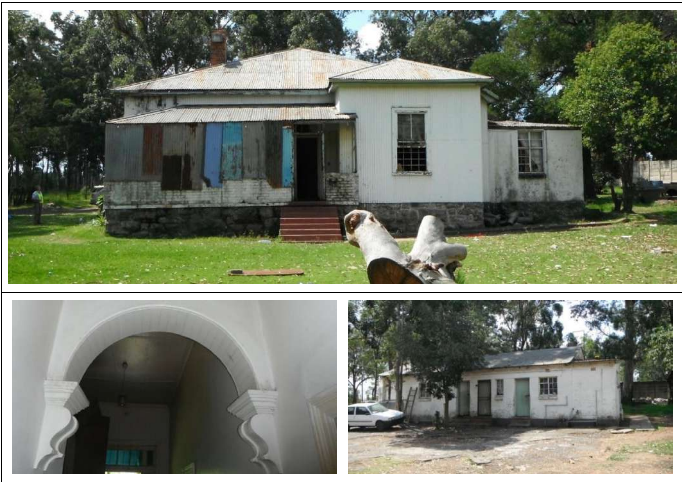
Figure 76 – General views of Building Type 33.
