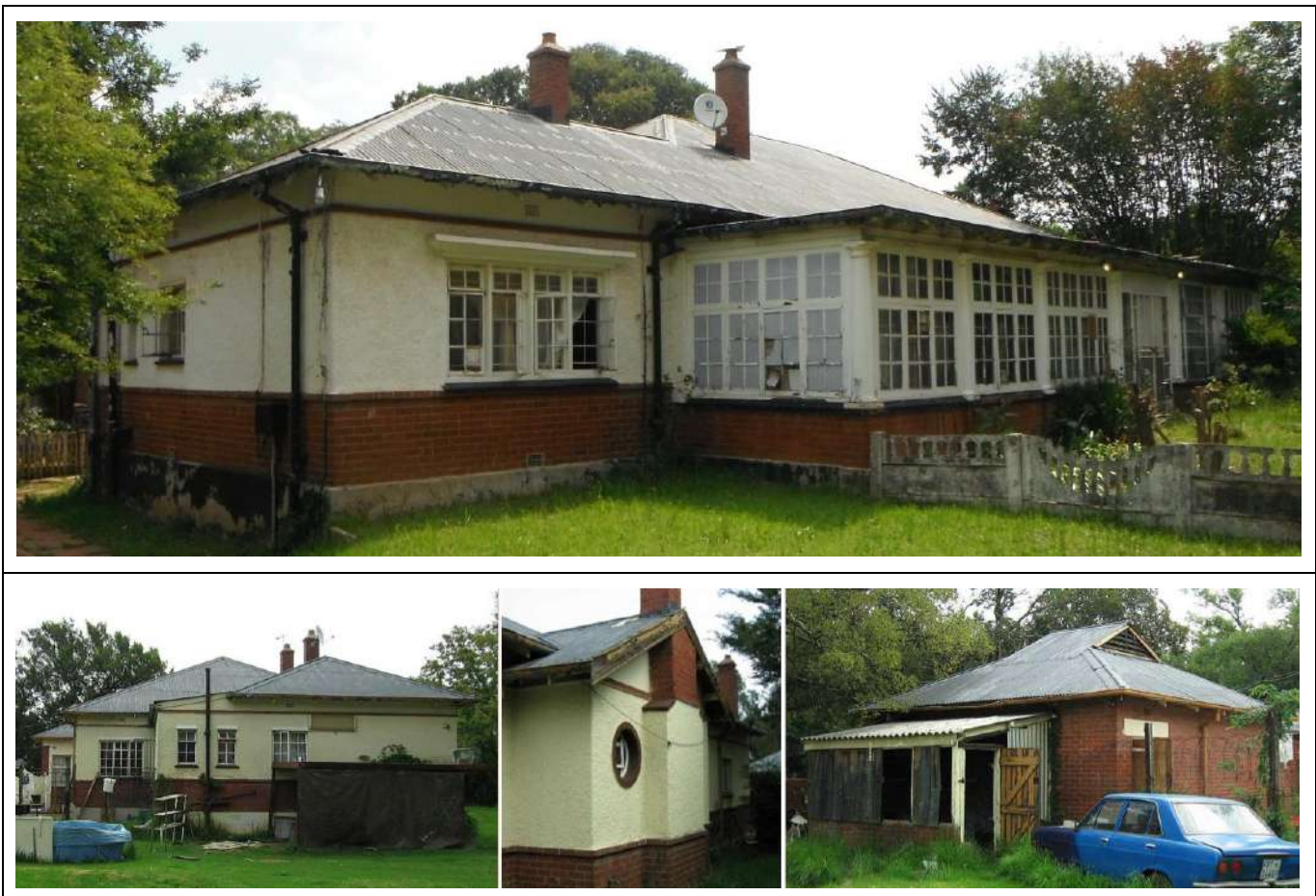
Figure 56 – General and detail views of Building Type 18.
