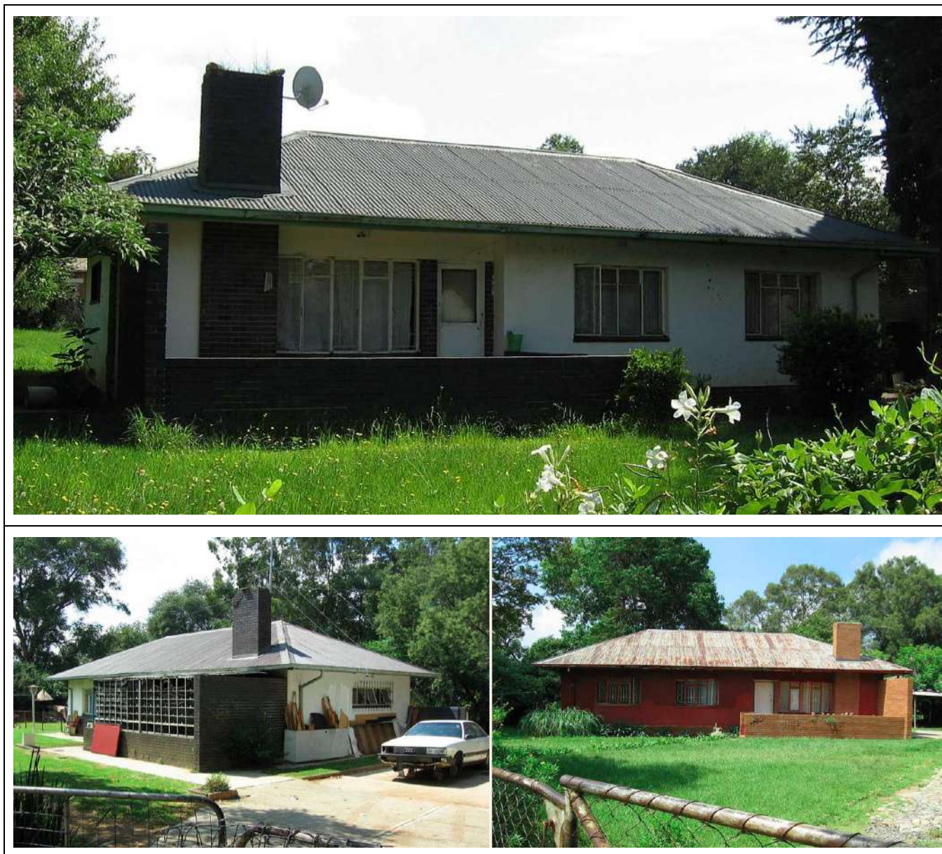
Figure 61 – General views of Building Type 20.
