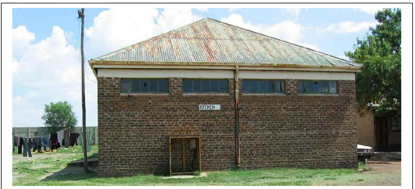
Figure 103 – General view of Building Type 59.
