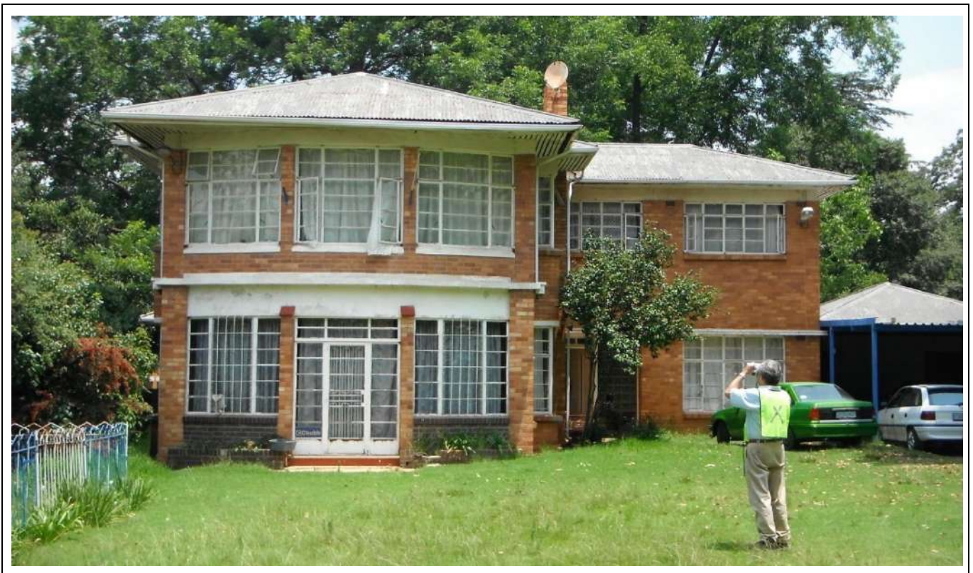
Figure 54 – The front façade of one of the examples of Building Type 17.
