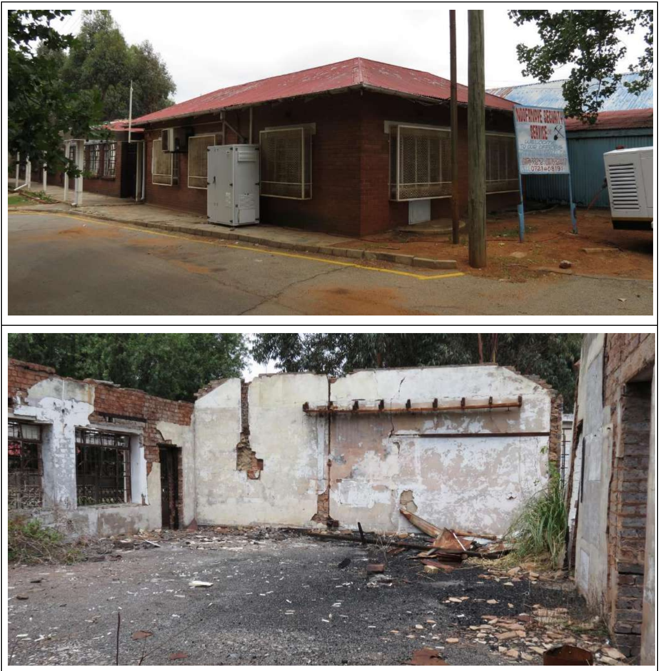
Figure 124 – General views of Building Type 83.
