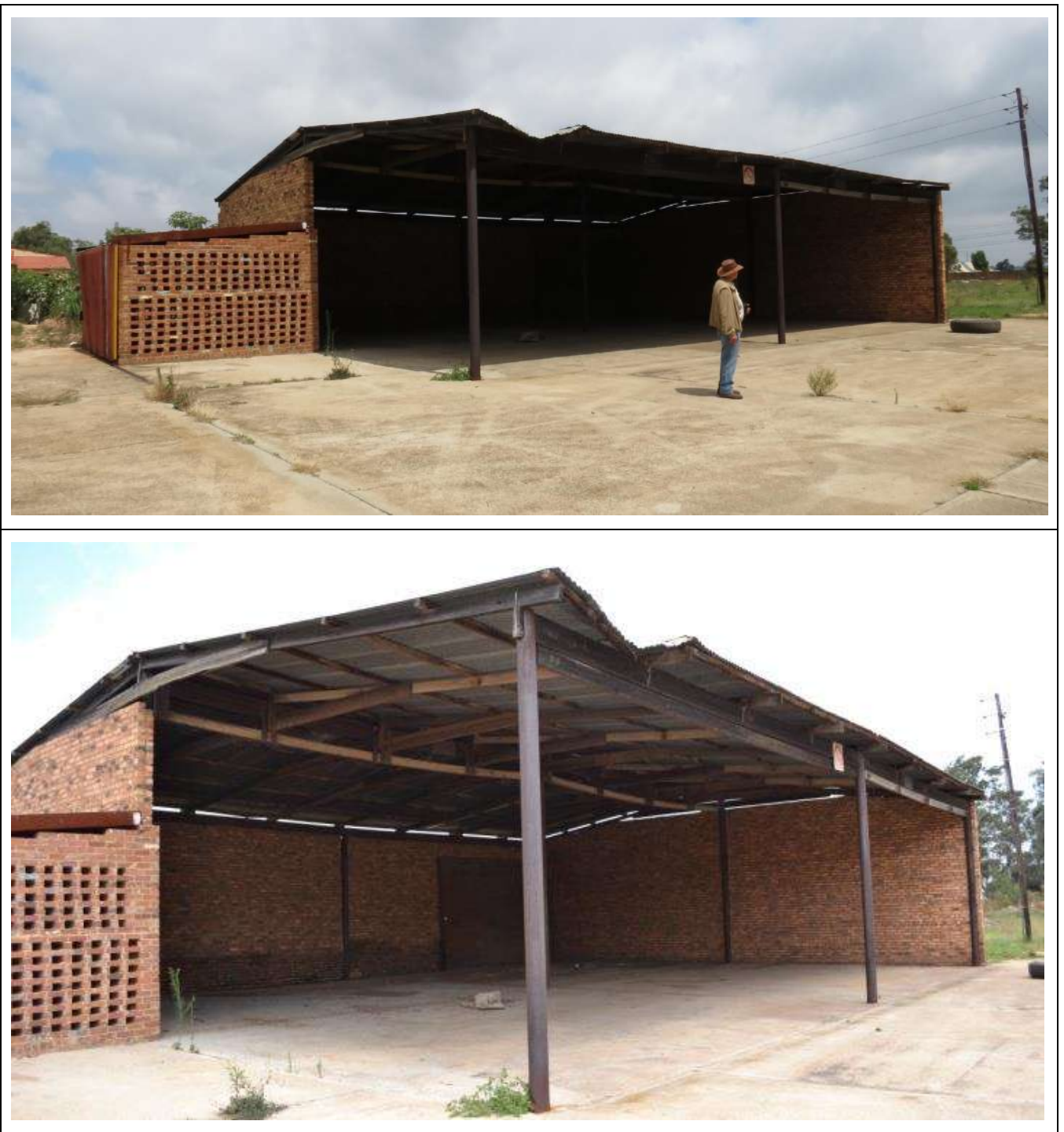
Figure 118 – General views of Building Type 77.
