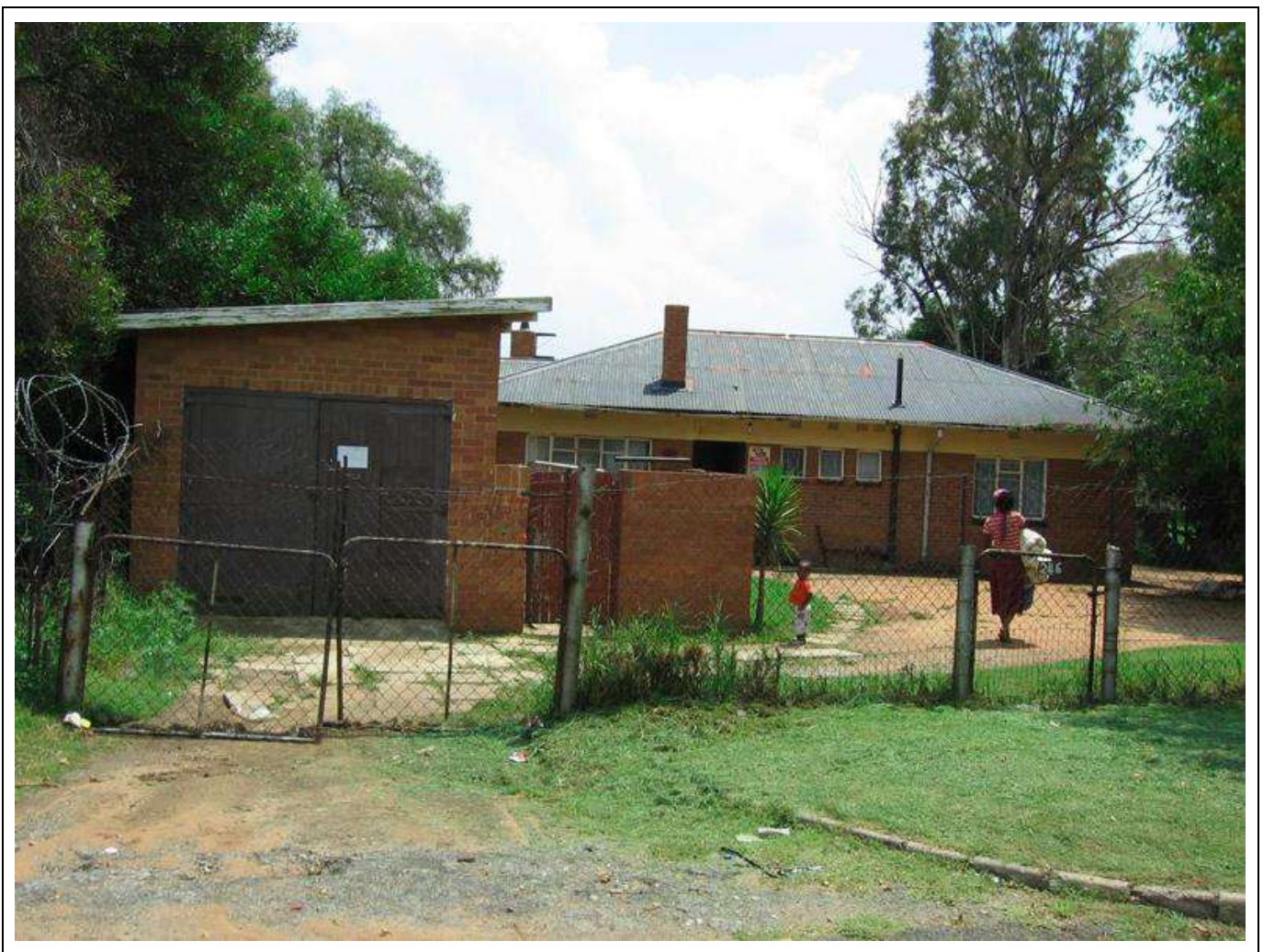
Figure 47 – General view of Building Type 10.
