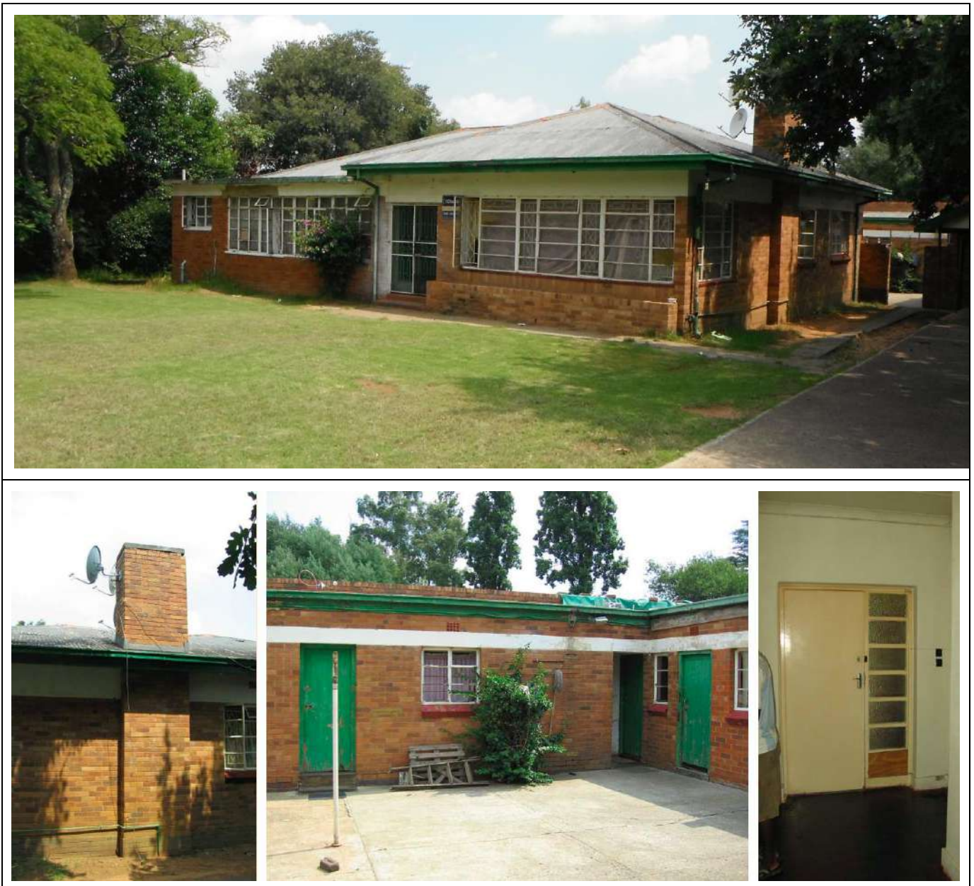
Figure 57 – General and detail views of Building Type 19.
