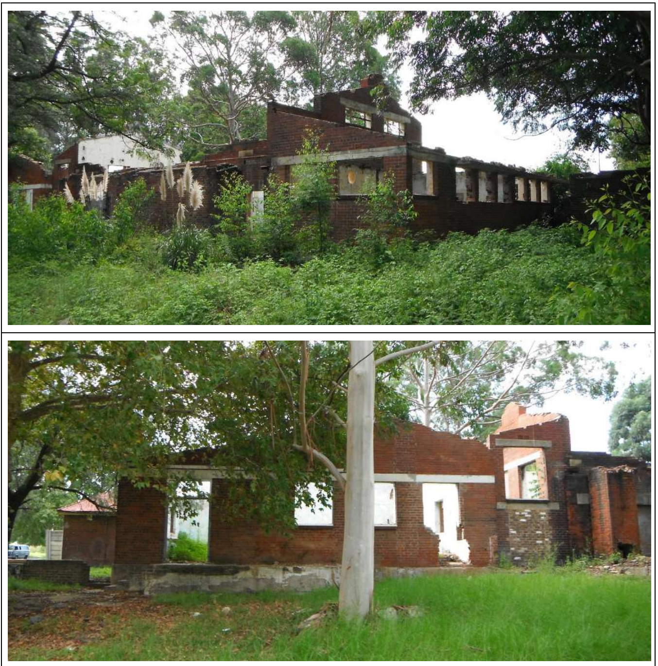
Figure 89 – General view of Building Type 45.
