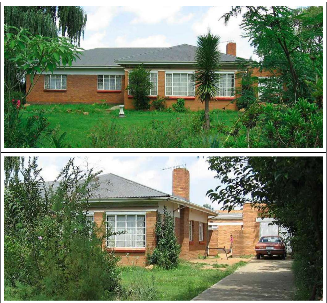
Figure 67 – General views of Building Type 26.
