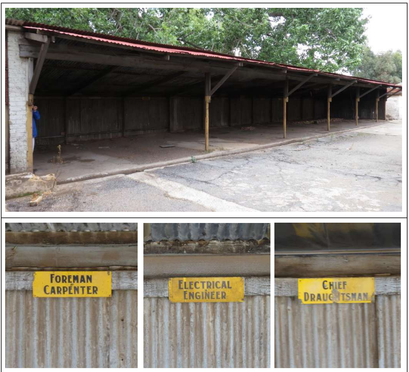
Figure 116 – General views of Building Type 75.
