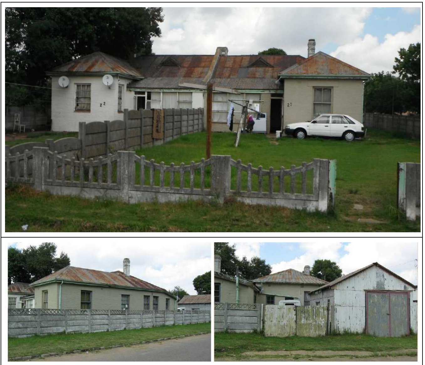
Figure 79 – General view of Building Type 36.
