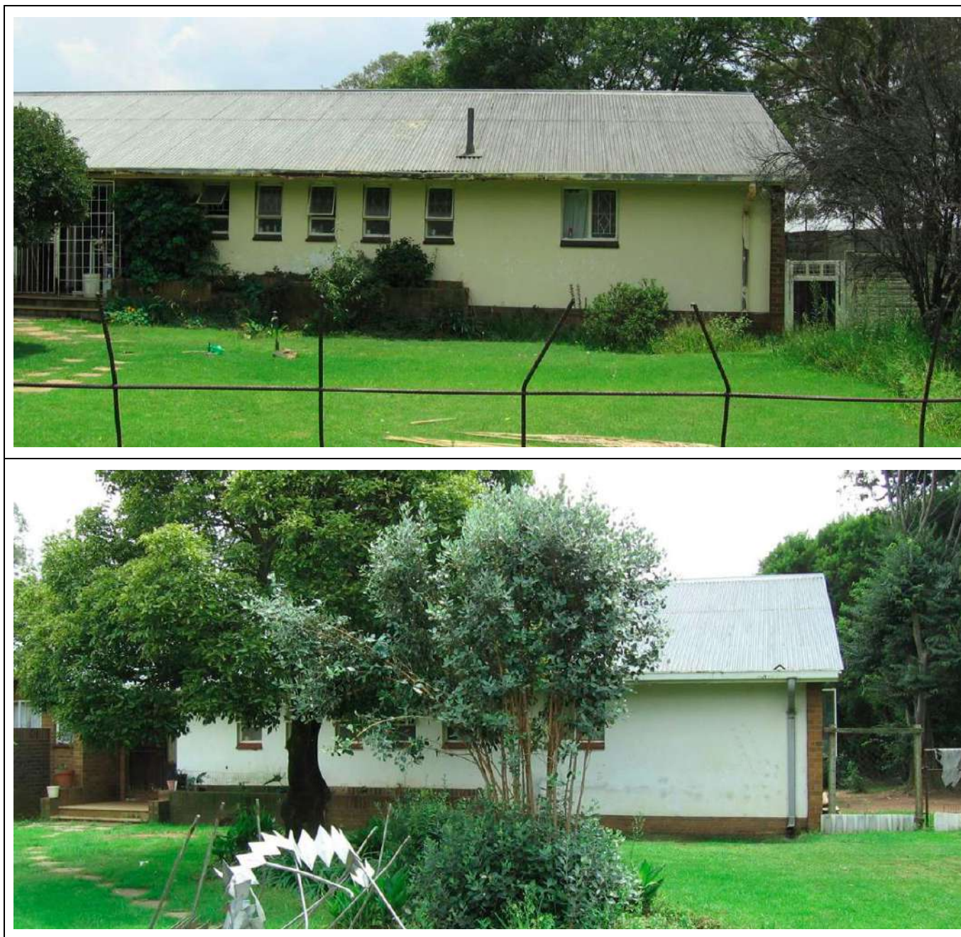
Figure 48 – General views of Building Type 11.
