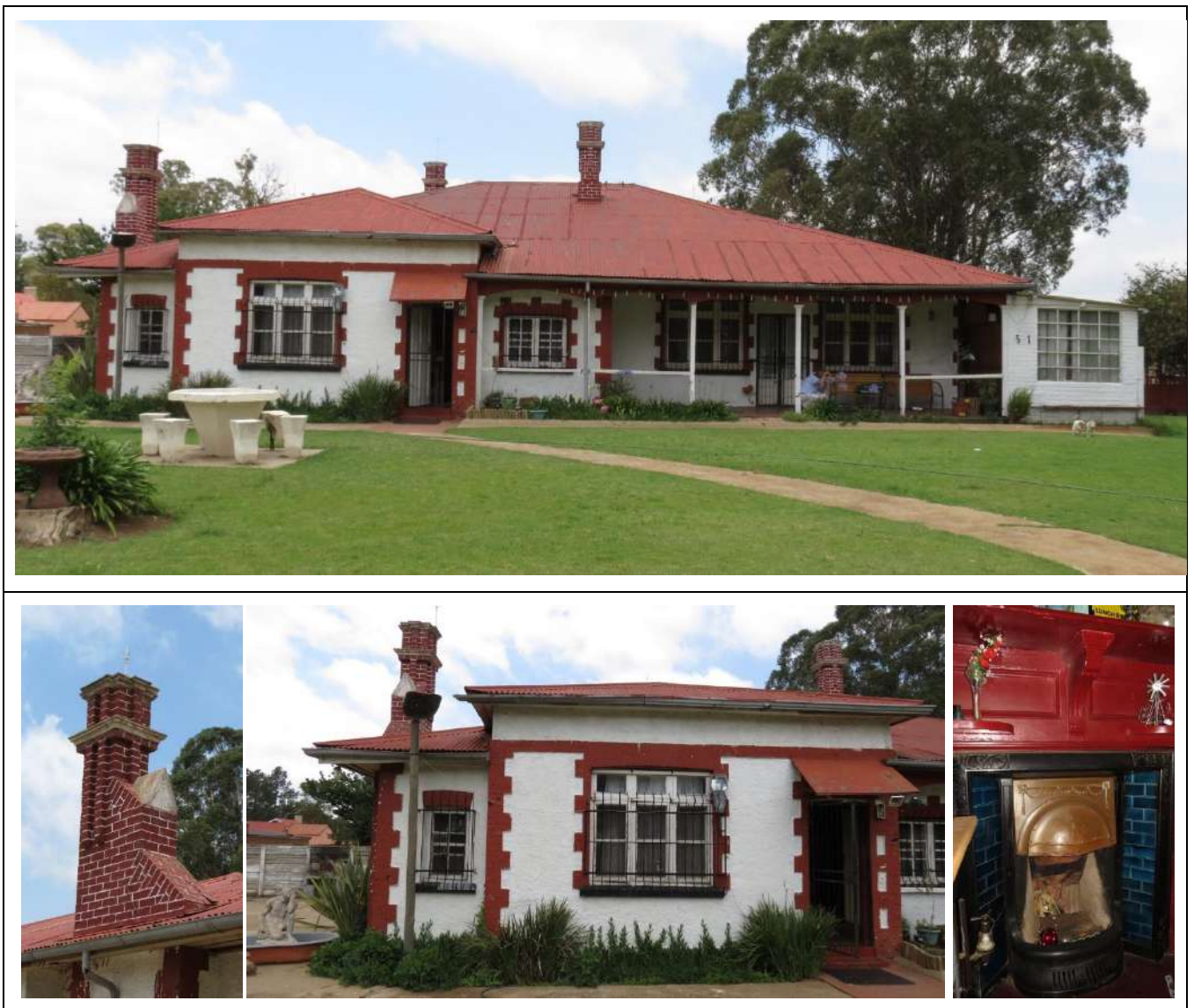
Figure 109 – General views of Building Type 68.
