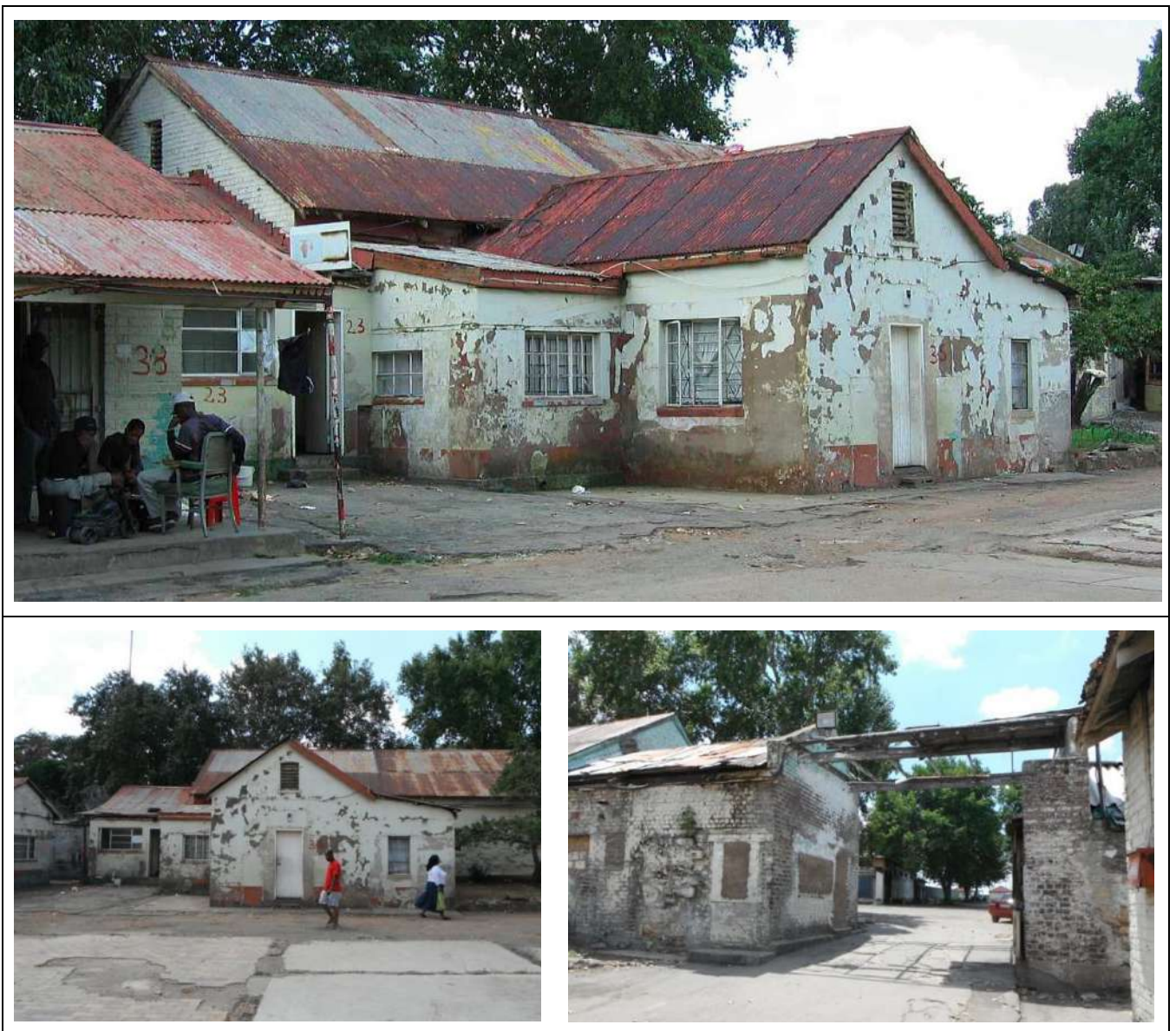
Figure 97 – General views of Building Type 52.
