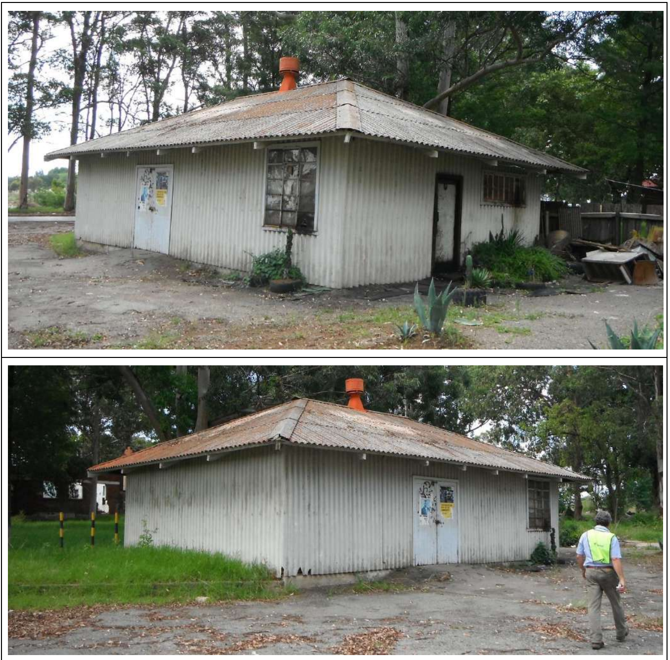
Figure 91 – General views of Building Type 47.
