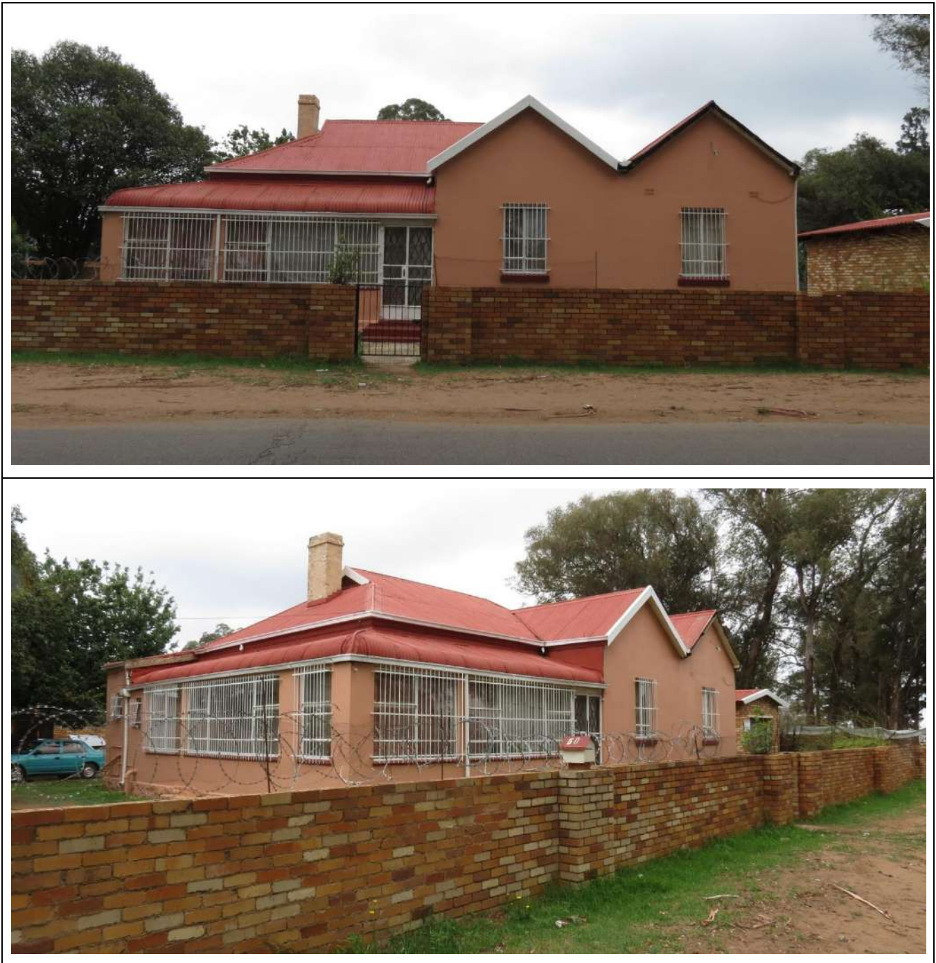
Figure 126 – General views of Building Type 85.
