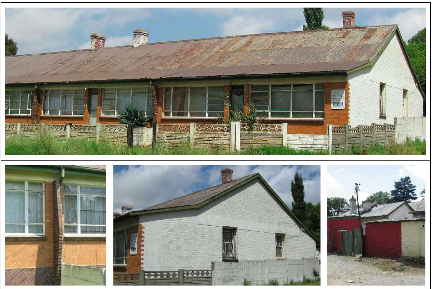
Figure 68 – General and detail views of Building Type 27.
