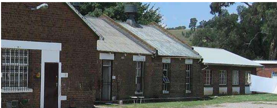
Figure 105 – General view of Building Type 61.
