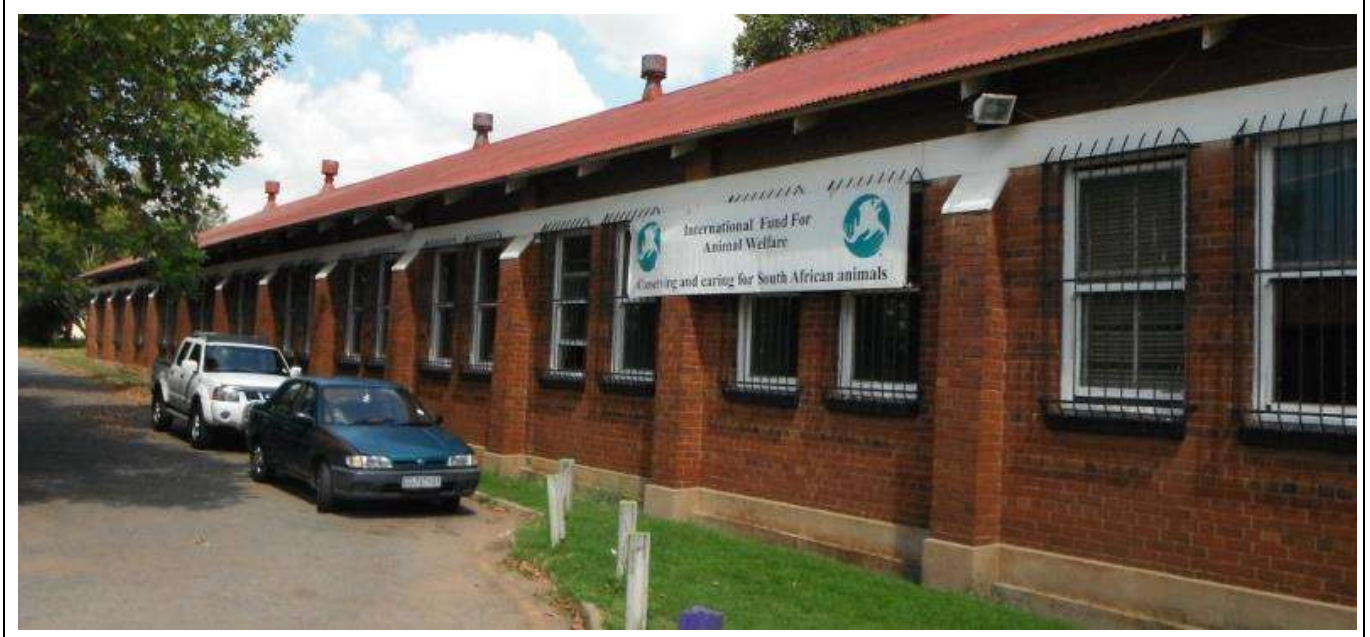
Figure 83 – General views of Building Type 39.
