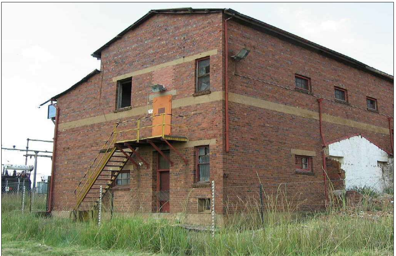
Figure 128 – General view of the electrical substation included in this report as Building Type 55. This photograph was taken during the fieldwork of December 2013.
