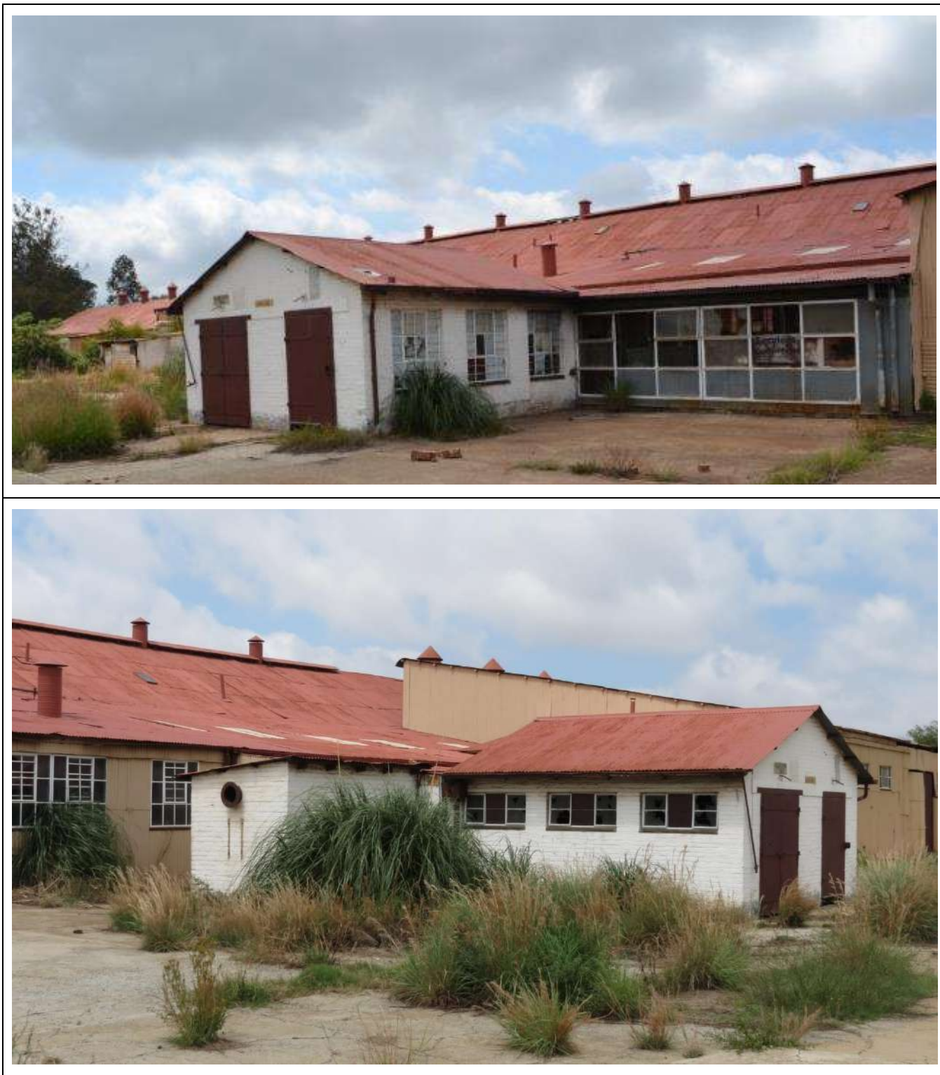
Figure 120 – General views of Building Type 79.
