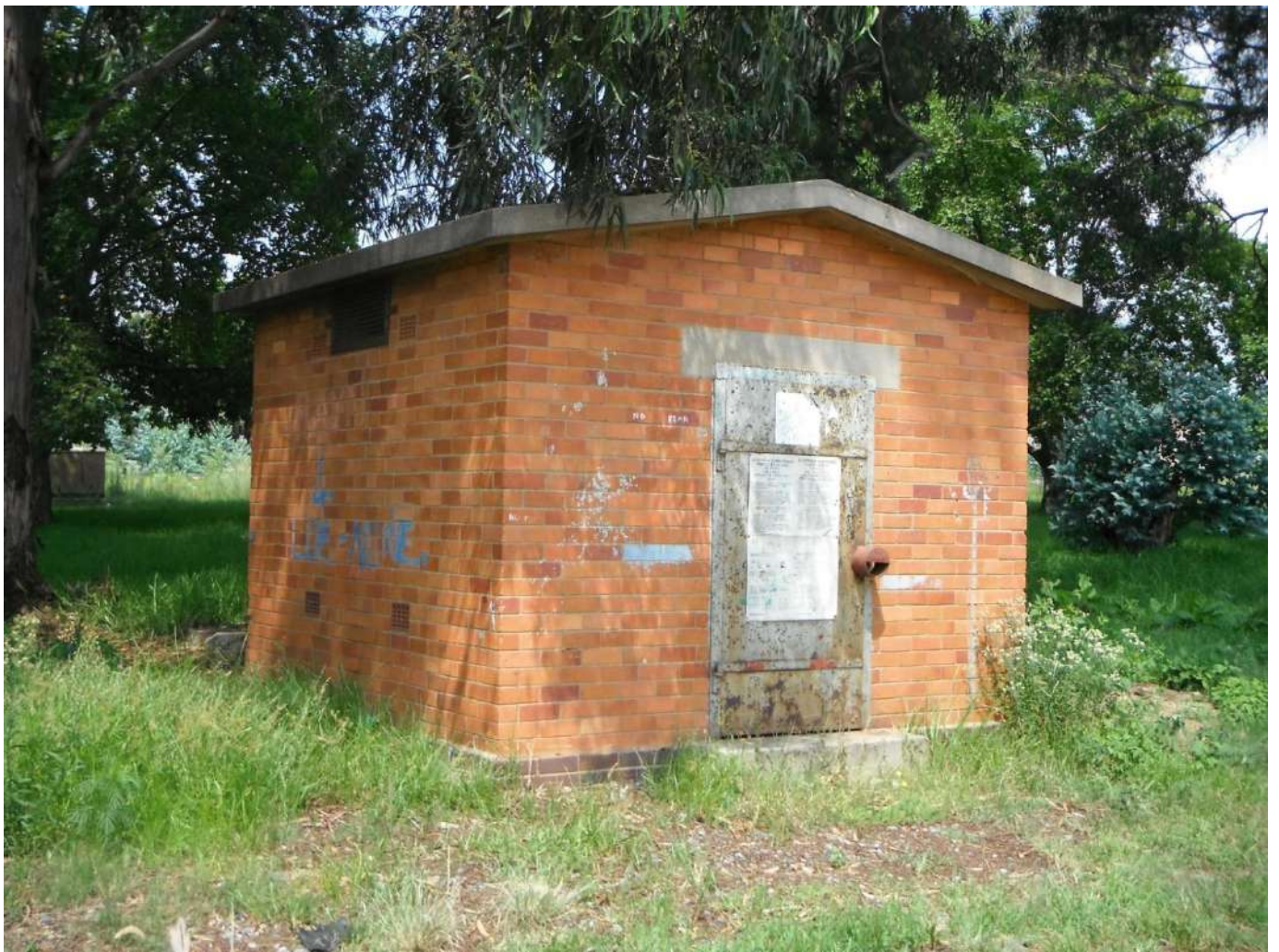
Figure 45 – General view of Building Type 8.
