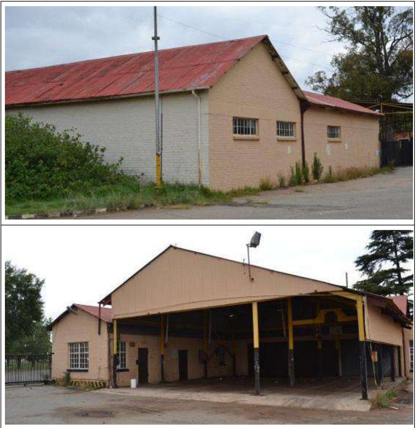
Figure 113 – General views of Building Type 72.
