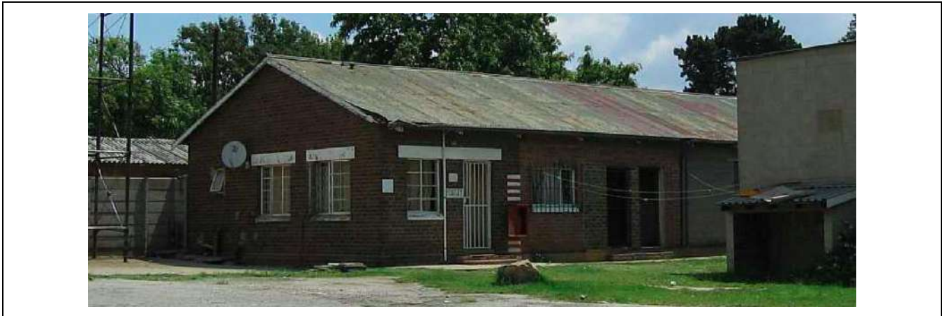
Figure 102 – General view of Building Type 58.
