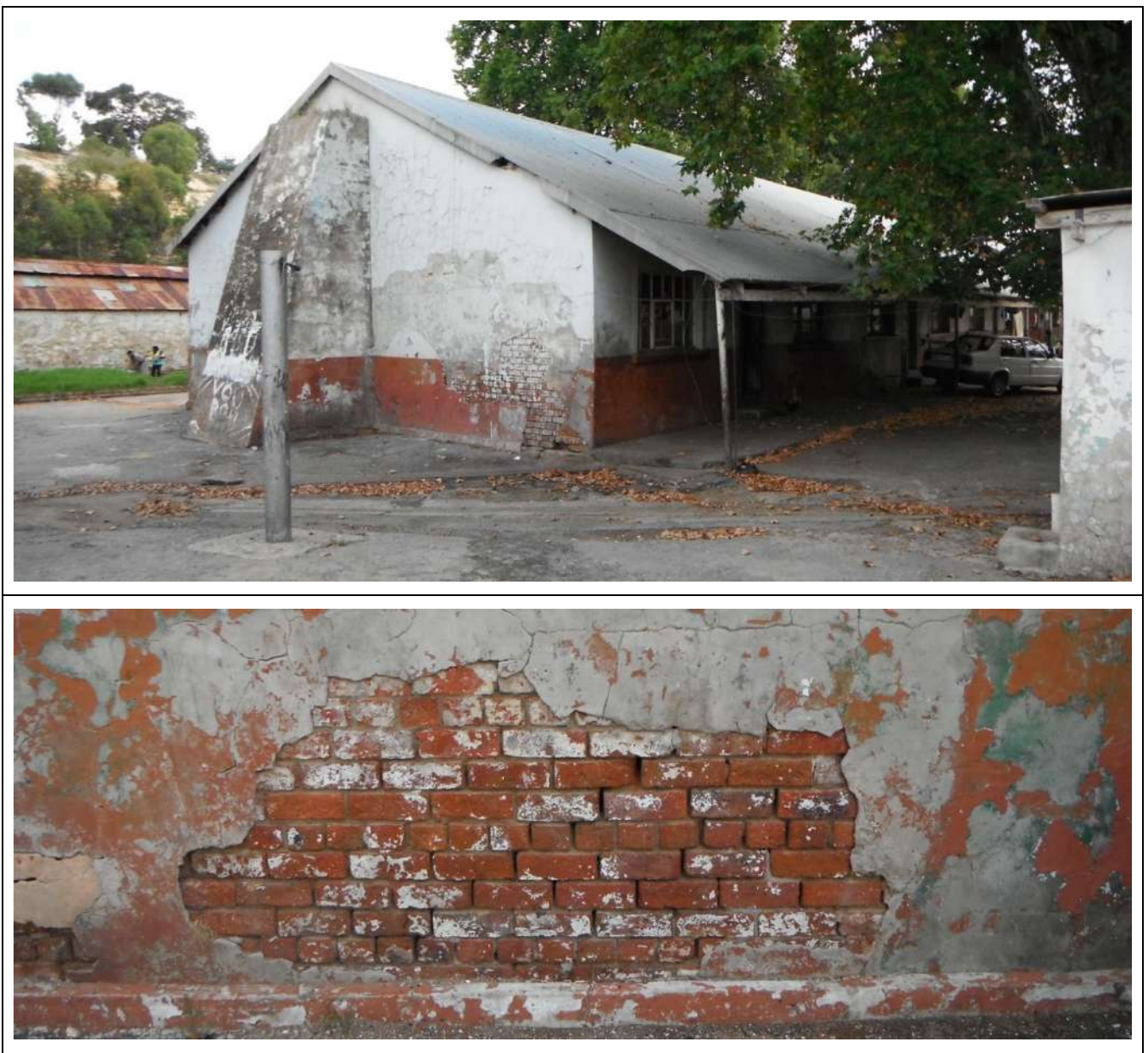
Figure 96 – General views of Building Type 51.
