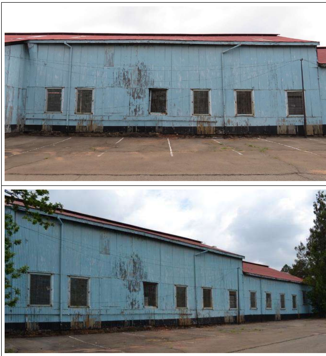
Figure 122 – General views of Building Type 81.
