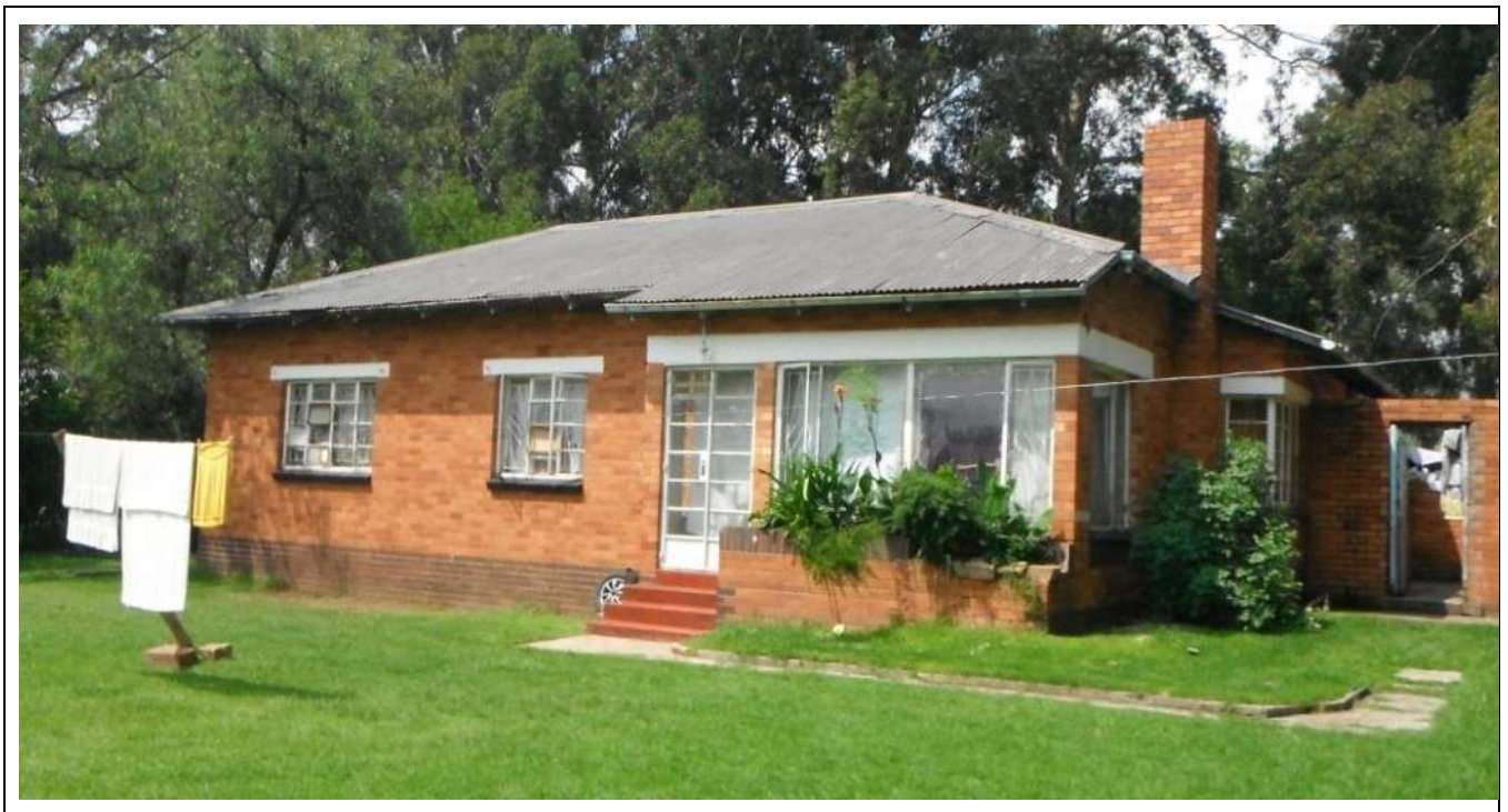
Figure 38 – General view of the front (northern) façade of one of the buildings classified as a Building Type 1 structure.
