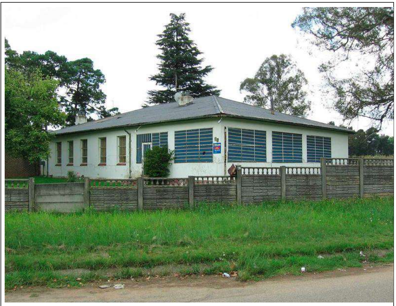
Figure 78 – General view of Building Type 35.
