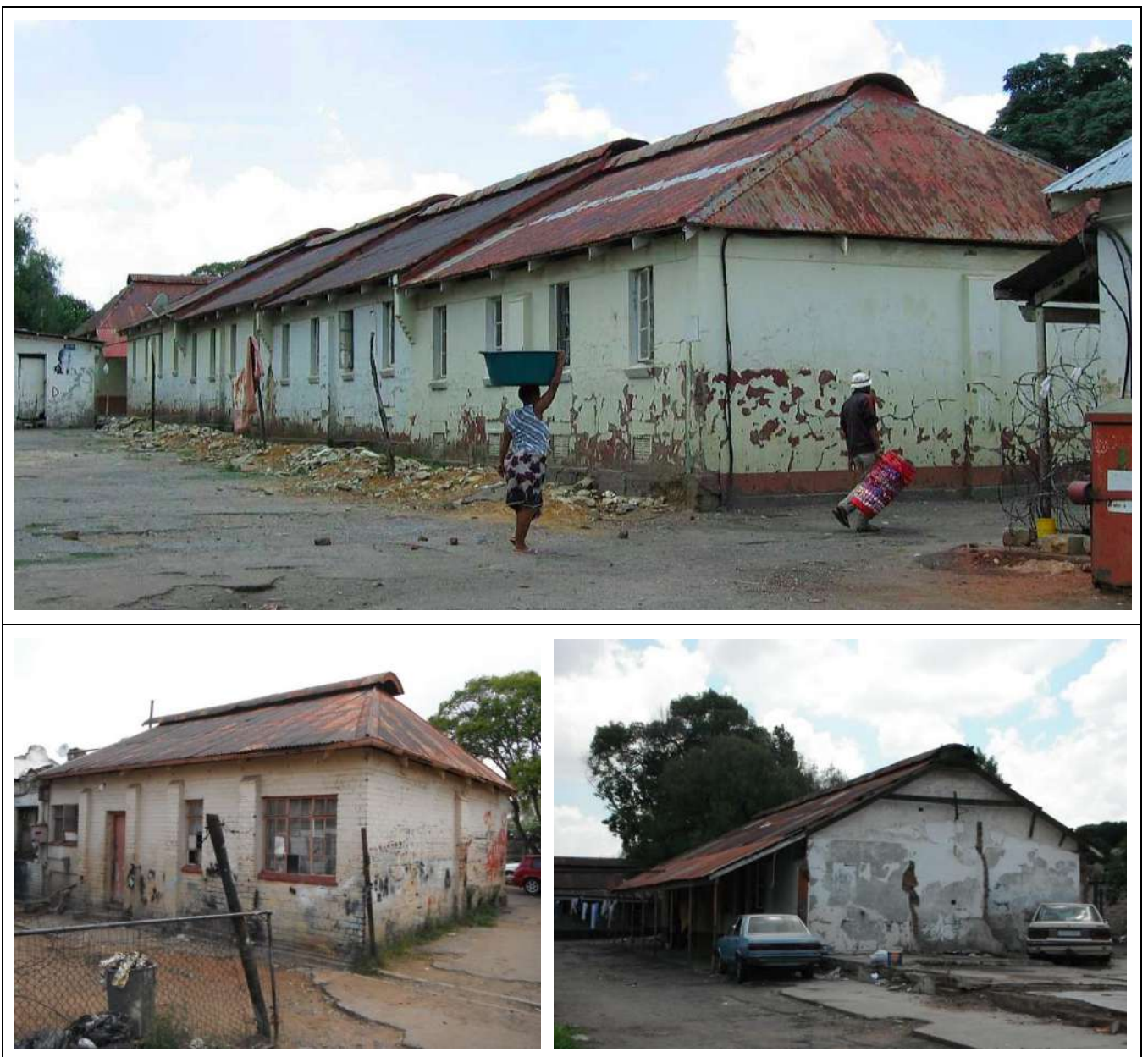
Figure 95 – General views of Building Type 50.
