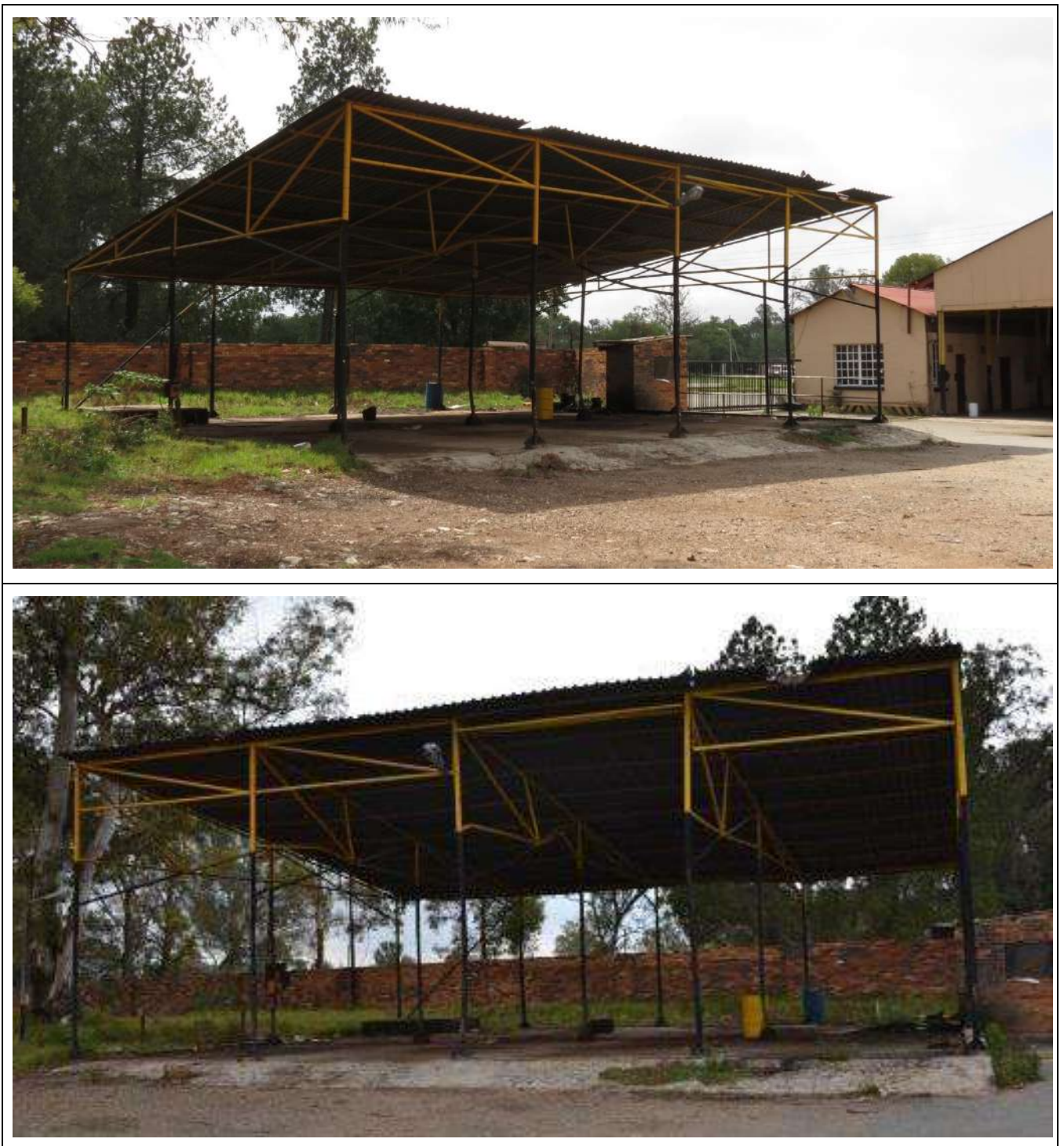
Figure 114 – General views of Building Type 73.
