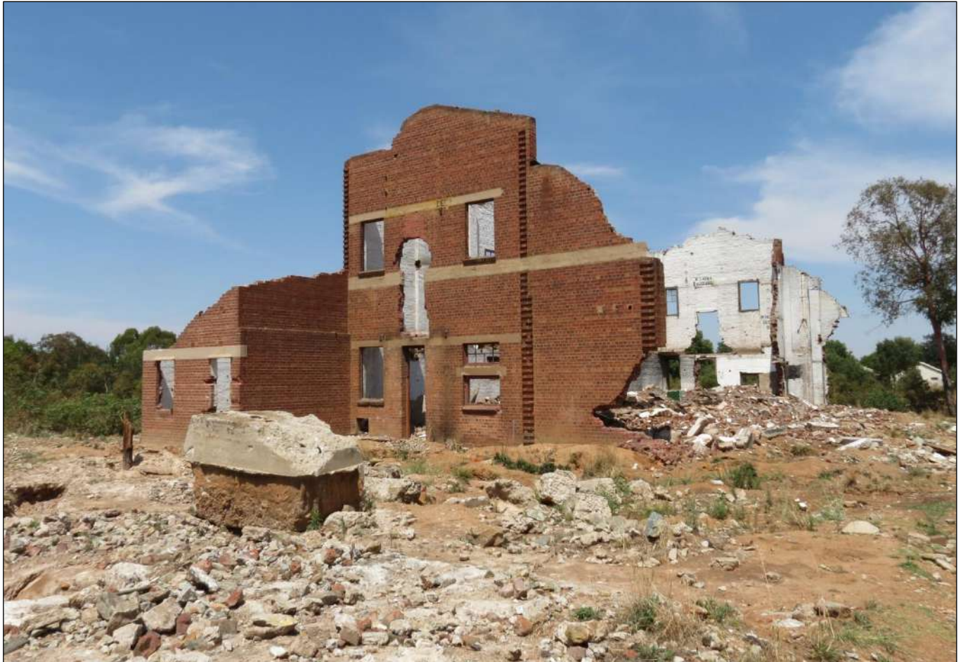
Figure 129 – General view of the electrical substation included in this report as Building Type 55. This photograph was taken during the site visit of Tuesday, 28 October 2014.
