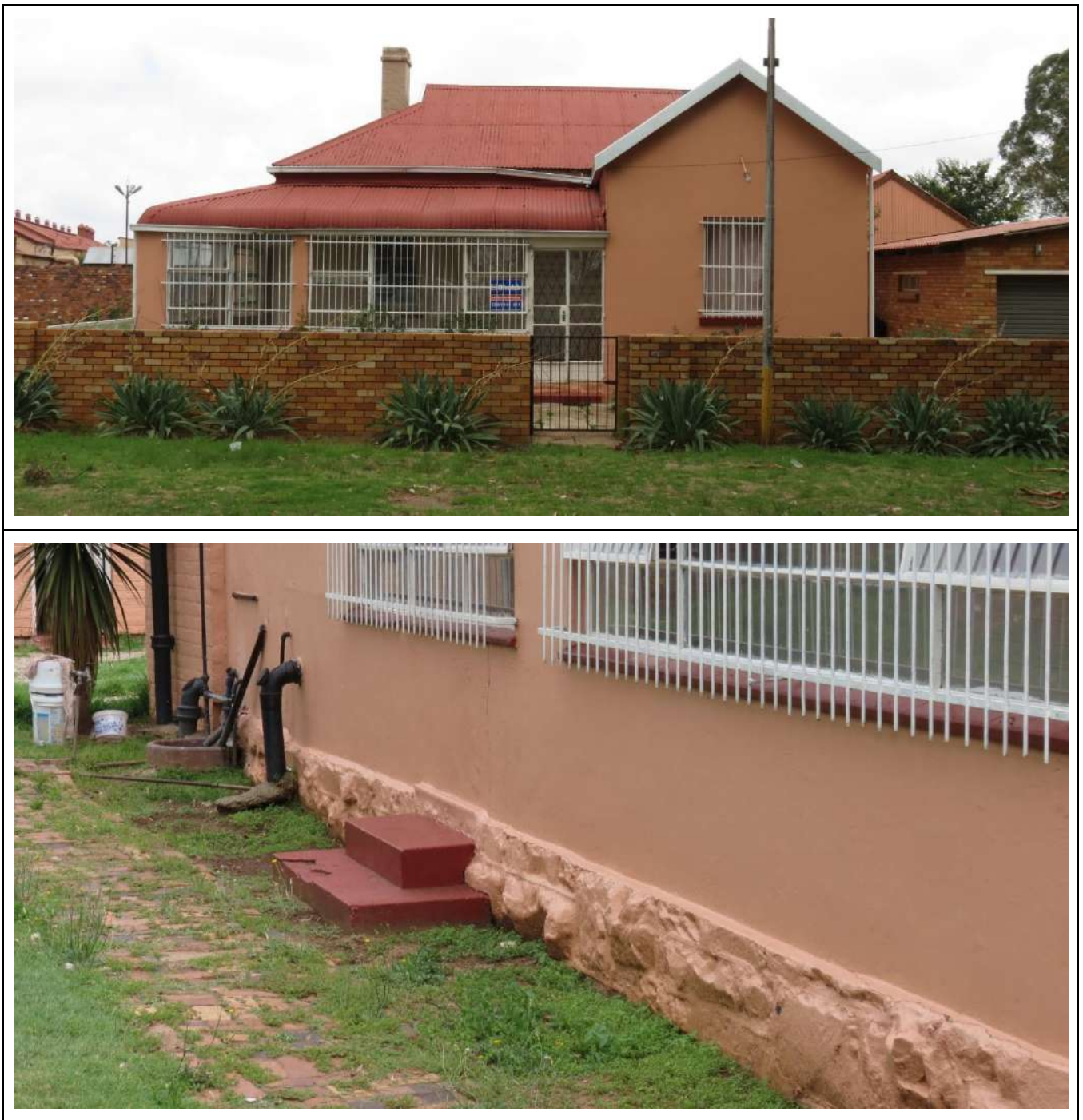
Figure 125 – General views of Building Type 84.
