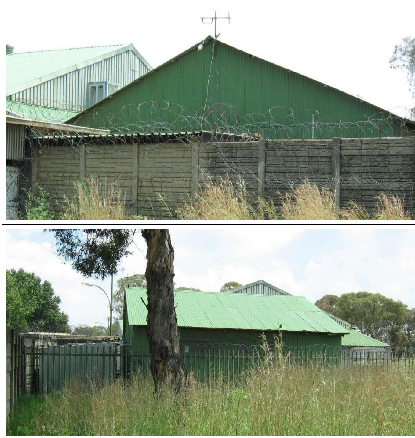
Figure 53 – General views of Building Type 16.
