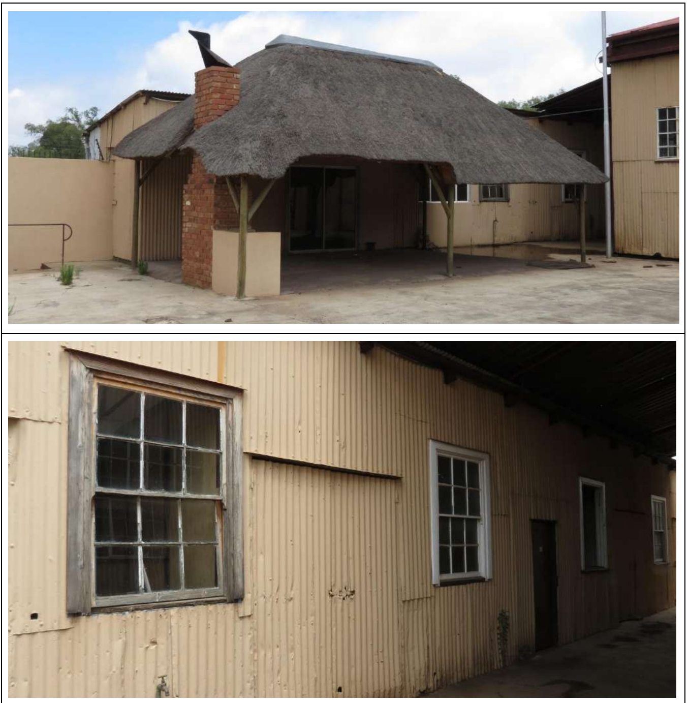
Figure 111 – General views of Building Type 70.
