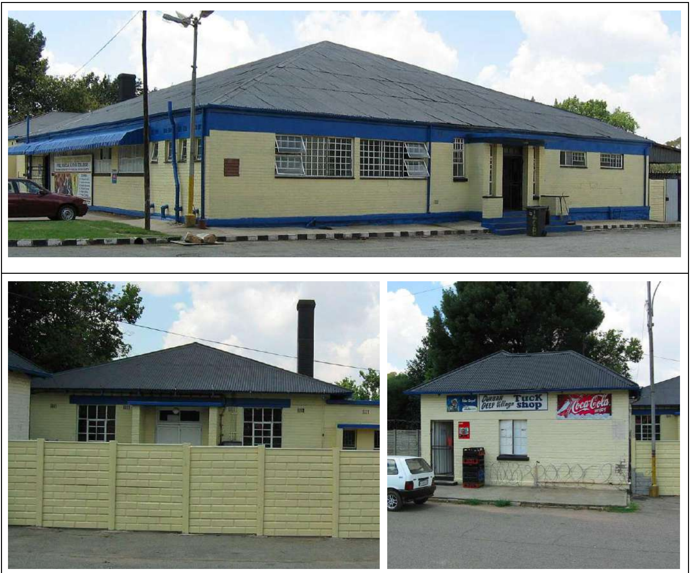
Figure 90 – General views of Building Type 46.
