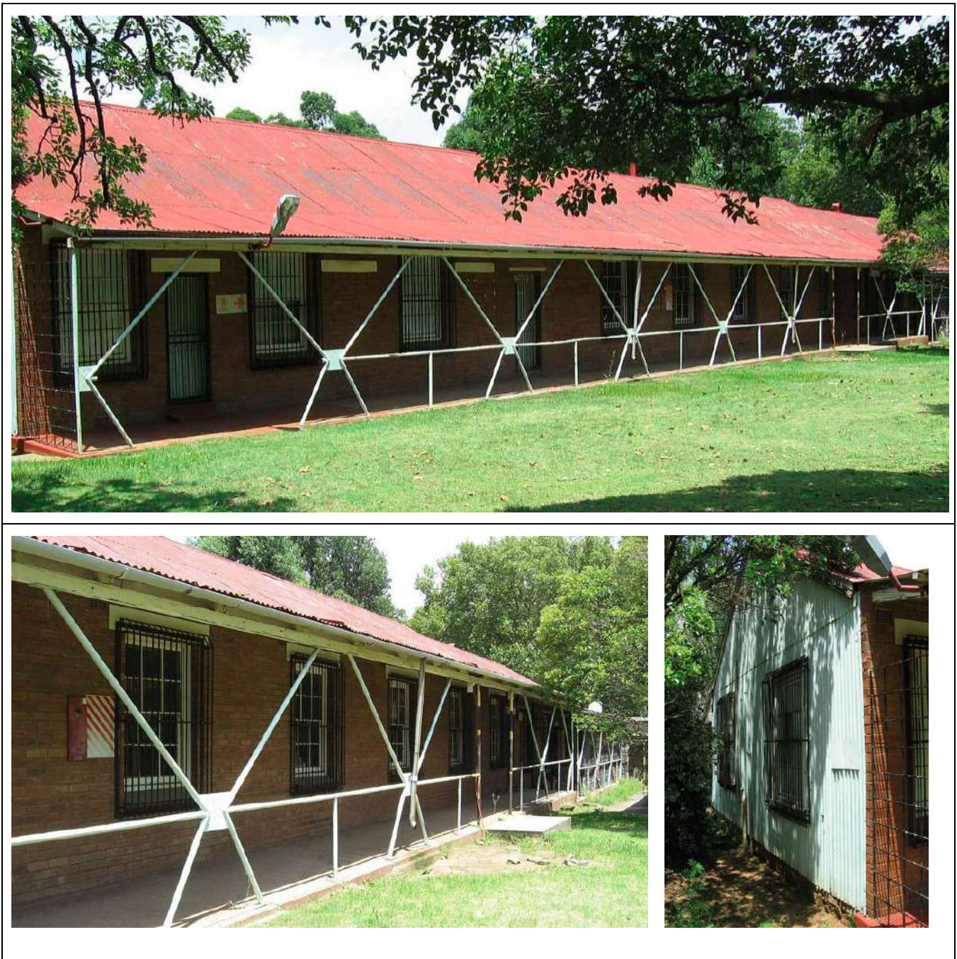
Figure 84 – General views of Building Type 40.
