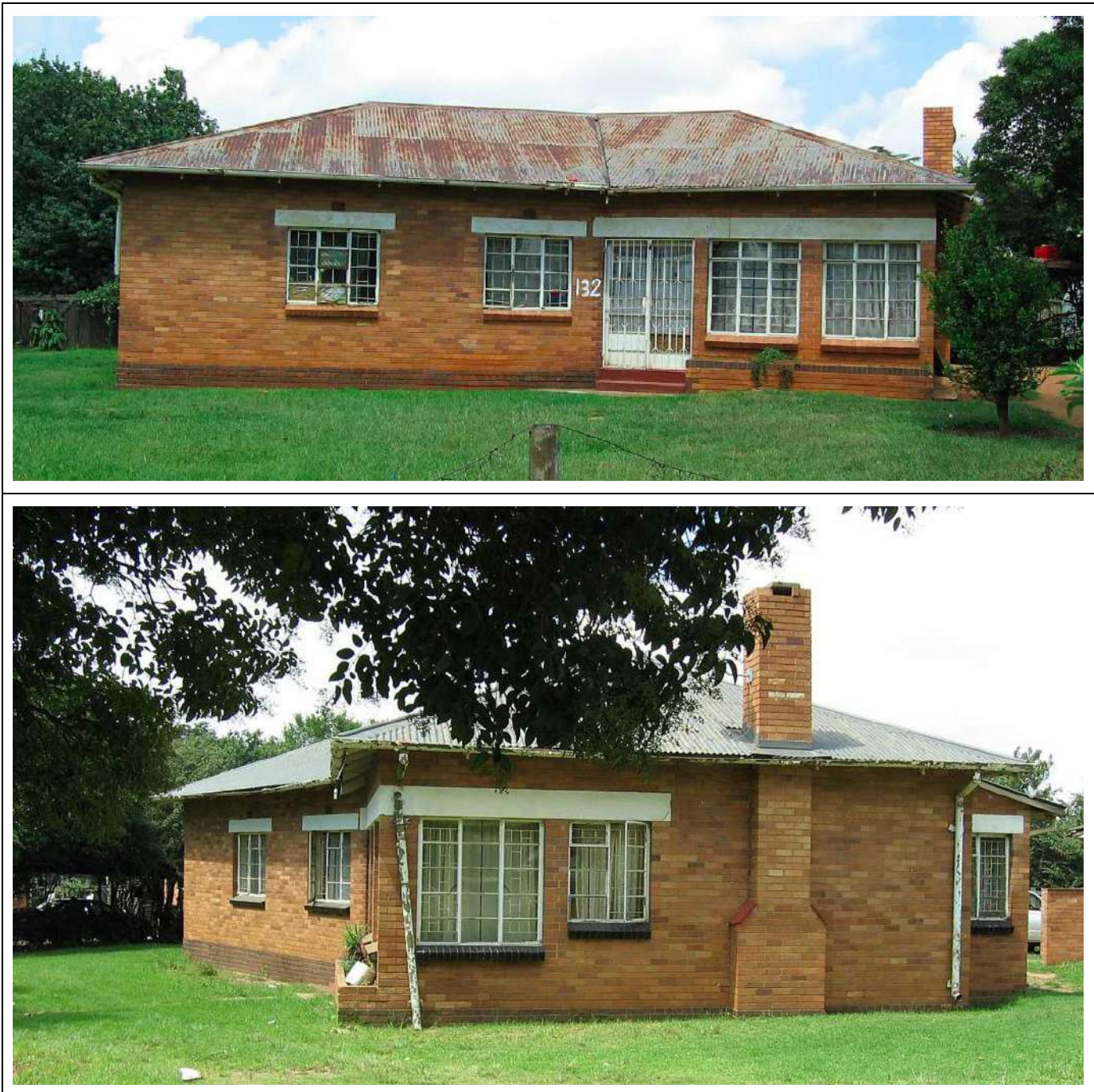
Figure 66 – General views of Building Type 25.
