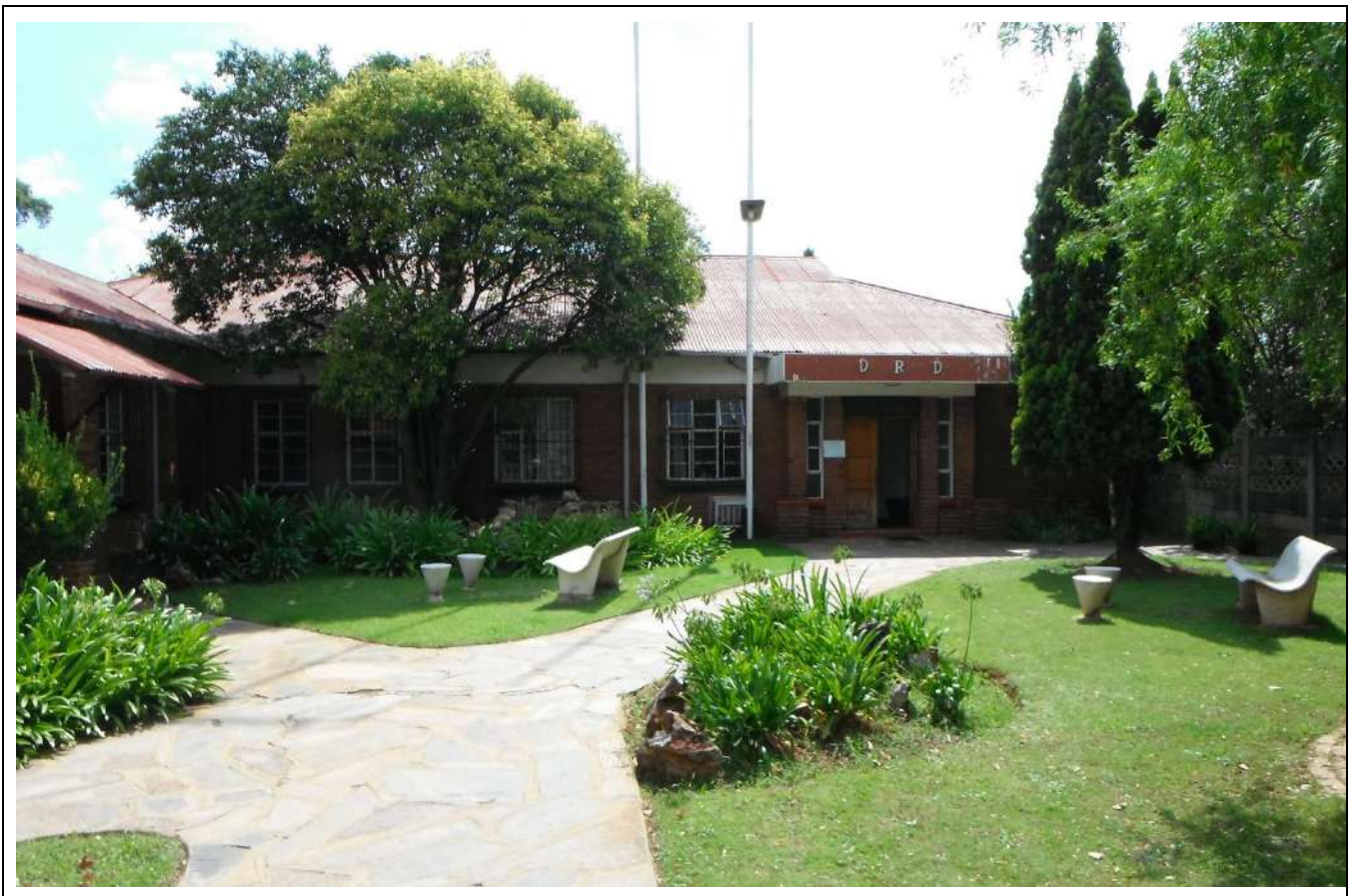
Figure 81 – General view of the front entrance of the old DRD office building at Building Type 38.
