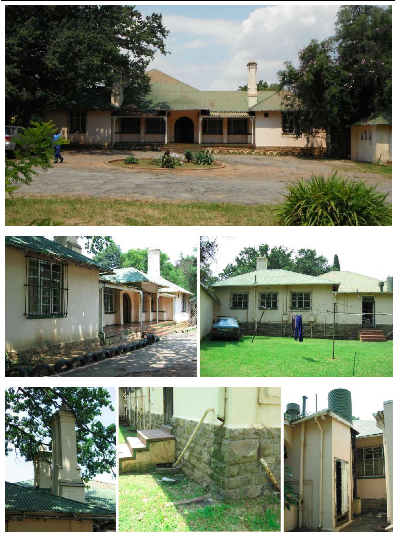
Figure 69 – General and detail views of Building Type 28.
