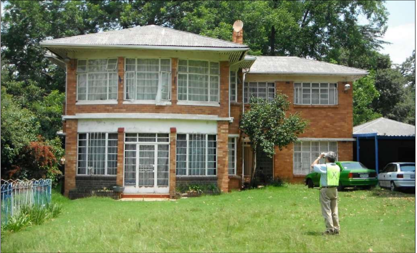
Figure 134 – General view of one of the examples of Building Type 17 as seen during the fieldwork of 2011.
