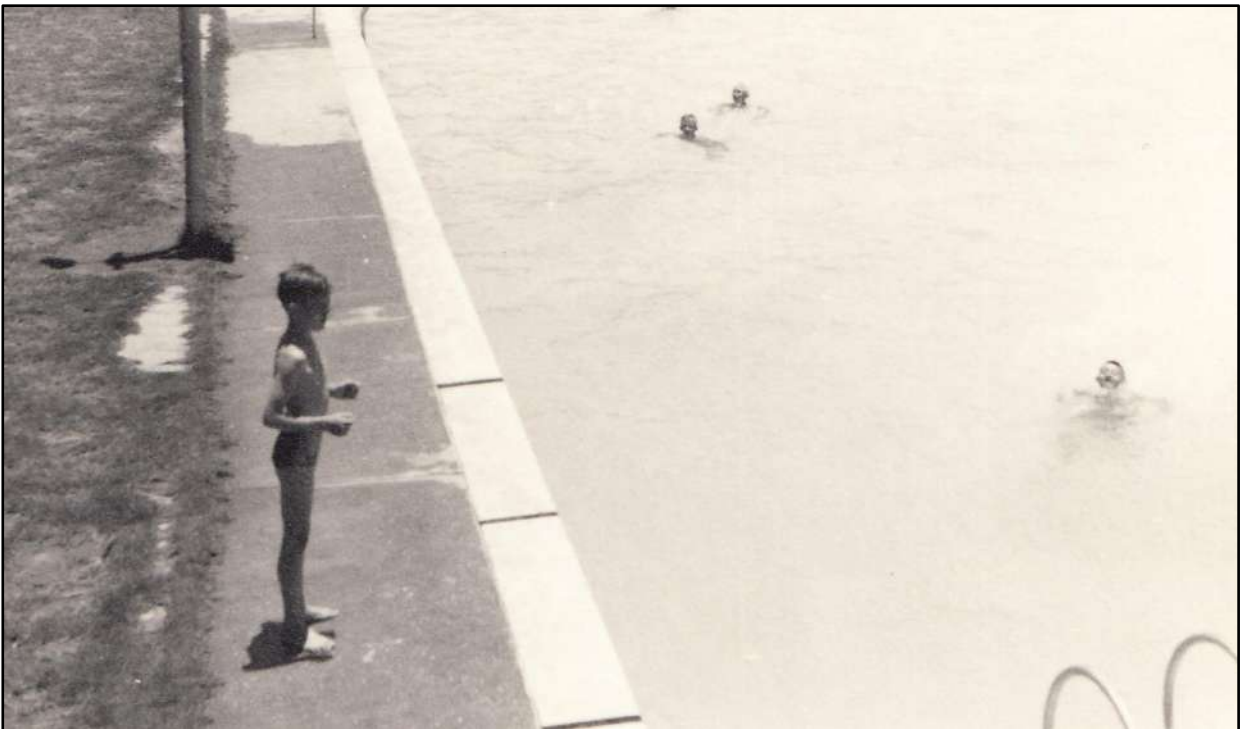
Figure 26 – Historic photograph of the staff village swimming pool. Obtained from the Barloworld Archives.
