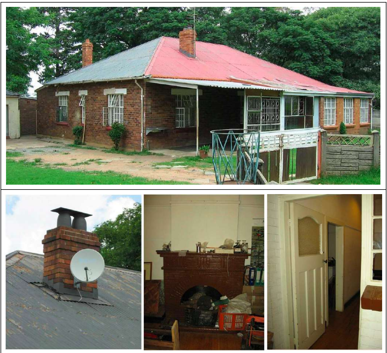
Figure 77 – General views of Building Type 34.
