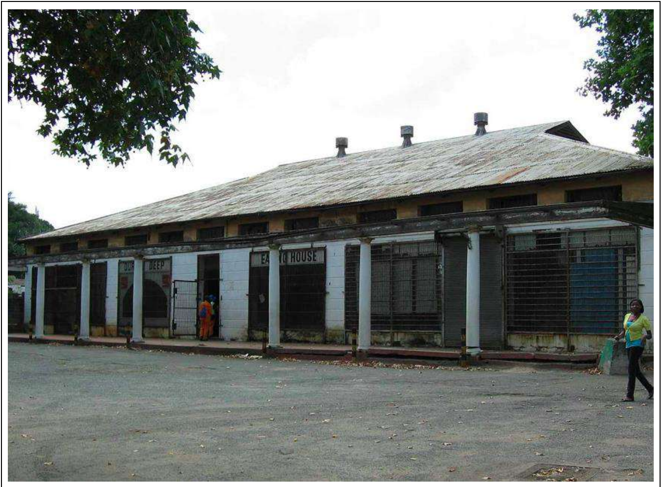
Figure 98 – General view of Building Type 53.
