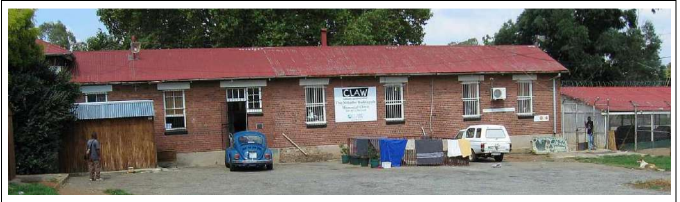
Figure 85 – General view of Building Type 41.
