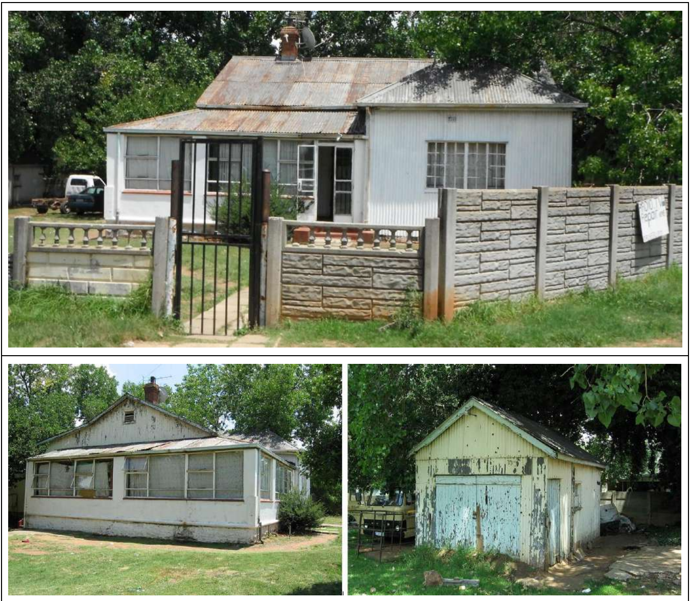
Figure 75 – General views of Building Type 32.
