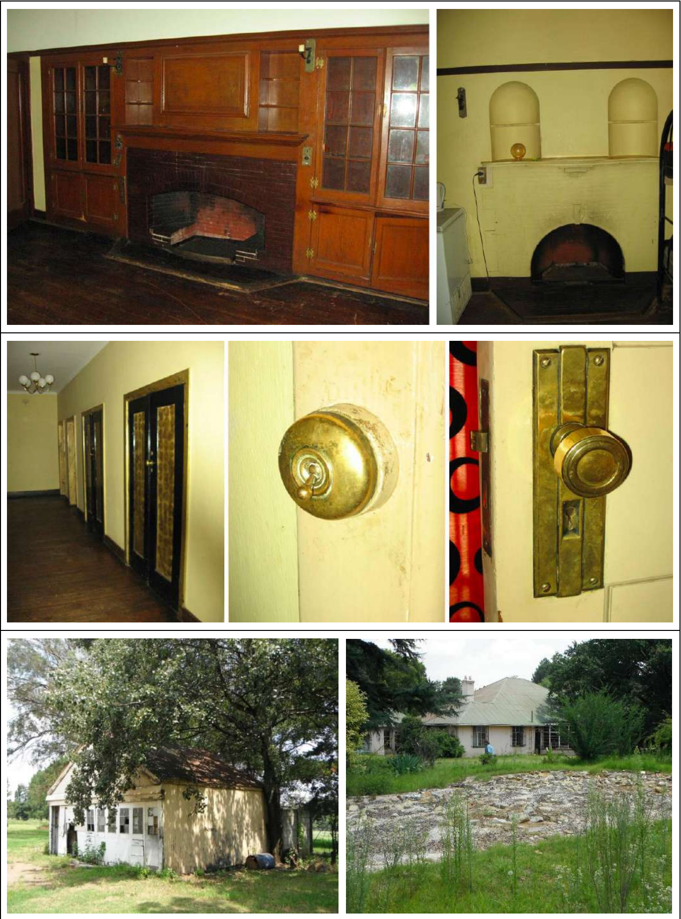
Figure 70 – Detail views of the interior of Building Type 28 as well as a general view of an associated garage.
