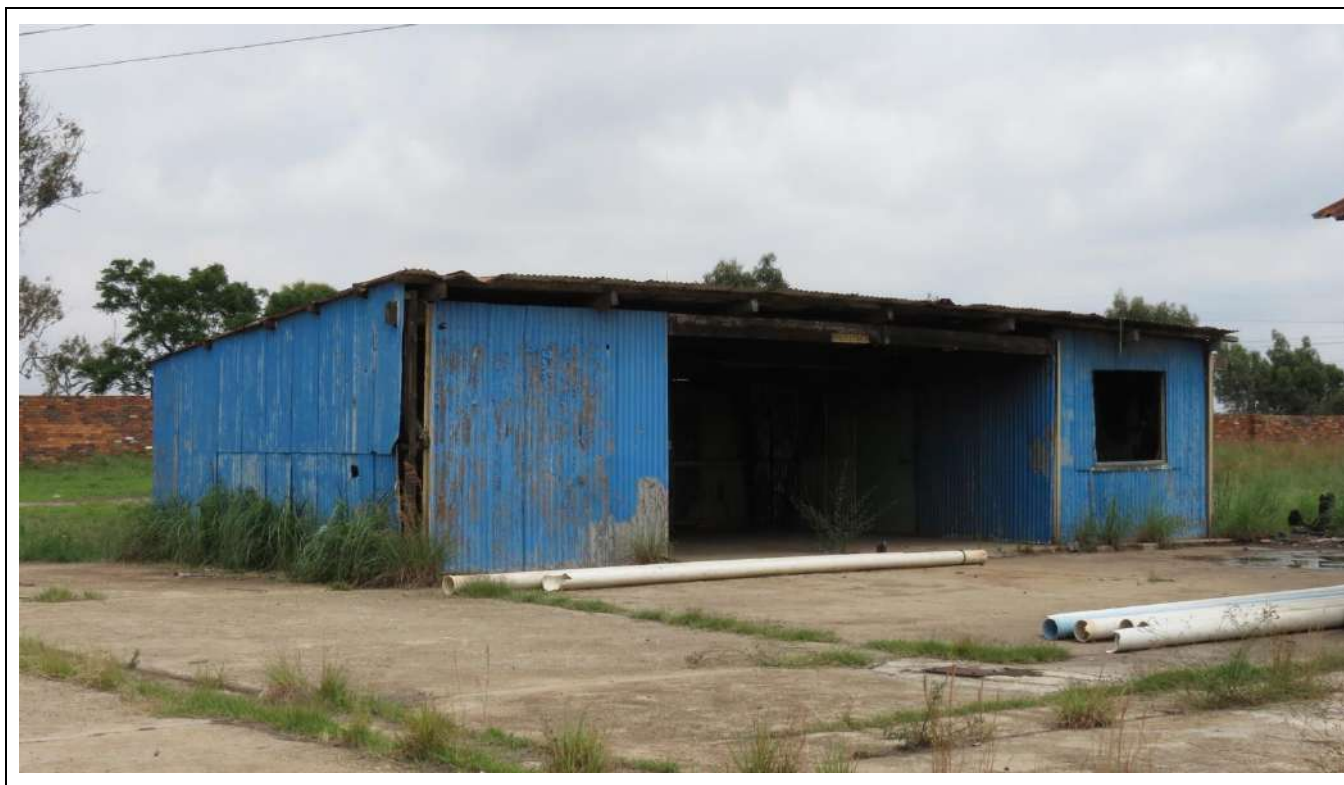
Figure 119 – General view of the front façade of Building Type 78.
