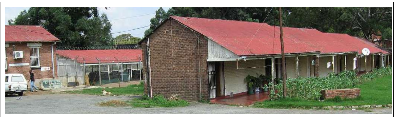
Figure 86 – General view of Building Type 42.
