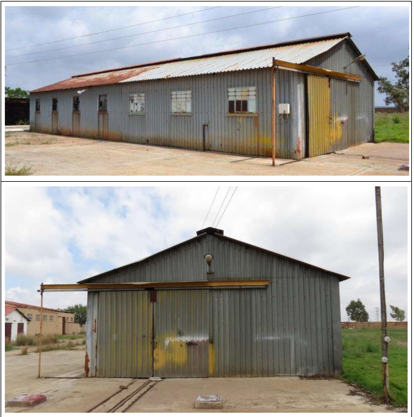
Figure 123 – General views of Building Type 82.
