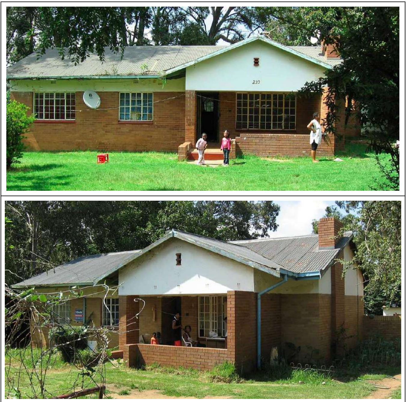
Figure 63 – General views of Building Type 22.
