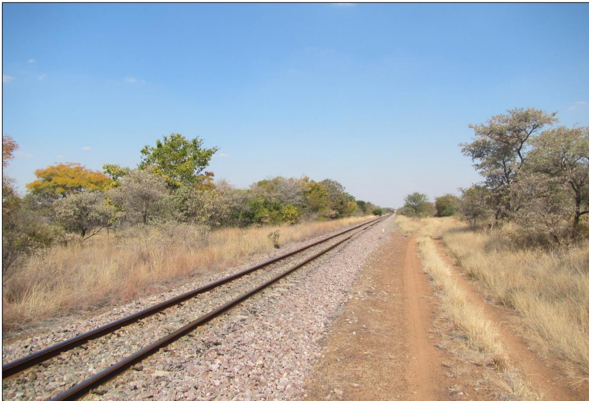
Figure 7 – A significant section of the central portion of the proposed pipeline will be constructed along the railway line between Thabazimbi and Lephalale. The development will be kept outside of the railway servitude.
