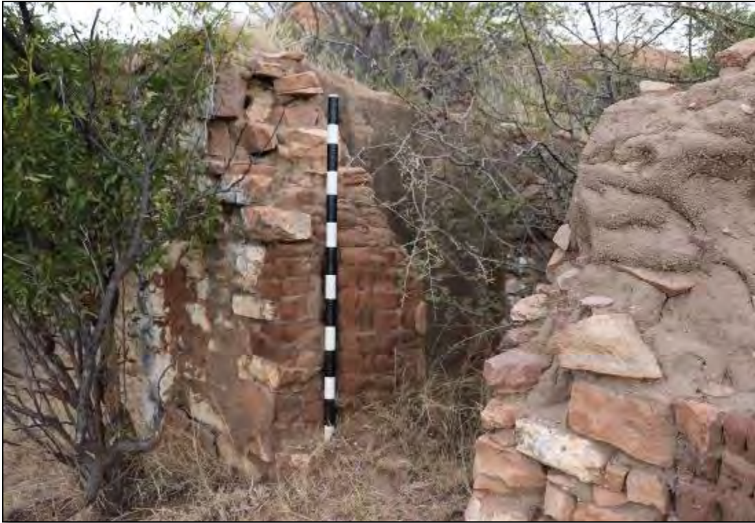
Figure 117 – This photograph of the front door shows the width of the walls as well as the use of both stone and clay bricks in the construction of the structure. Scale in 10cm increments.
