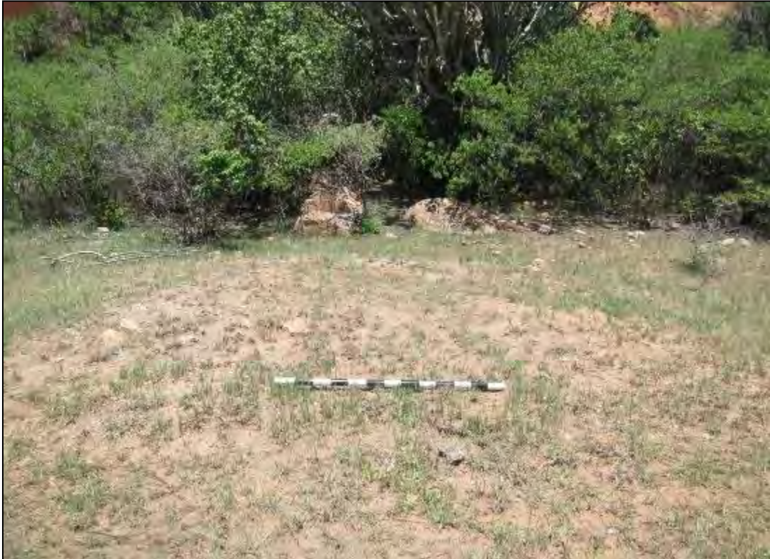
Figure 142 – View of the foundation of the mud rondavel. Scale is in 10cm increments.
