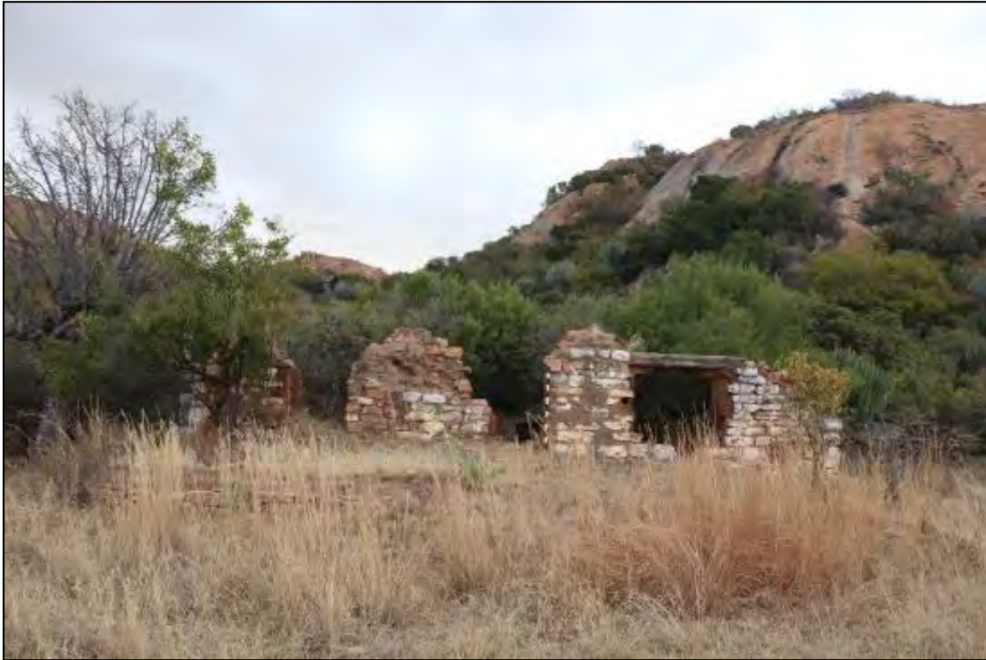
Figure 115 – General view of the front façade of the historic farmstead as seen from the east. Scale in 10cm increments.
