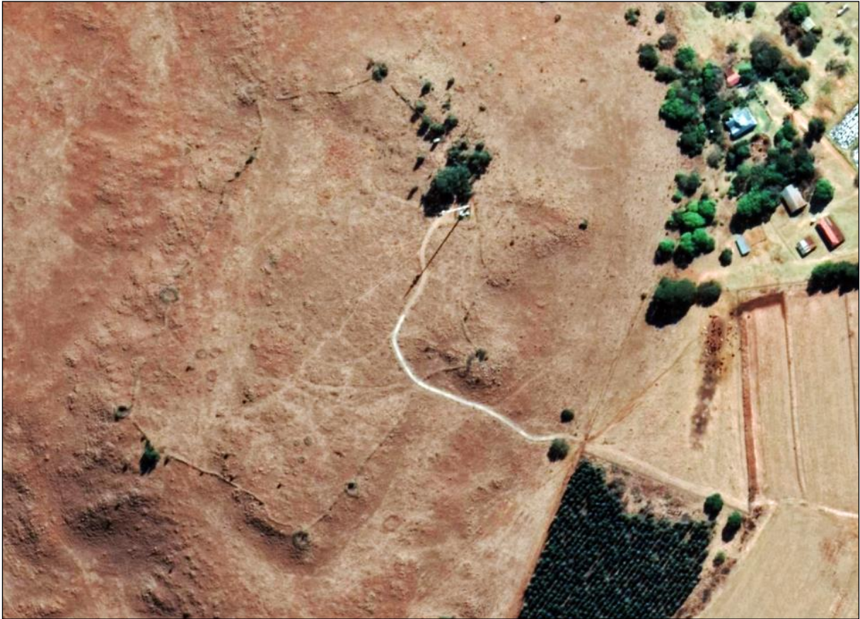
Figure 12 – Google Earth image showing the Amsterdam farmstead on the right with the stonewalled British fortifications visible on the left. These fortifications formed part of the blockhouse line between Wakkerstroom and Piet Retief during the South African War (1899-1902).
