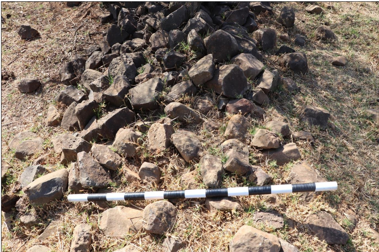
Figure 36 – Cross-section view of a section of walling from the livestock enclosure at site KCP 5. The scale is in 10cm increments.
