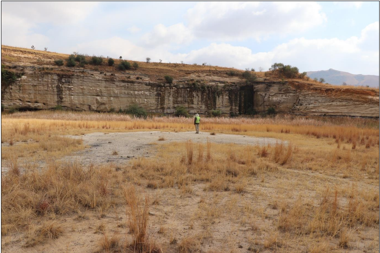
Figure 5 – General view of a section of the proposed Balgarthen Adit. As can be seen from this image, this section of the study area was extensively disturbed by previous mining activities.
