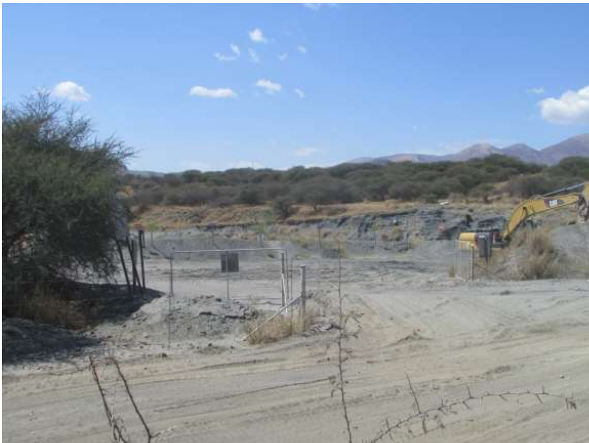
Figure 3: A view of ongoing Mining operations in the TWF3 area.
