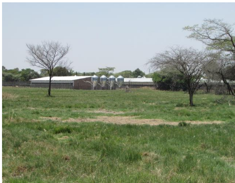
Figure 2: View of the existing Piggery adjacent to the Site 1 location.
