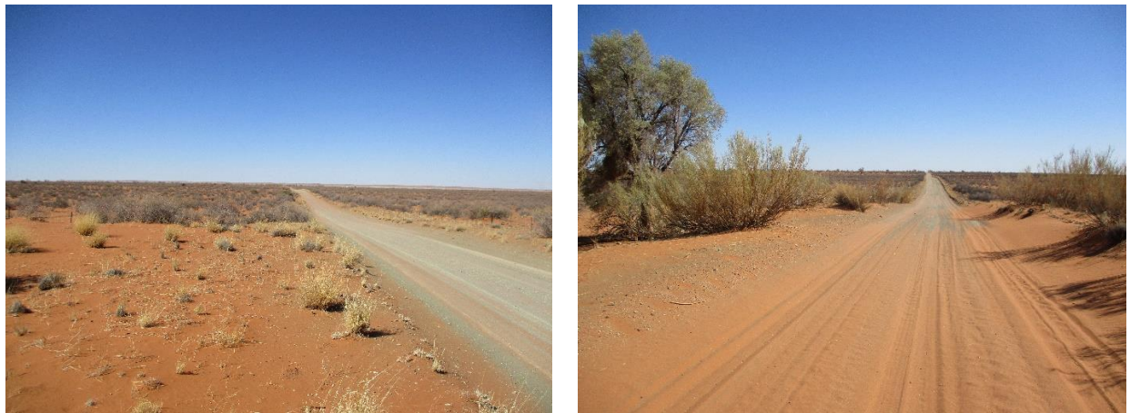
Figure 3. Panoramic view of the service road, Swartkopdam alignment.
