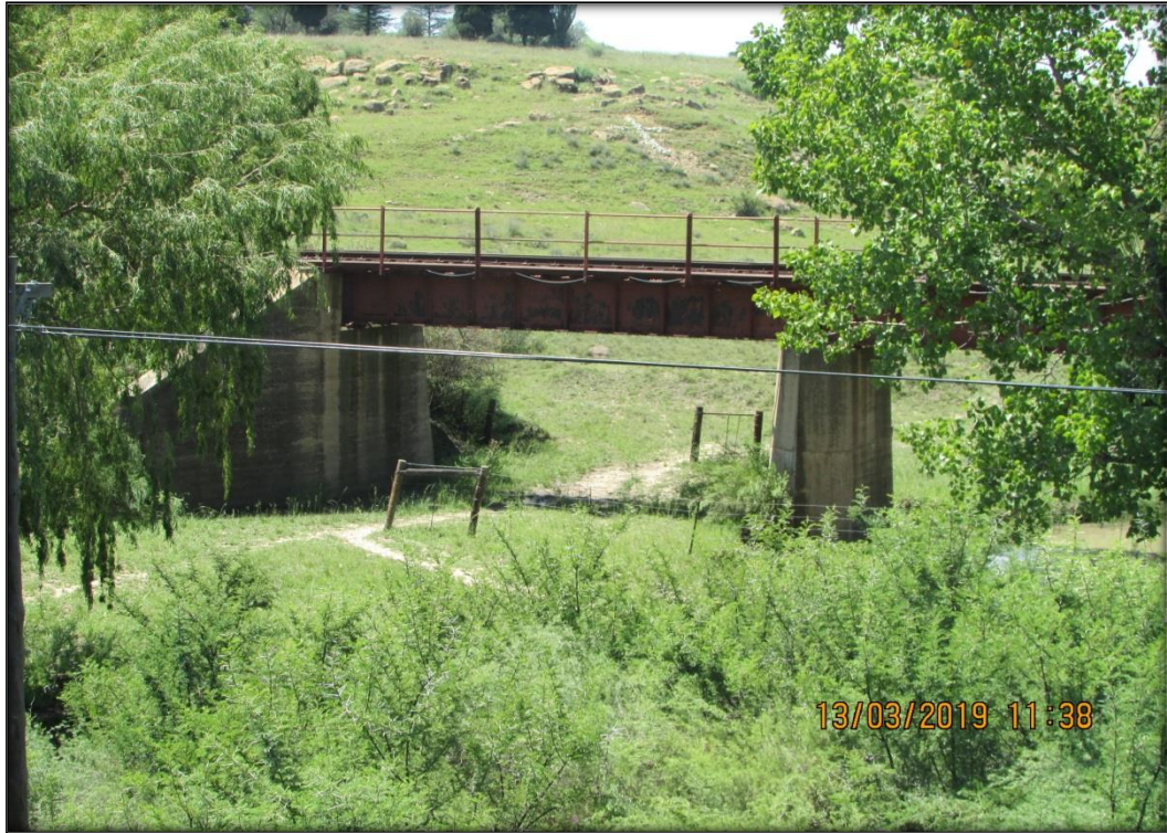
Figure 27: Site 2 Railway Bridge.
