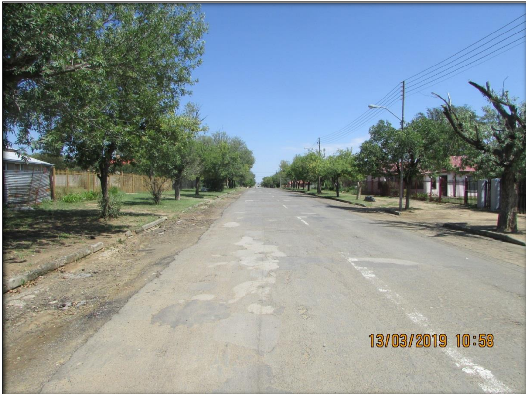
Figure 13: A section of the pipeline route follows an existing road through Lindley.
