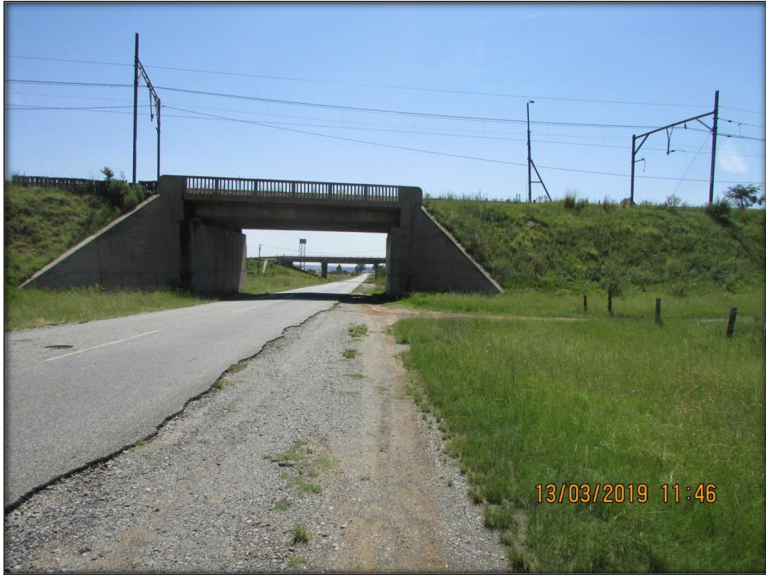
Figure 22: View of another recent bridge crossing near Arlington.
