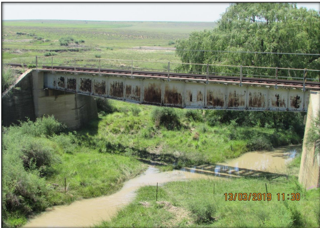
Figure 26: Site 1 Railway Bridge.
