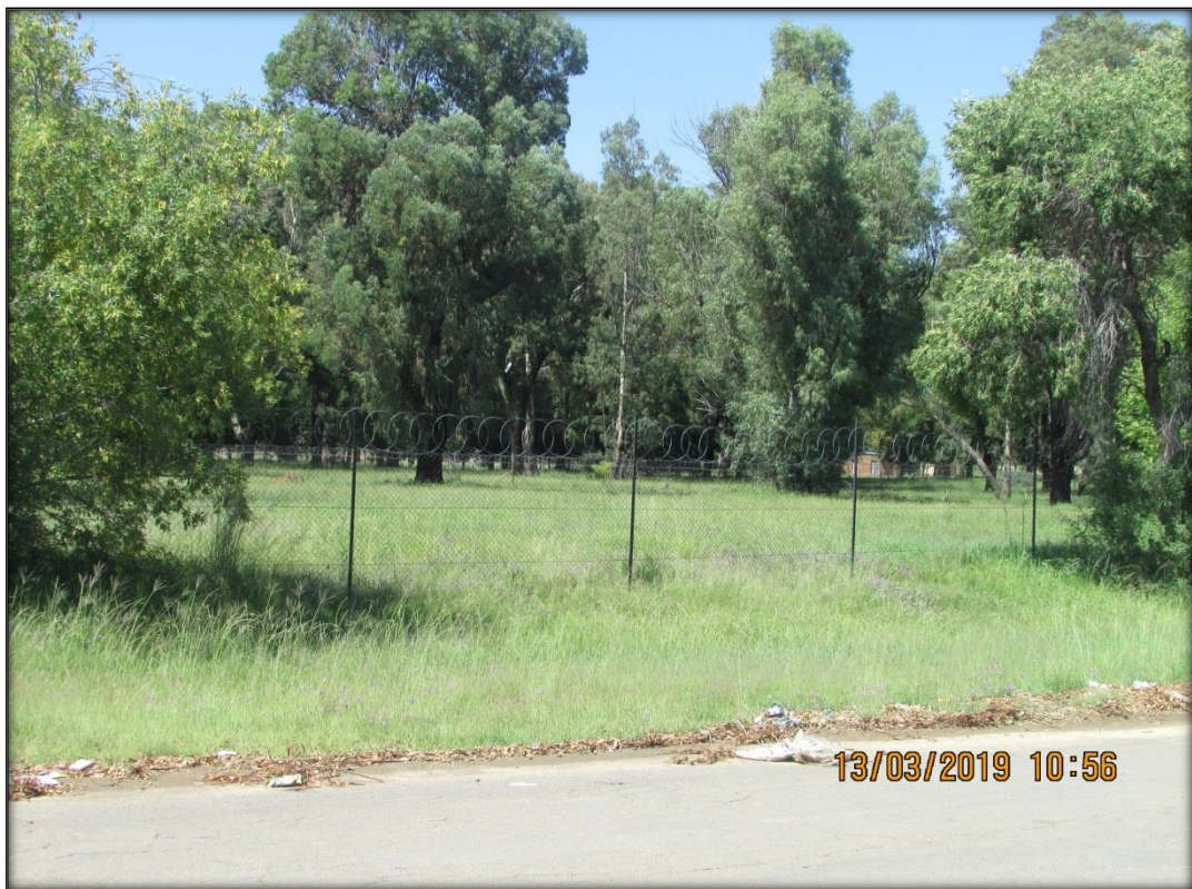
Figure 12: A section of the route in Lindley close to the WTP.
