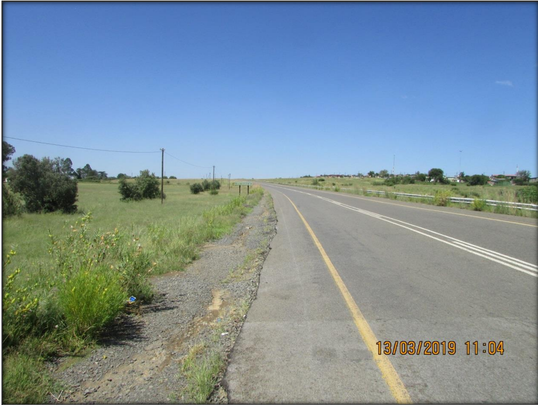
Figure 15: View down the R707 from Lindley towards Arlington. The pipeline will follow the existing servitude and road reserve.
