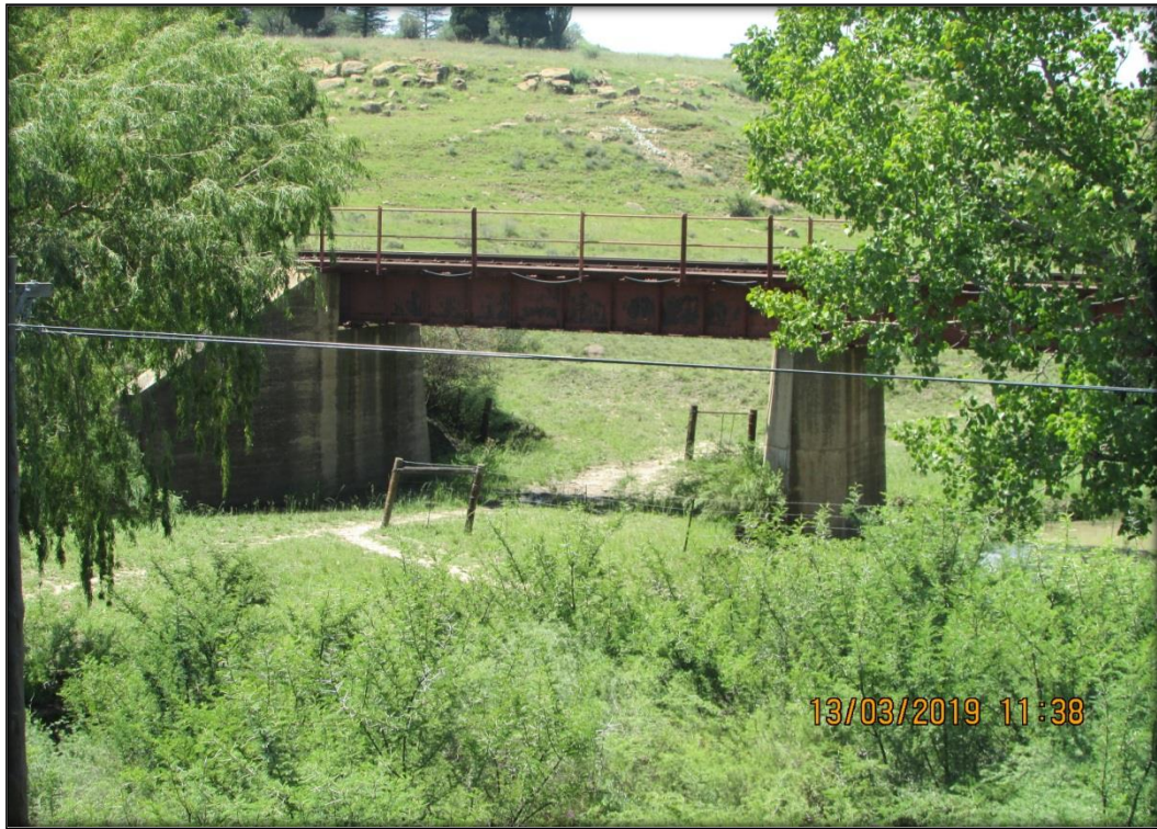
Figure 27: Site 2 Railway Bridge.
