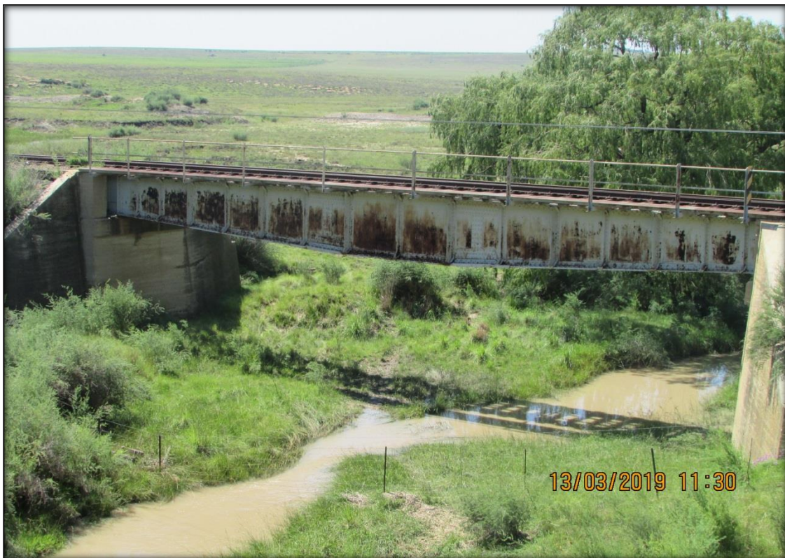
Figure 26: Site 1 Railway Bridge.
