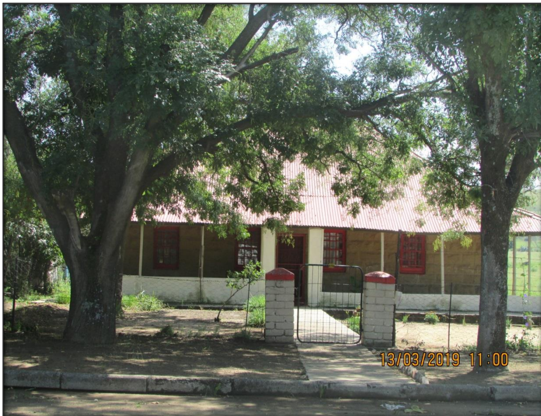
Figure 14: Old (historic) house in Lindley adjacent to a section of the pipeline. The proposed pipeline route will not impact on it.
