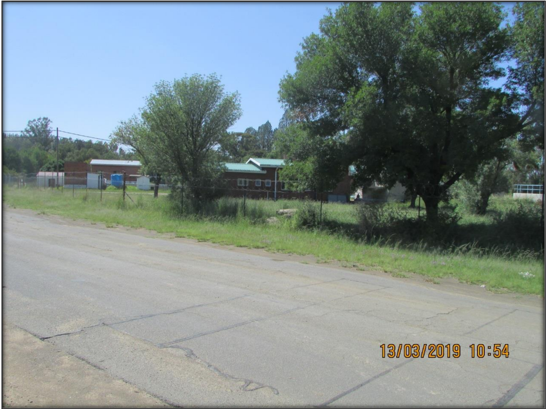
Figure 11: Start of pipeline route in Lindley at the Water Treatment Plant.
