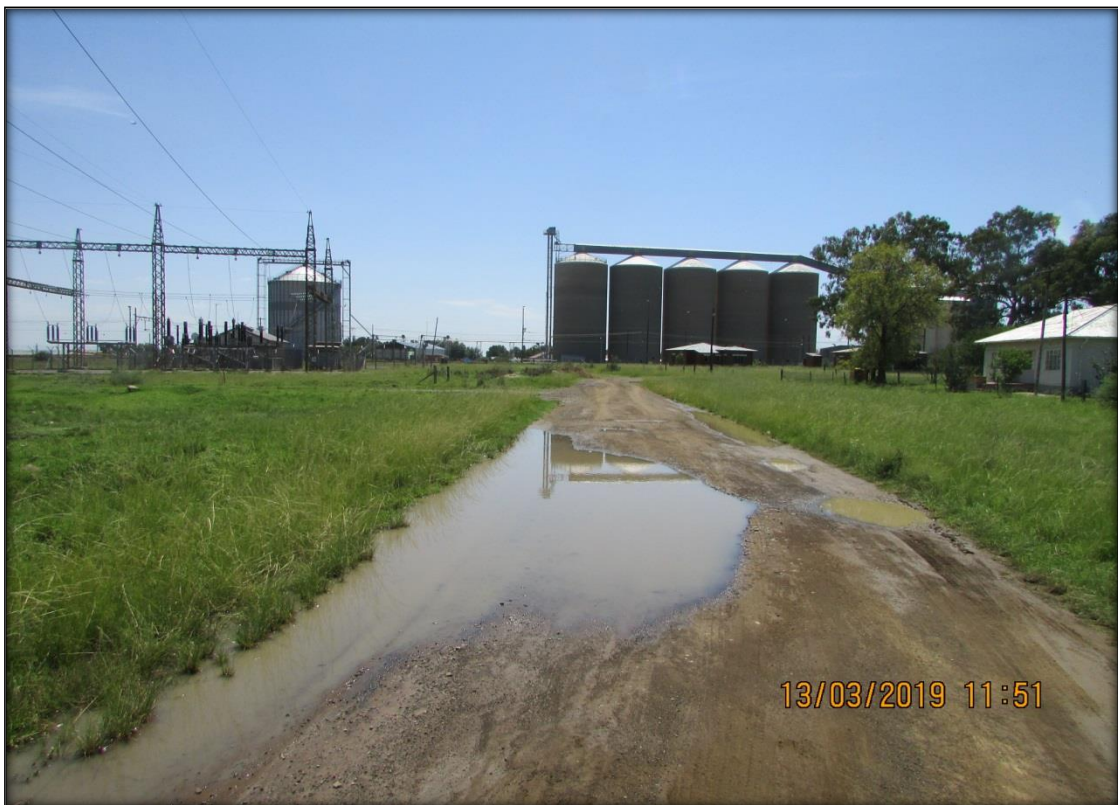
Figure 23: A view of a section of the pipeline route into Arlington.
