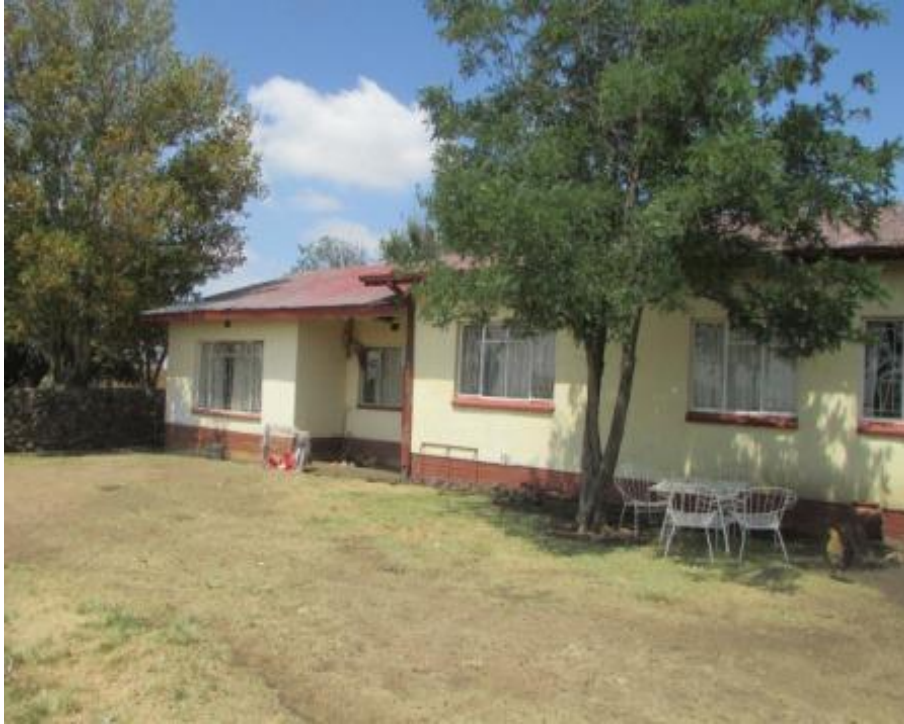
Figure 7: Partial view of the homestead on Merino. The homestead and related buildings are younger than 60 years of age & will be utilized as part of the farm management offices and for storage purposes.
