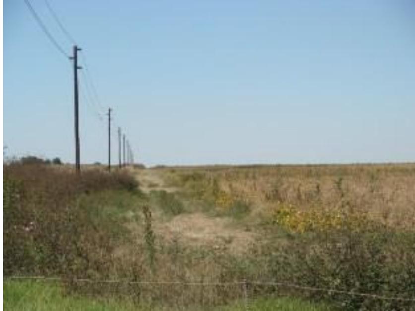
Figure 9: View on section of Option 2 route running on an existing servitude. Note the ploughed fields.
