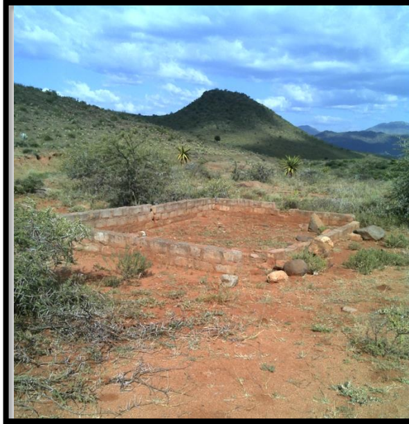
Figure 7: The abandoned residential infrastructure at the edge of the western dome.
