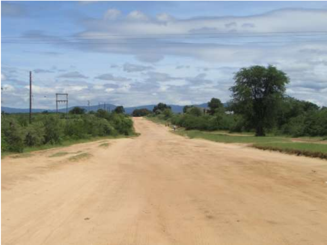
Figure 10: Another view down the line route towards Matsephane.
