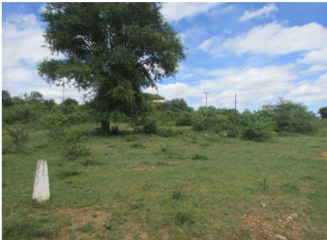
Figure 15: A view of the line route running up to the Matsephane Water Reservoir.
