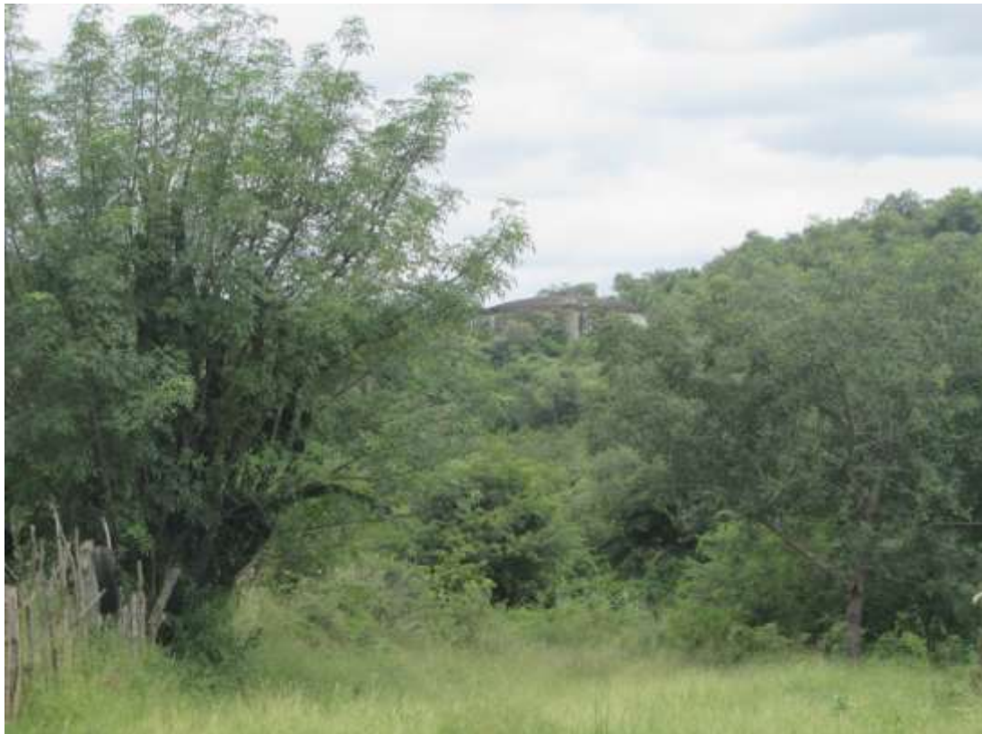
Figure 23: View of the line route up to the Babanana Water Reservoir.
