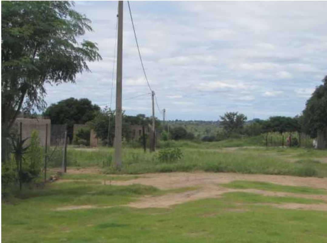
Figure 22: Section of the line route close to Babanana Water Reservoir.
