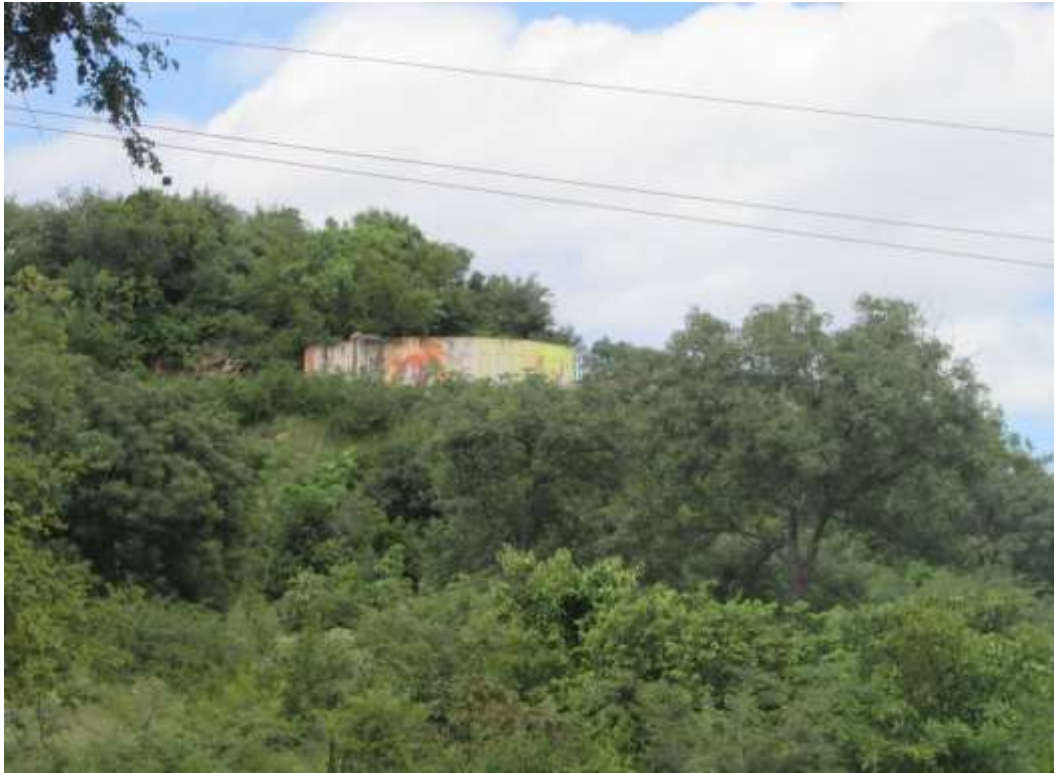
Figure 16: View of Matsephane Water Reservoir.
