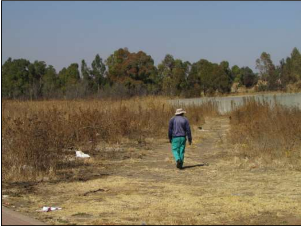
Figure 19: The sewer line route follows existing servitudes in most sections.
