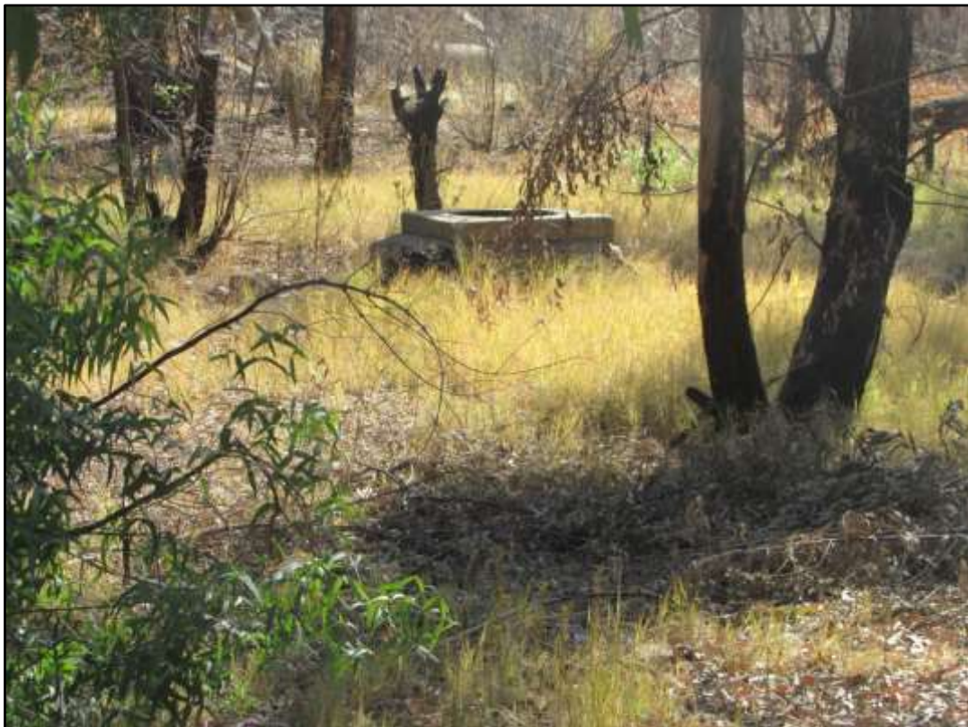
Figure 22: An old sewer connection point in the area seen in Figure 21.
