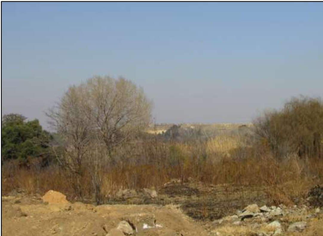
Figure 14: Another section of the Comet Sewer Line route.
