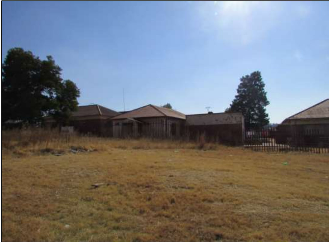
Figure 15: Part of the line route will run past these old railway-type houses but will not impact them (close to Reiger Park).
