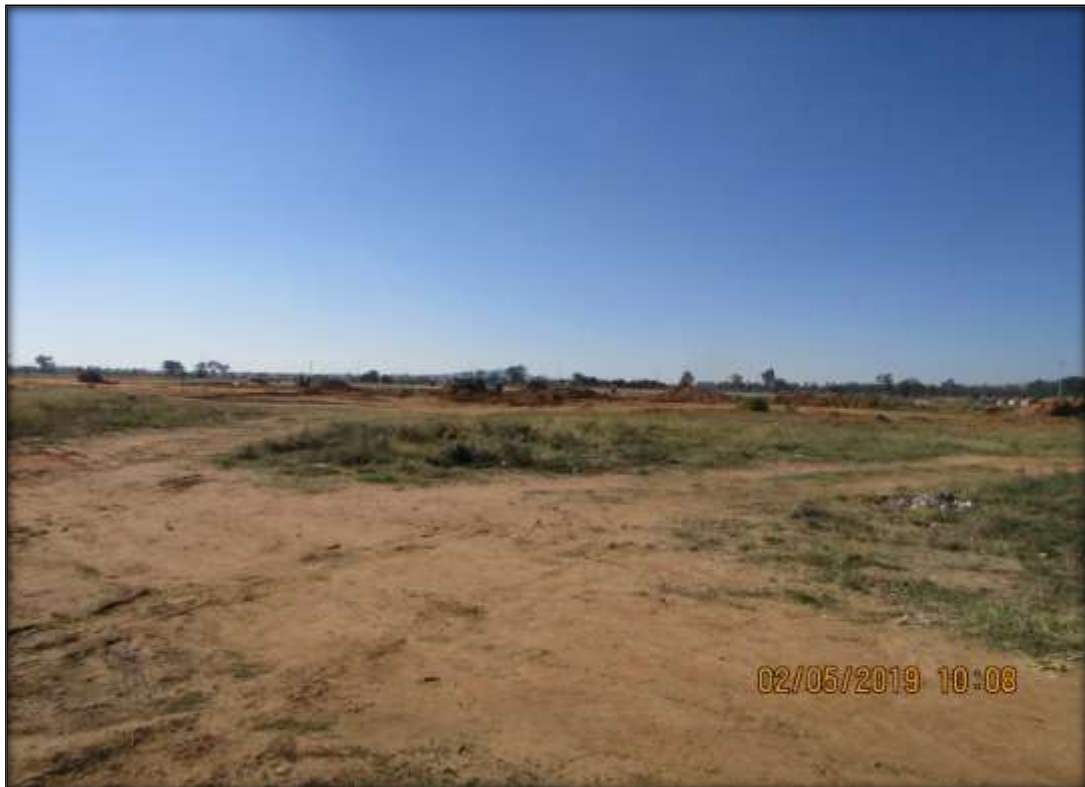
Figure 5: A view of current & ongoing development work in the area.
