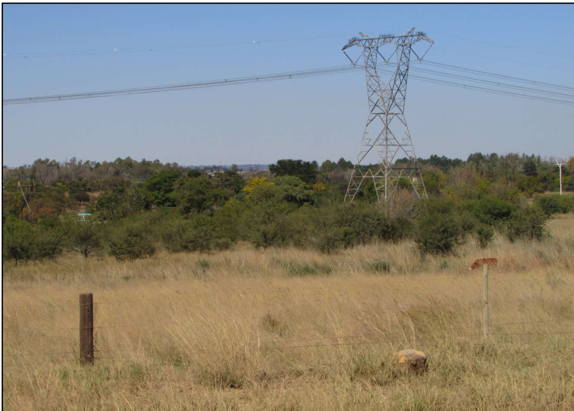
Figure 25: View of section close to A98.
