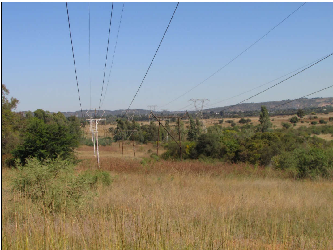
Figure 27: A general view of the area towards A115.
