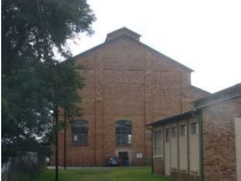
Figure 19: Main building next to headgear.
