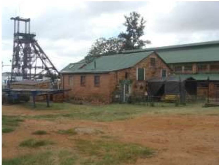
Figure 8: A view of one of the warehouses/businesses with the old No.4 Shaft headgear visible.
