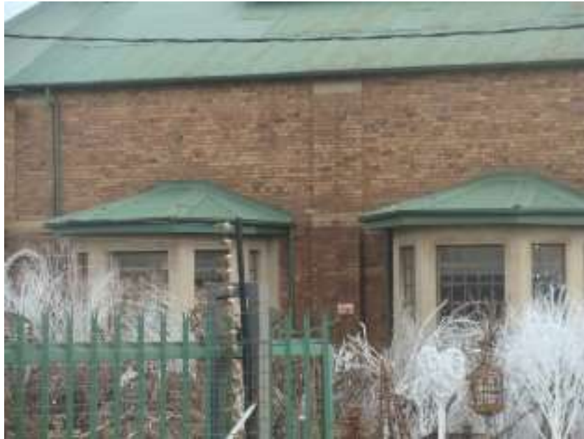
Figure 23: View of Main warehouse with recent additions visible.
