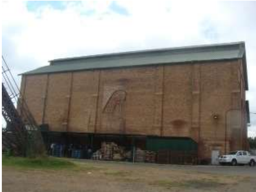
Figure 21: Another view of the same building.
