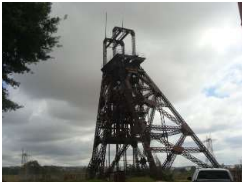
Figure 12: Old No.4 Shaft Headgear.
