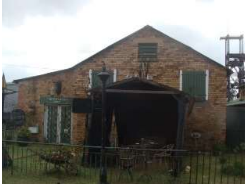
Figure 17: Another structure on the property.
