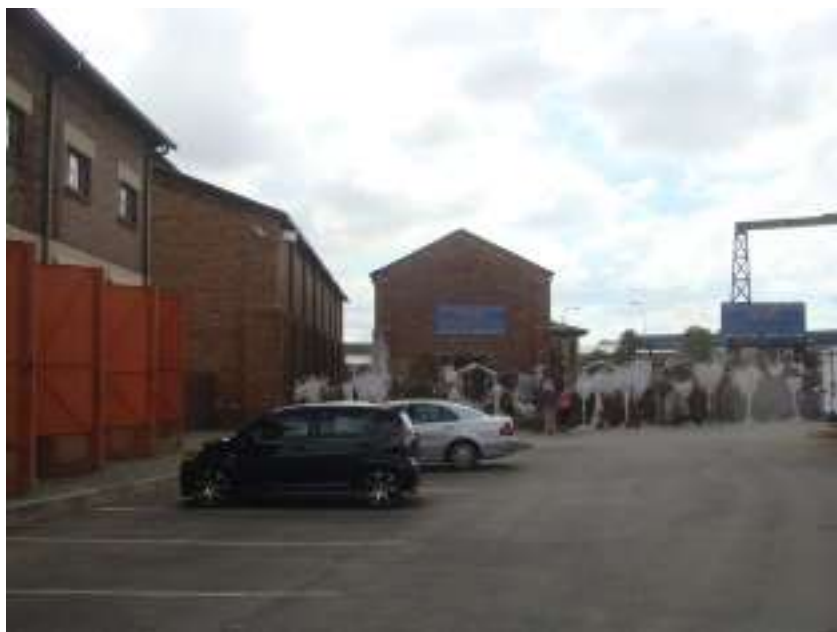
Figure 6: Commercial businesses are located in some of the buildings.
