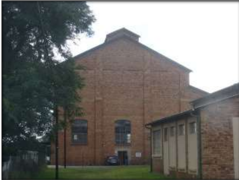
Fig.19: Main building next to headgear (2014).
