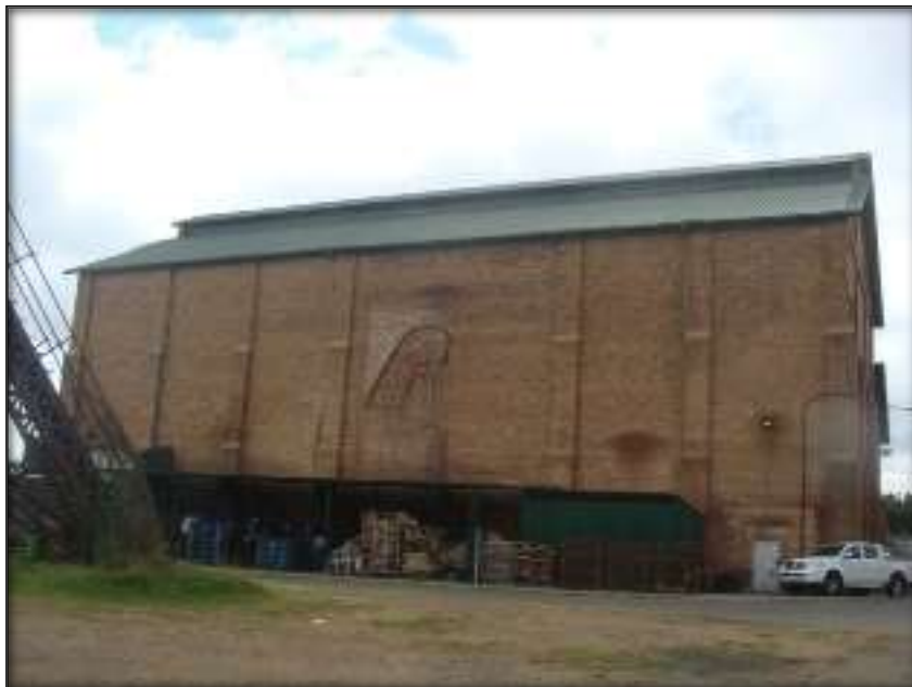
Fig.20: Another view of the same building in 2014.
