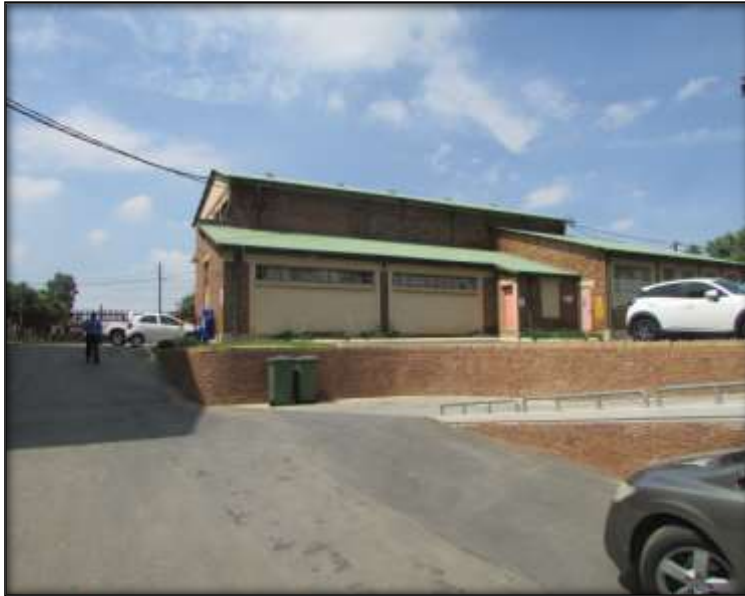
Fig.8: Another view of one of the warehouses (2019).
