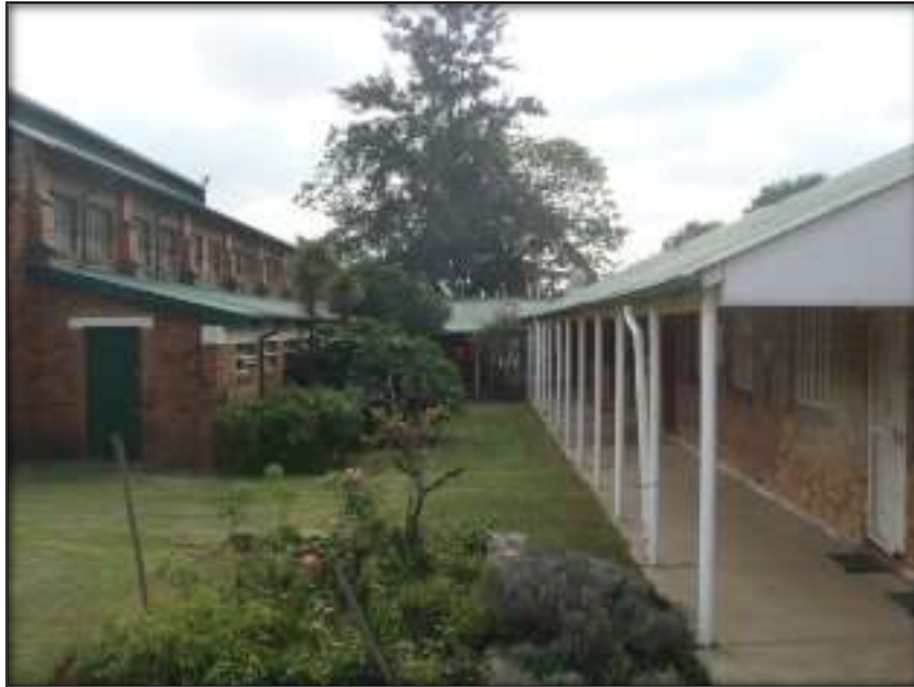
Fig.17: More office buildings and warehouse section (2014).
