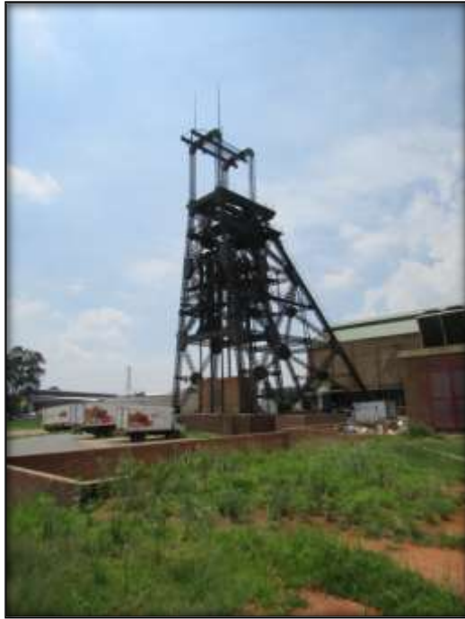
Fig.26: Another view of the structure in 2019.
