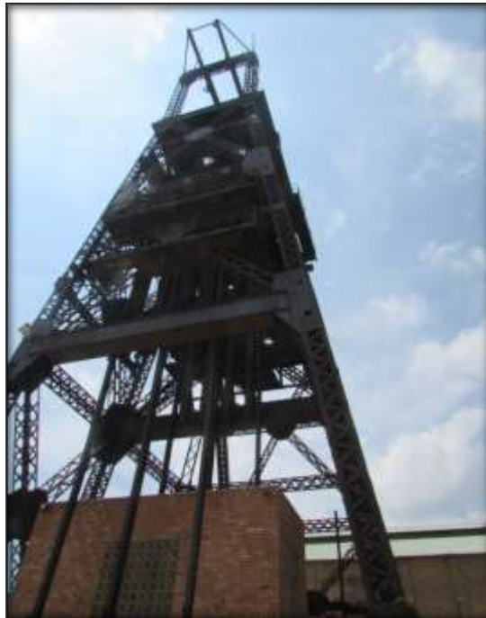
Fig.27: Closer view of part of the structure
