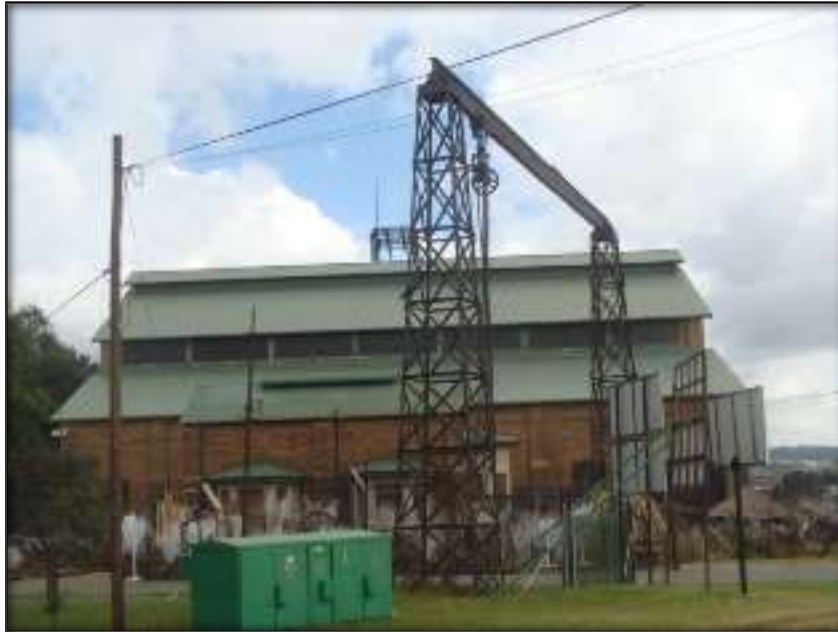
Fig.21: View of entrance feature taken in 2014. This structure was erected by the current tenant and does not form part of the historic fabric of the site as it was brought in from another location to the site.
