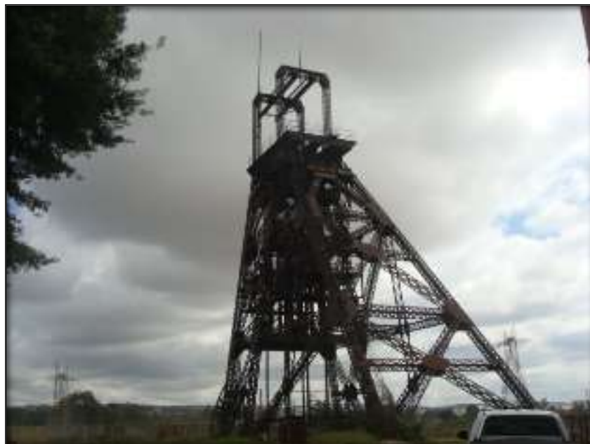
Fig.14: Old No.4 Shaft Headgear during 2014.
