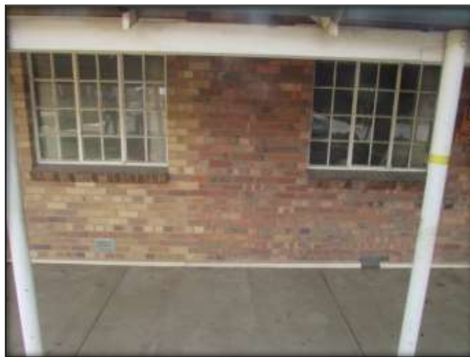
Fig.31: View of outside walling of Office Block. Two different bricks can be seen. This probably indicates changes & additions to the original structure.
