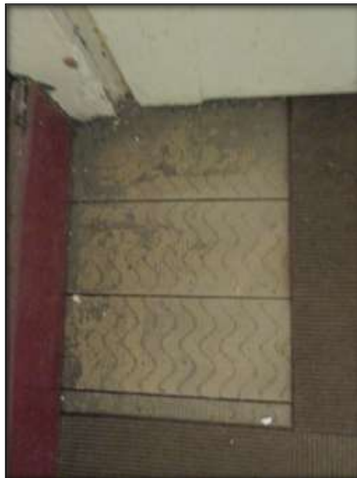
Fig.27: Modern carpets covering Wooden floor boards. The wood is most likely pine and not yellow wood as would be expected in an historical structure.
