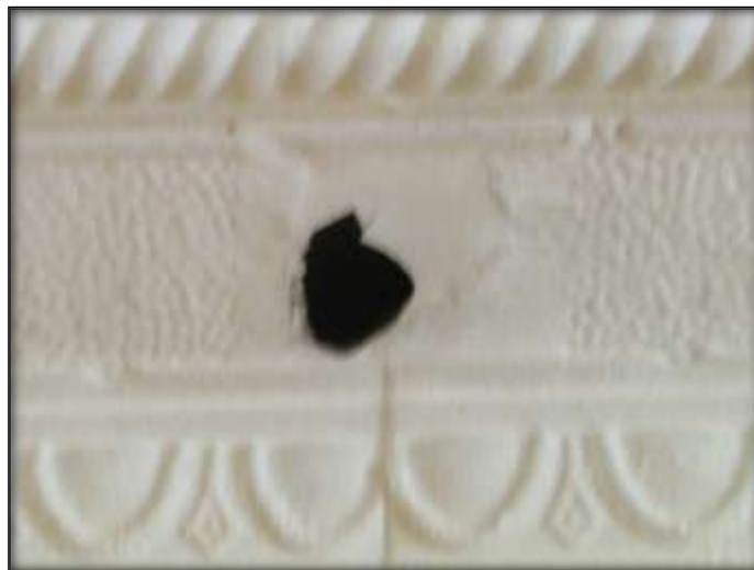
Fig.33: Closer view. Note the hole caused by rust.
