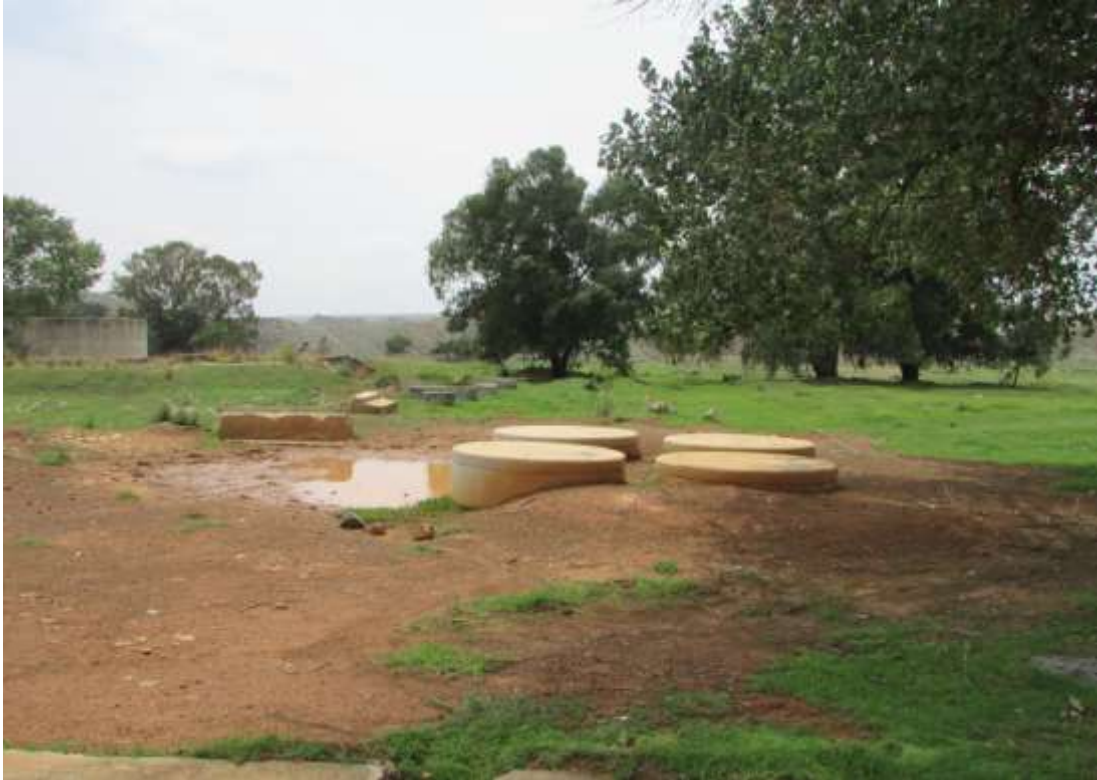
Figure 5: Another general view of the new pump station location. Note the existing sewer infrastructure.
