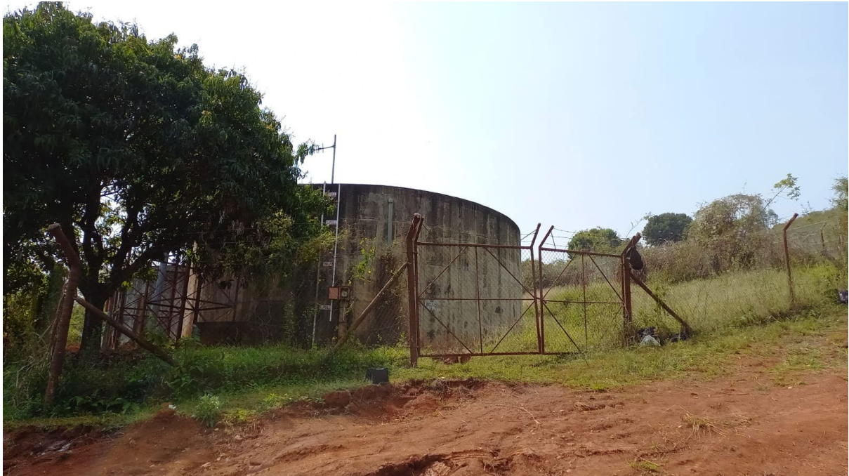
Figure 8: Large Water reservoir at entrance to the site accessible from the university (courtesy Reach Archaeology).
