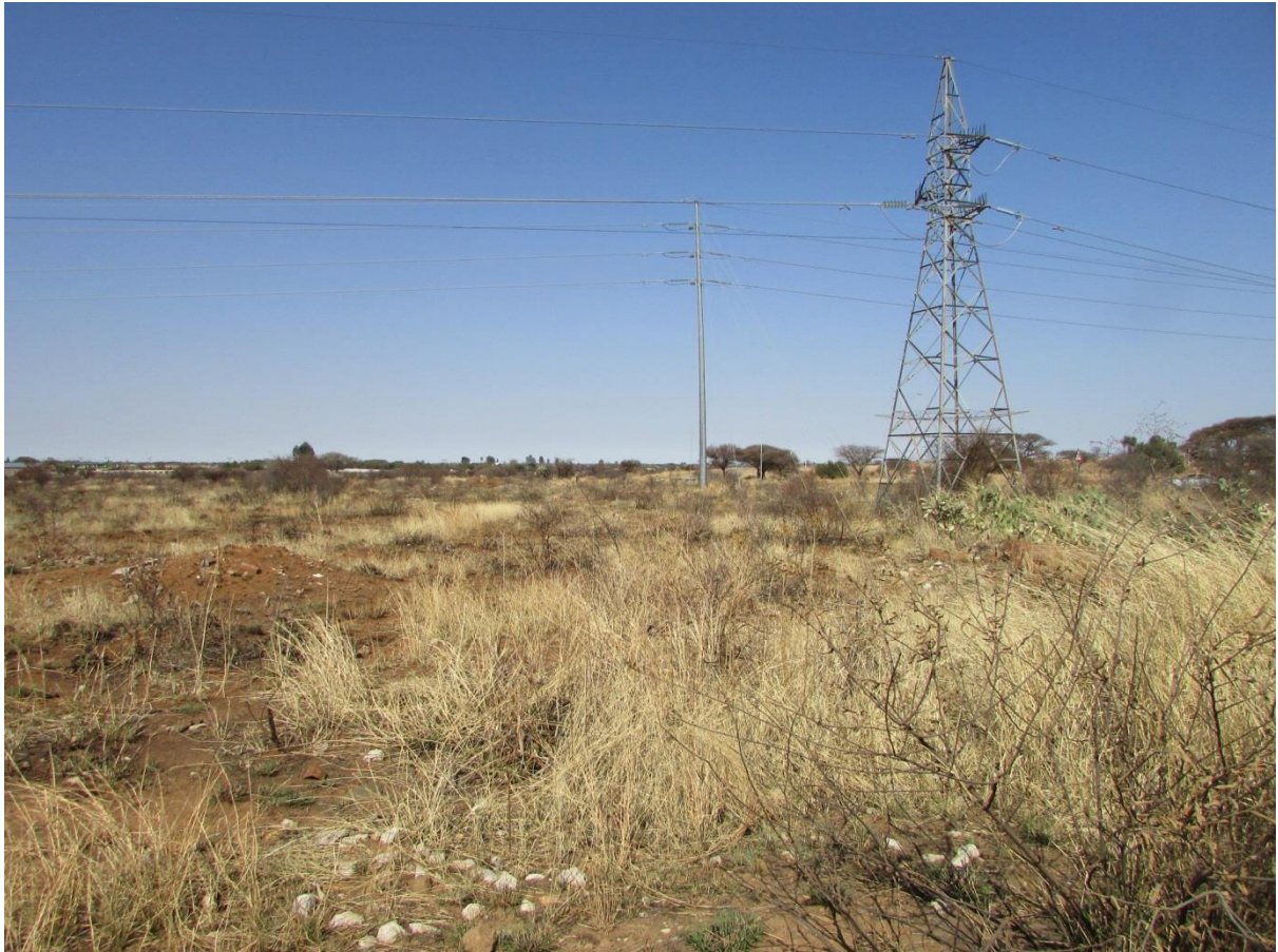
Figure 4: Another view of a section of the area. Note the ESKOM Powerlines, pylons & servitudes.
