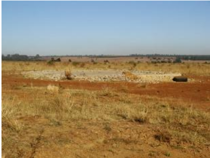
Figure 16: Site 2 cement and brick foundations.
