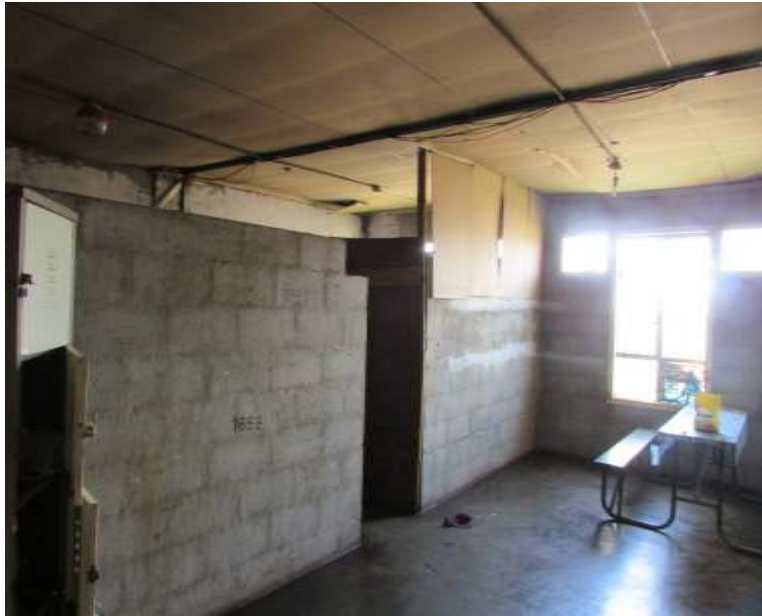
Figure 13: One of the bigger rooms with temporary partitions to form more rooms.
