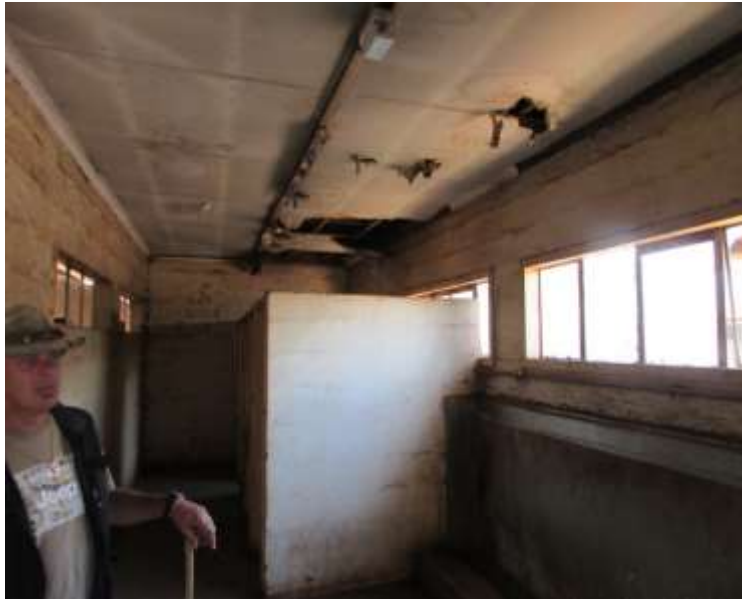
Figure 11: Inside one of the bathrooms.
