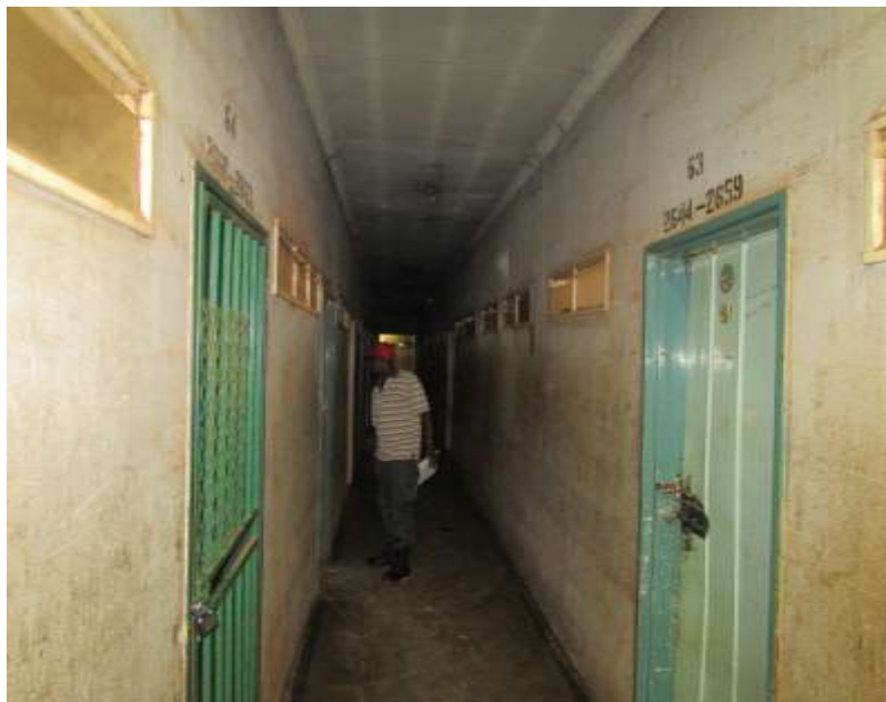
Figure 8: Inside the hostel showing the rooms and small corridors.
