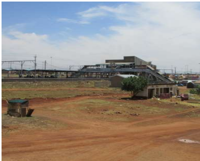
Figure 5: A view of Kwesine Railway Station taken from Kwa-Mazibuko Hostel.
