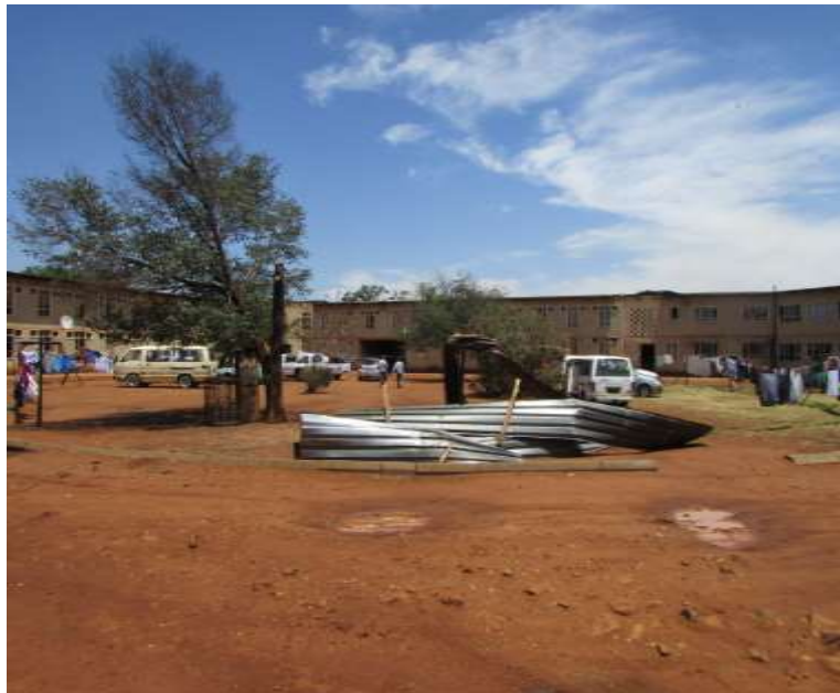
Figure 16: A view of the inner space of one of the other Blocks.
