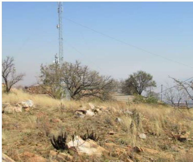
Figure 6: View of the approximate location of New Reservoir. The existing old reservoir is also visible.
