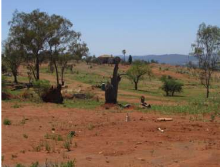
Figure 9: The feeder line route passes by some historical structures (visible in background) that form part of the West Fort Historical Village but has minimal if any impact.
