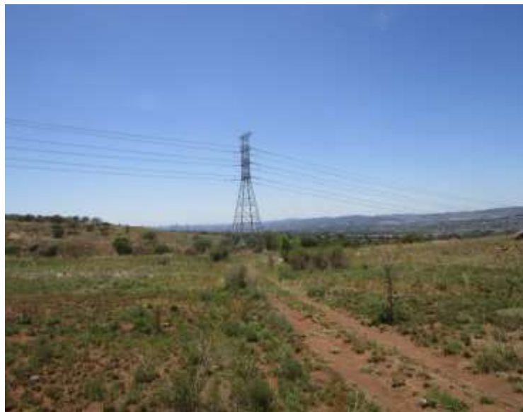
Figure 14: Other impacts on the area include Power lines.
