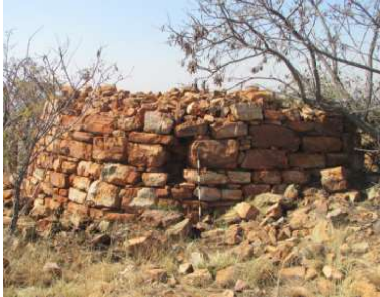
Figure 17: Another view of the structure.
