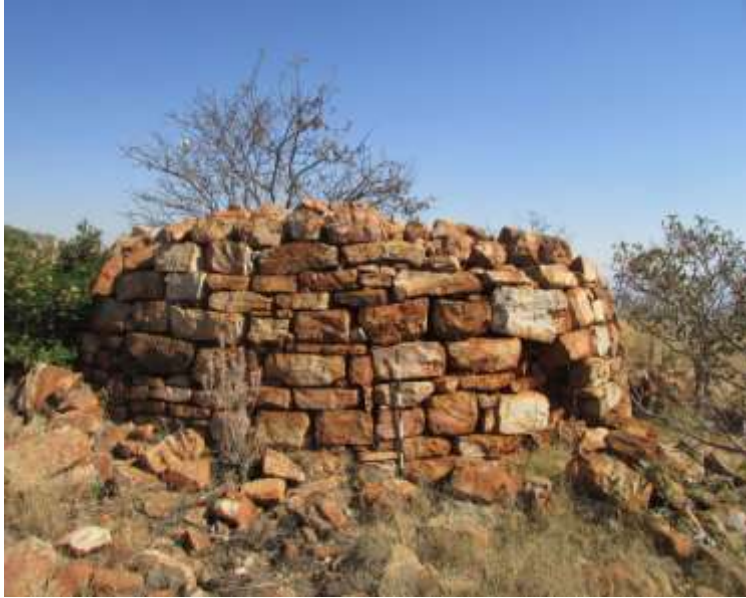
Figure 15: A view of the blockhouse.
