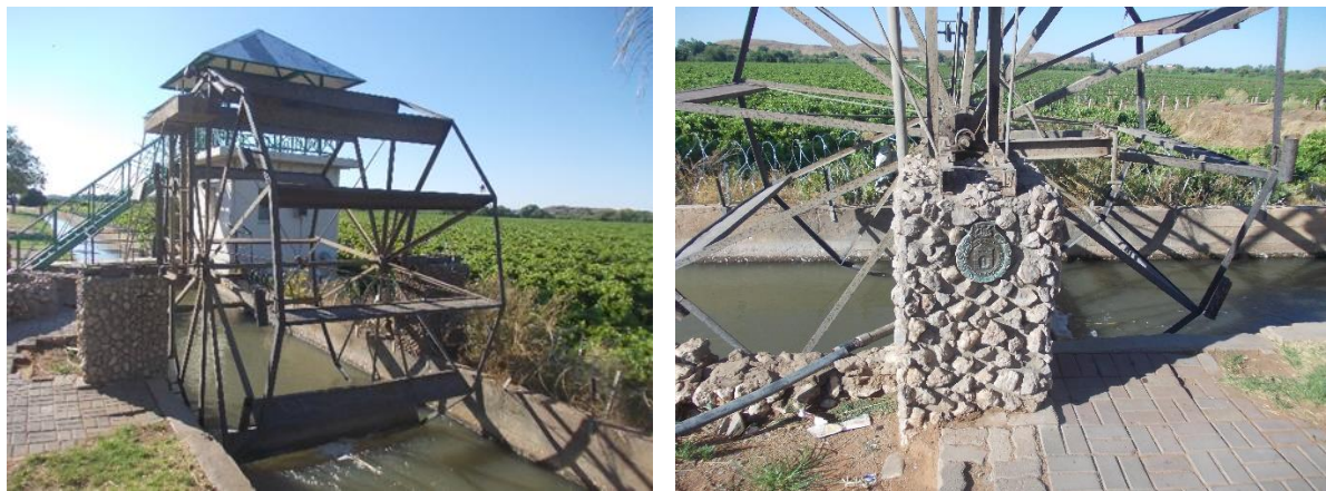
Figure 6 Historic water wheel, a declared provincial heritage site in Keimoes.
