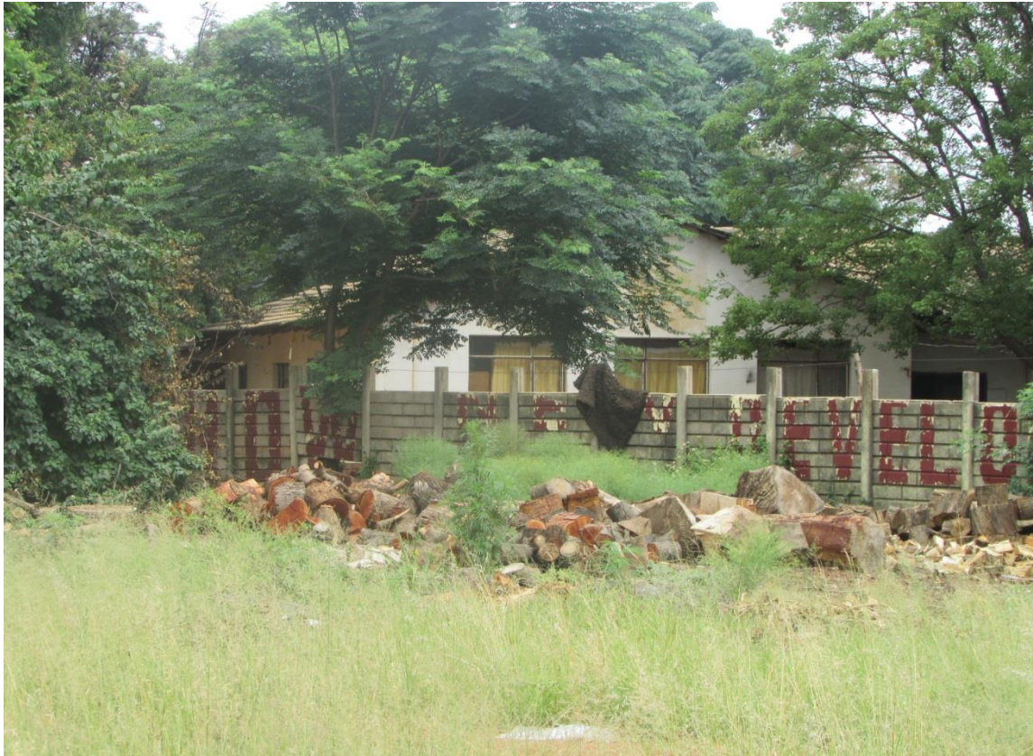
Figure 10: Partial front-view of the house on the property. The house and related structures most likely date to the 1970's.
