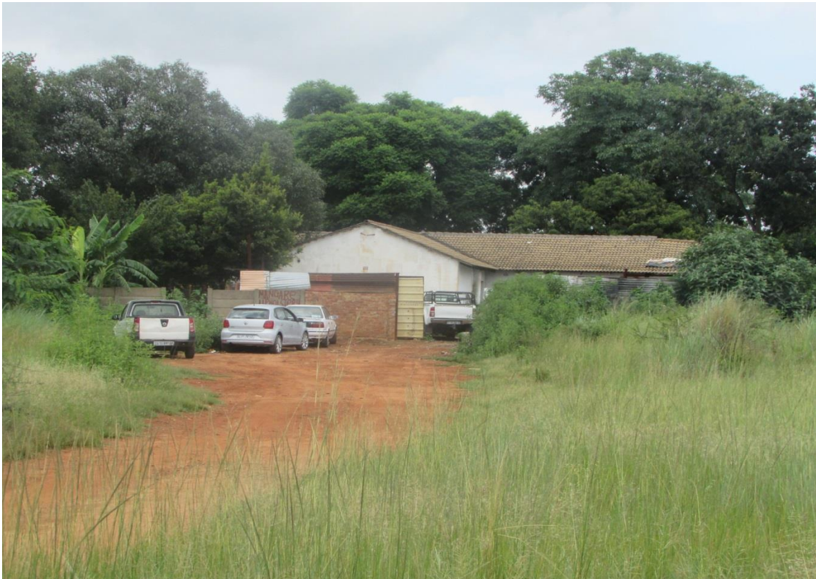
Figure 9: Back-view of the home and related structures on the property.
